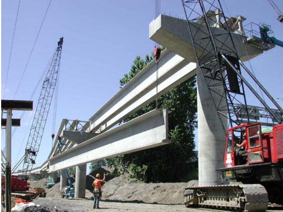
FIGURE 5 Interstate MAX light rail construction workers hoisting steel beam.
