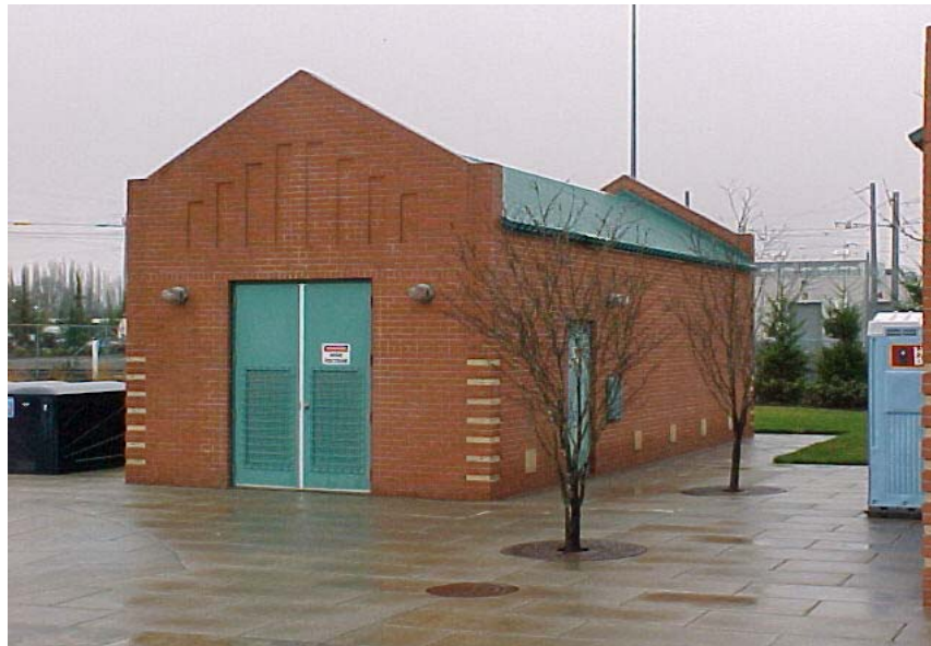
FIGURE 4 TriMet Westside LRT Expansion 170th Street Substation, 1998.
