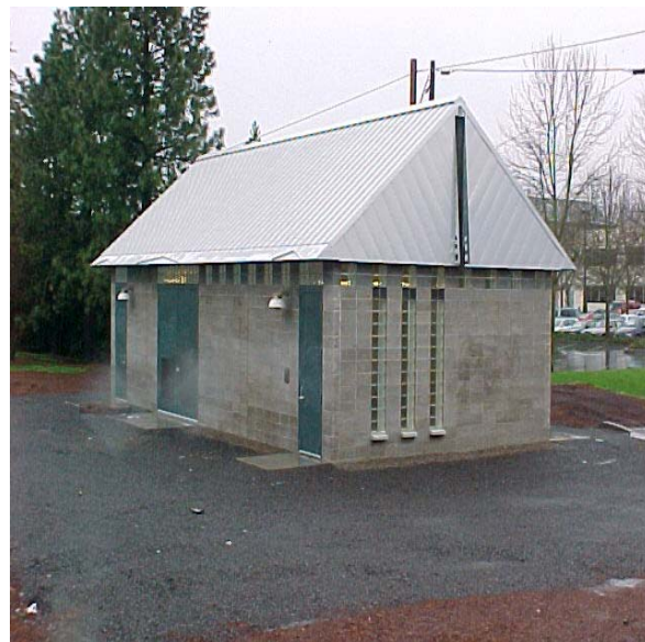
FIGURE 8 TriMet Interstate MAX LRT Failing Street Substation, 2003.
