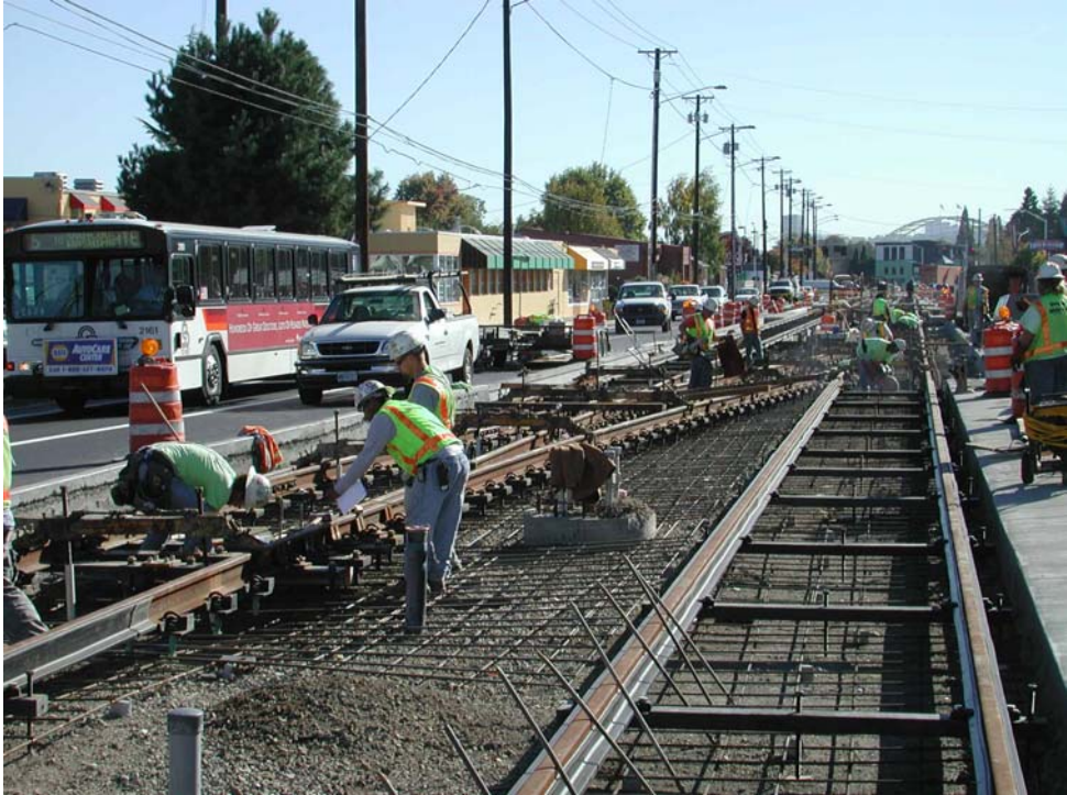
FIGURE 4 Interstate MAX light rail construction workers—track work.
