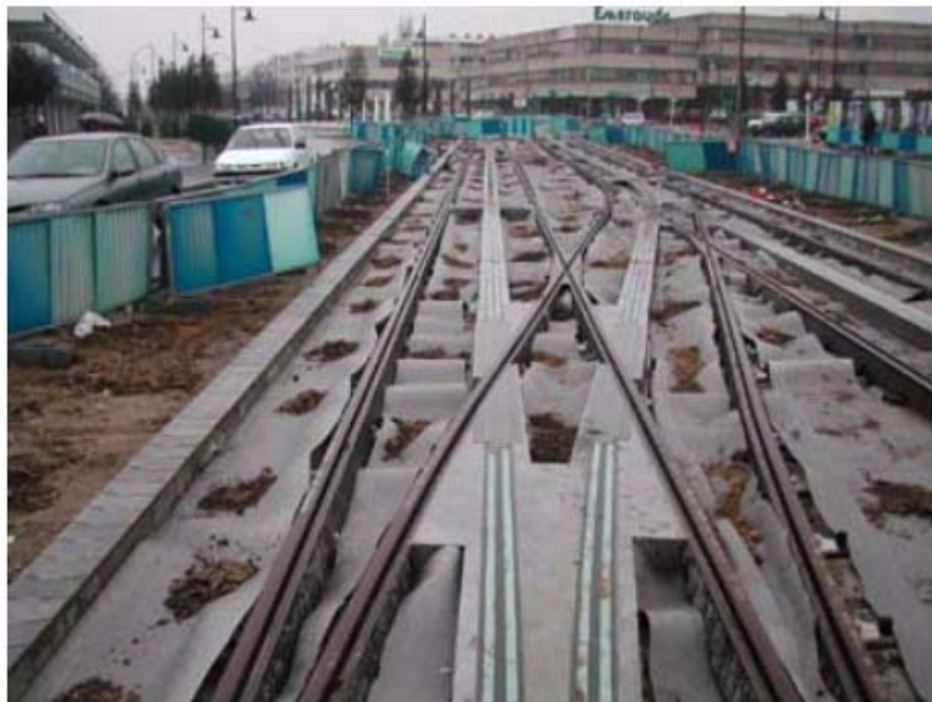
FIGURE 7 Crossing special trackwork.
