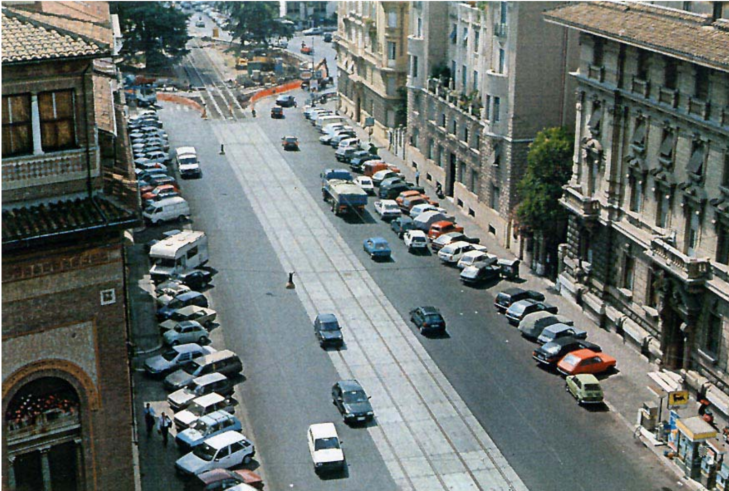
FIGURE 3 Aerial view of the construction site (last phase) on Viale Regina Margherita.
