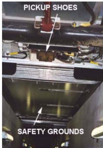
FIGURE 17 Shoe gear installation.
