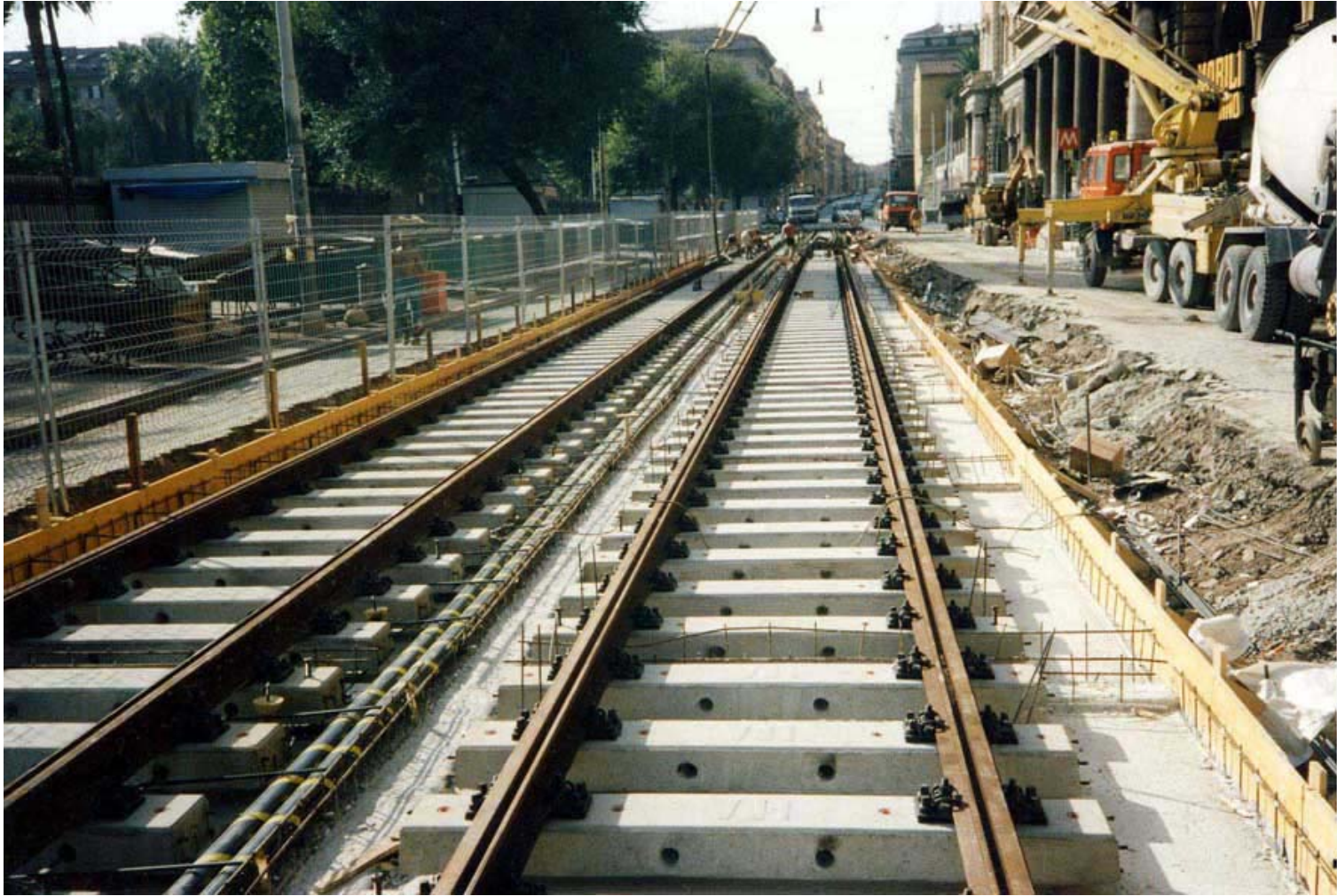
FIGURE 7 Piazza Vittorio Emanuele under construction.
