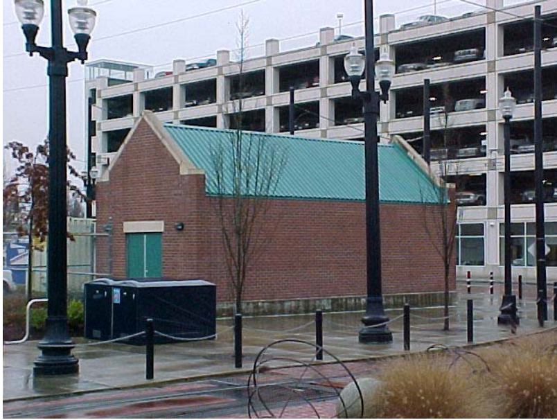
FIGURE 5 TriMet Hillsboro LRT Extension Government Center Substation, 1998.
