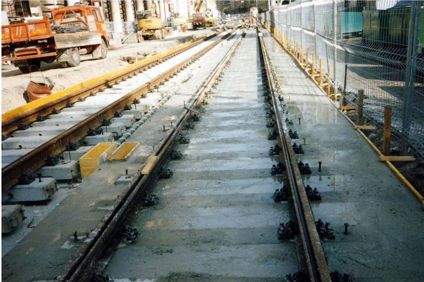
FIGURE 6 Piazza Vittorio Emanuele under construction. On the left, the first layer of concrete has been laid. On the right, the second layer of concrete has been laid, up to the top level of the concrete sleepers.
