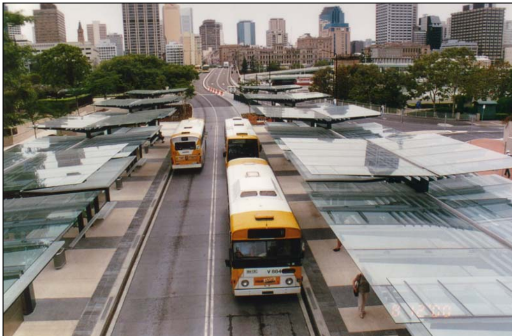
FIGURE 3 South–East busway at Southbank
