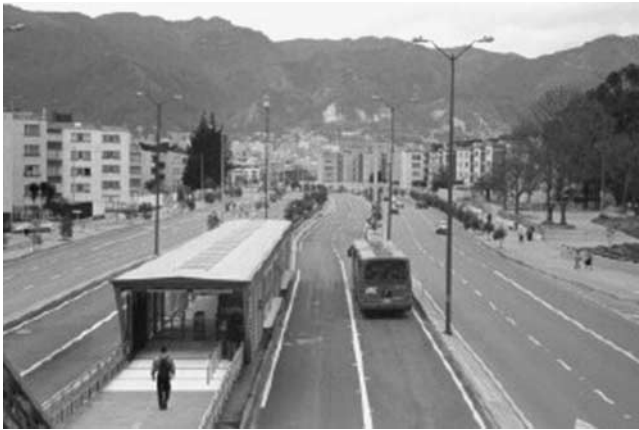
Photo 3-C. Median arterial busway, Bogotá.
