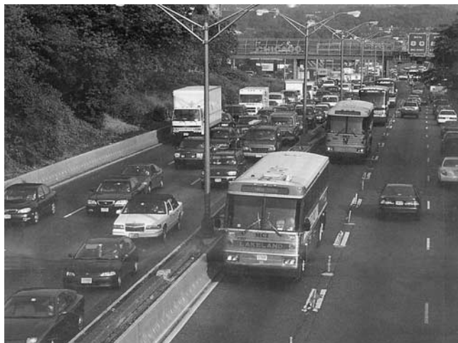
Photo 3-J. Contra flow lane on approach to Lincoln Tunnel, New Jersey.
