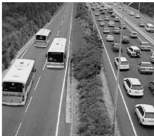
Photo 3-G. Busway adjacent to freeway, Brisbane, Australia.
