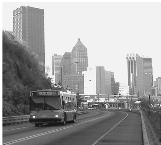
Photo 3-F. East (MLK) Busway, Pittsburgh.
