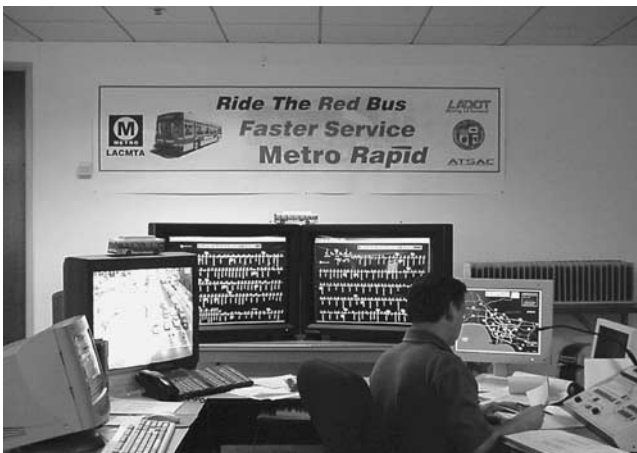
Photo 7-E. Central control room, Metro Rapid, Los Angeles.
