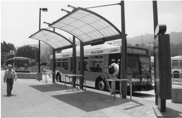
Photo 5-C. Los Angeles shelter.
