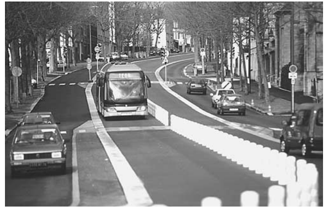
Photo 3-E. Median running way, Rouen, France, TEOR system.
