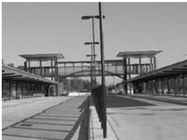
Photo 5-E. Grade-separated pedestrian crossing from Brisbane.
