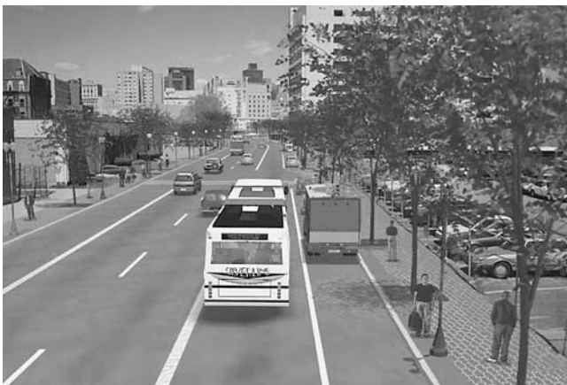
Photo 3-B. Interior bus lane, Silver Line, Boston.
