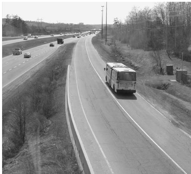
Photo 3-I. Queensway Busway shoulder lane, Ottawa.
