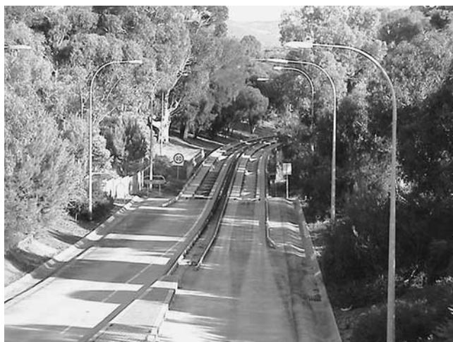
Photo 6-T. Running way with vertical guidance walls used by mechanically guided O-Bahn system (Adelaide, Australia).
