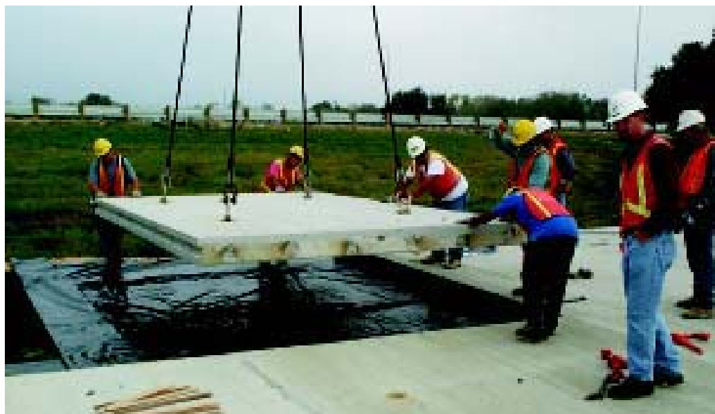
FIGURE 5 Precast deck panel construction.
