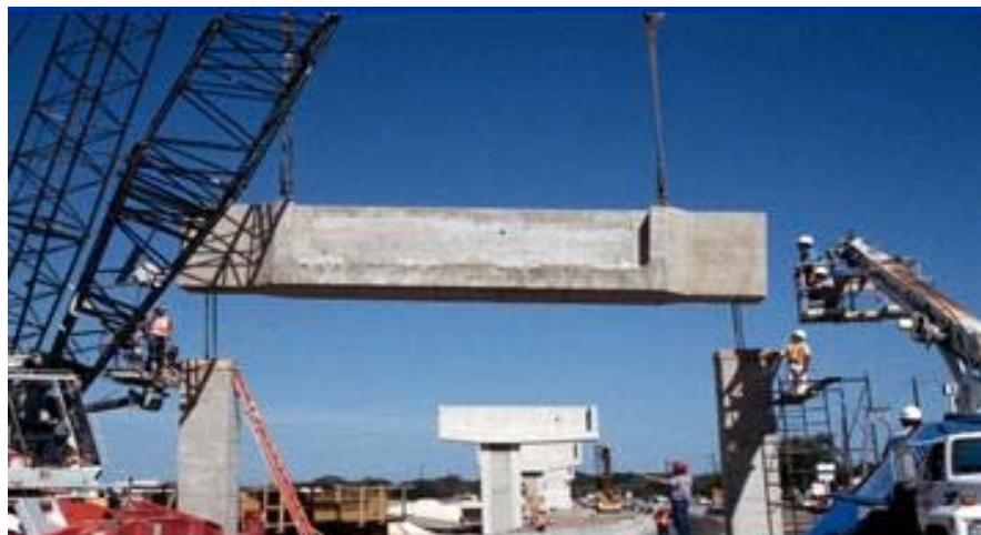
FIGURE 8 Texas DOT precast, prestressed bridge construction.
