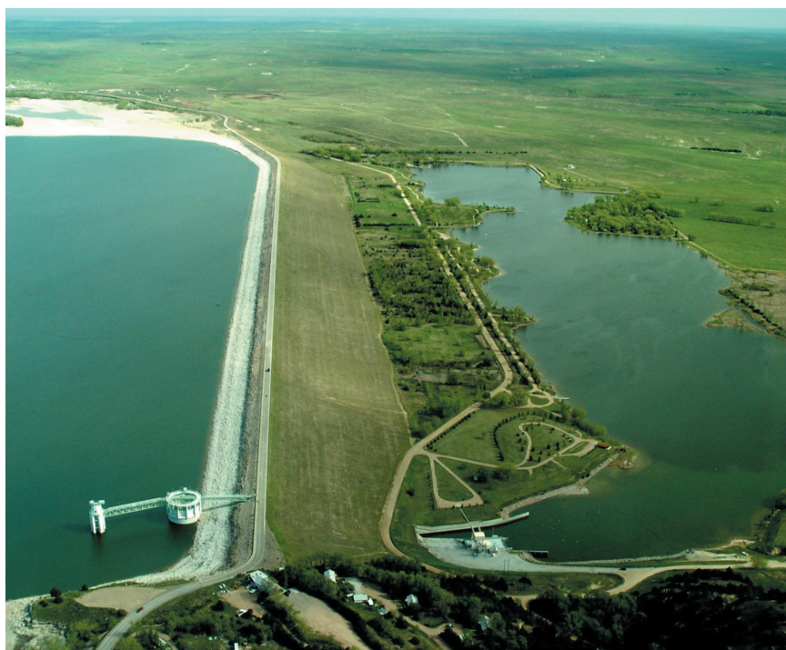
FIGURE 2-5 Kingsley Dam on North Platte River, completed in 1941, directly controls flows downstream through central Platte River. Source: Photograph by W.L. Graf, May 2003.
