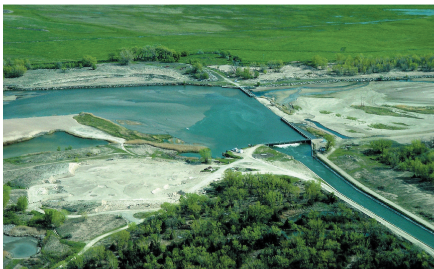
FIGURE 3-2 Keystone Diversion on the North Platte River, upstream from the central Platte River, represents an example of an effectively irreversible feature of the watershed that has enduring effects on flows. Source: Photograph by W.L. Graf, May 2003.
