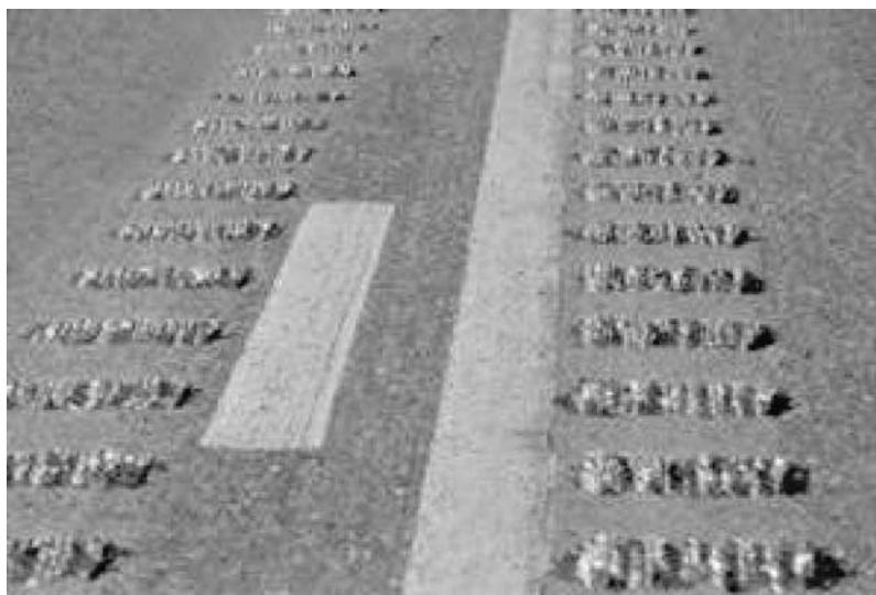
EXHIBIT V-7 Centerline Rumble Strips (Photo Provided by MnDOT)
