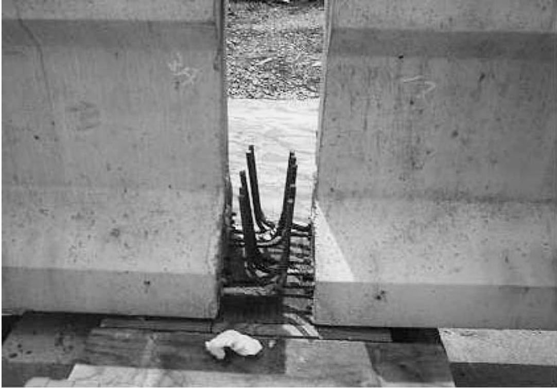
Figure 1. Bent-bar positive moment connection.
