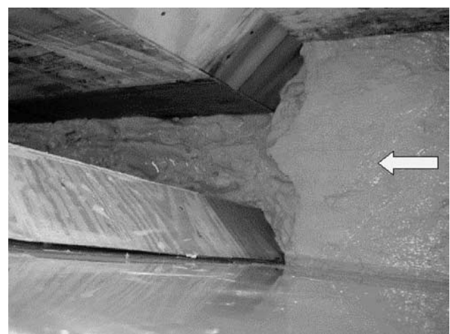
Figure A29 Scour Hole in Contraction Scour Test 10.
