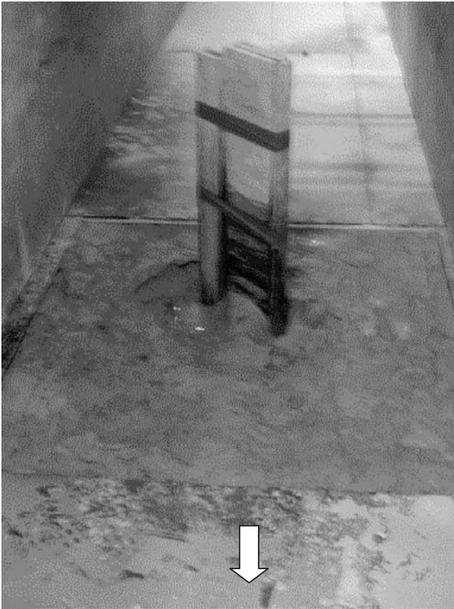
Figure A19 Scour Hole in Test At-8.
