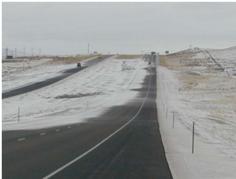
FIGURE 10 Blowing snow caused by absence of vegetation following reconstruction at I-80 mile 233 (January 15, 2003).
