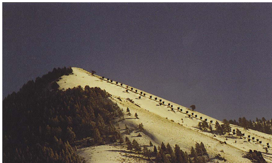
FIGURE 6 A view from the valley floor of the full 50-sail deployment of snow sails on the 151 avalanche.
