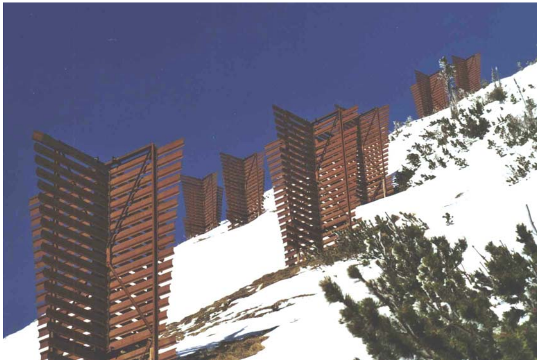
FIGURE 2 Modern European technology trails with omni (wind) directional kolktafeln in the Austrian Alps.
