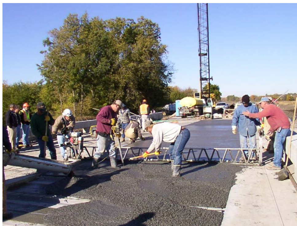
FIGURE 9 Casting the westbound lane with conductive concrete.
