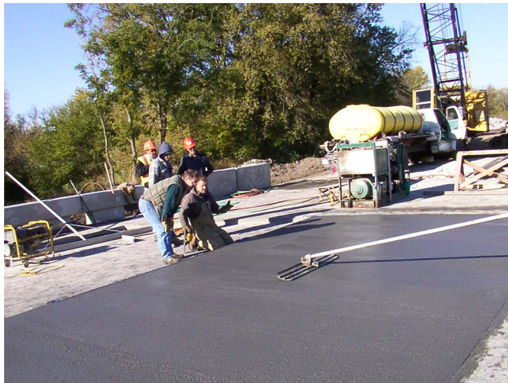
FIGURE 10 Finishing the conductive concrete inlay.
