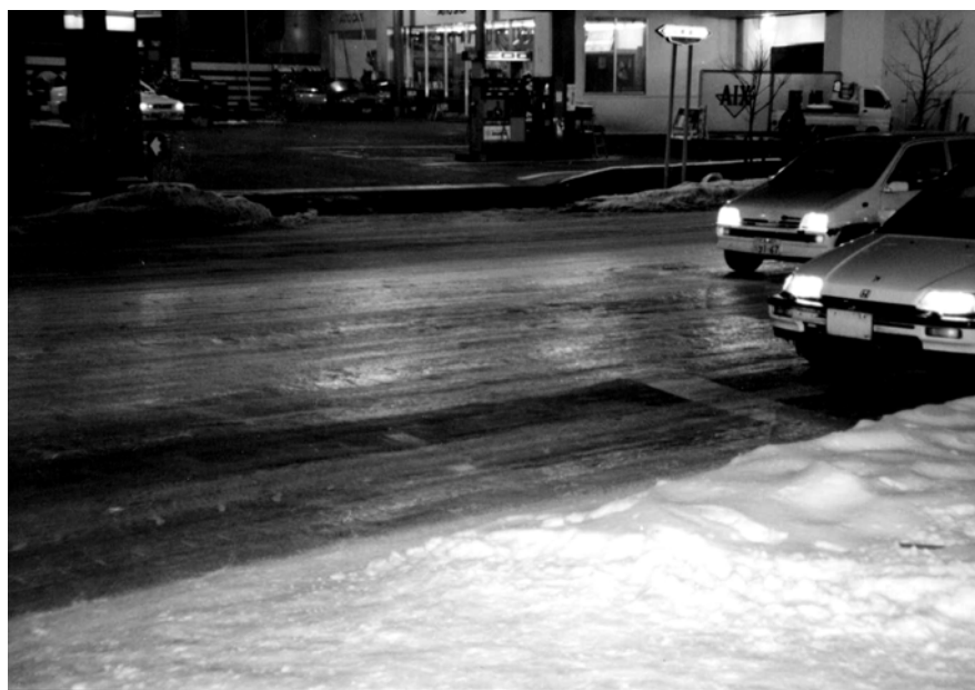
FIGURE 2 Extremely slippery crosswalk caused by studless tires.
