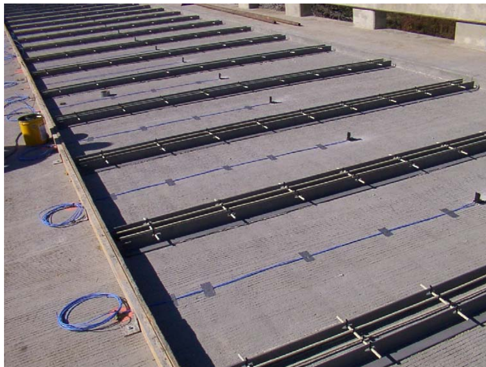
FIGURE 8 Electrode layout during construction.
