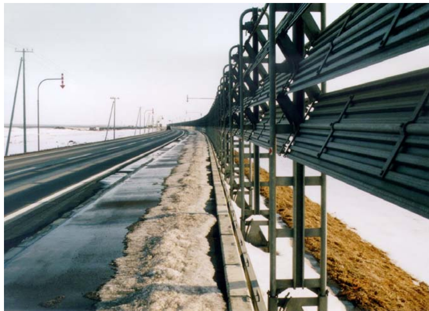
FIGURE 1 Blower snow fence equipped with angled fins that redirect wind downward to prevent snow from suspending the driver's line of sight.
