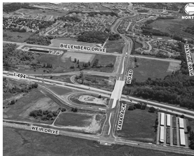
FIGURE 28 Tamarack Road/I-494 interchange after the project.
