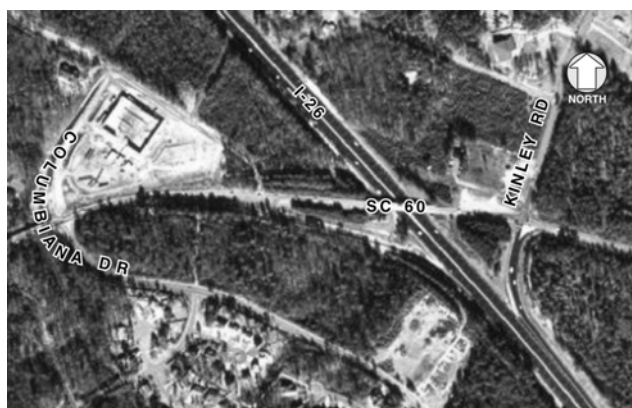
FIGURE 43 SC-60/I-26 interchange before the project (Courtesy: South Carolina DOT).
