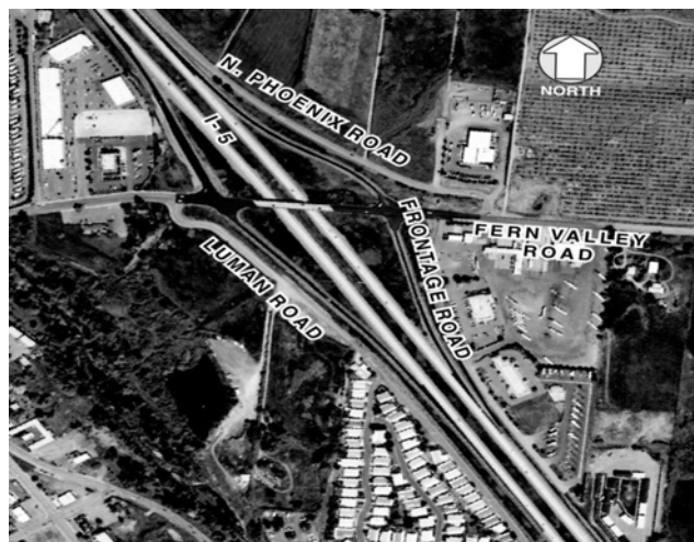
FIGURE 40 Fern Valley interchange before interchange project (Courtesy: Oregon DOT).
