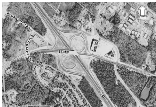
FIGURE 44 SC-60/I-26 interchange after the project (Courtesy: South Carolina DOT).
