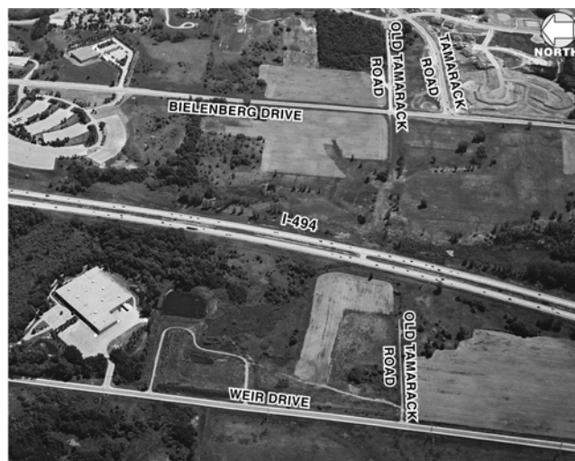
FIGURE 27 Tamarack Road/I-494 interchange before the project.
