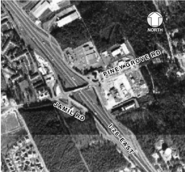
FIGURE 46 Piney Grove Road/I-26 interchange before the project (Courtesy: South Carolina DOT).
