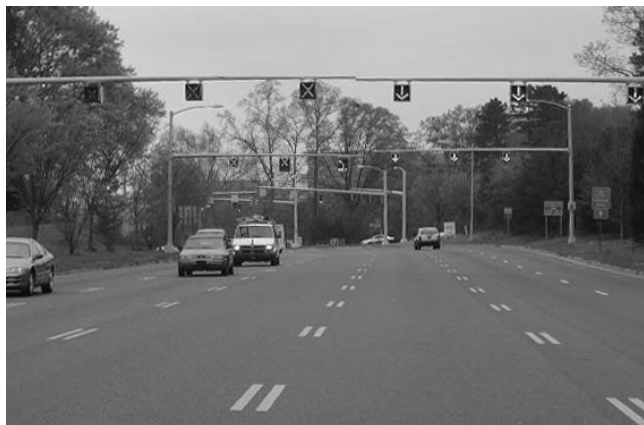
FIGURE 20 Overhead lane-use signals, Tyvola Road, Charlotte, N.C.
