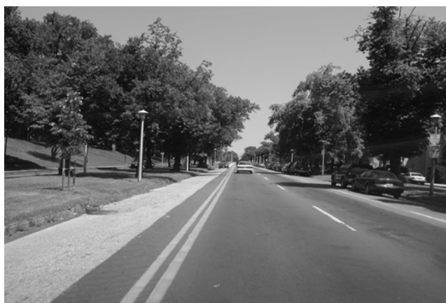
FIGURE 3 Charles Street southbound concurrent flow lane, Baltimore, Md.
