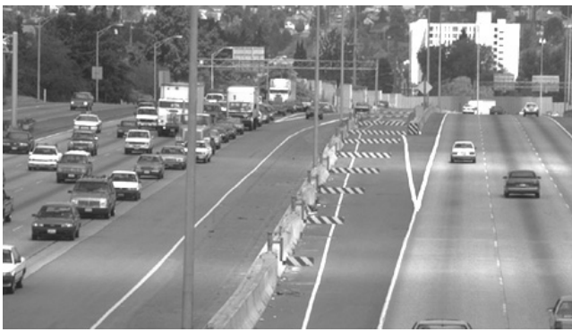
FIGURE 13 Typical gate design to prevent bidirectional entry, Seattle, Wash. [Source: "High Occupancy Vehicle (HOV) Interactive 1.0" 1996].
