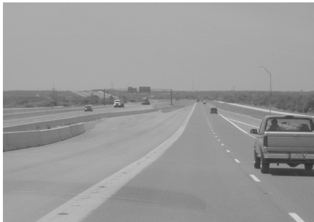
FIGURE 15 I-37 evacuation contraflow entry point, Corpus Christi, Tex. (Courtesy: Garry Ford, Texas Transportation Institute, San Antonio).
