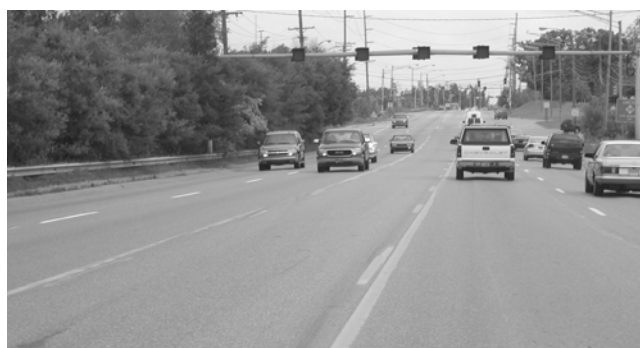
FIGURE 22 Deactivated lane-use signals and nonreversible pavement markings, Opdyke Road, Pontiac, Mich.
