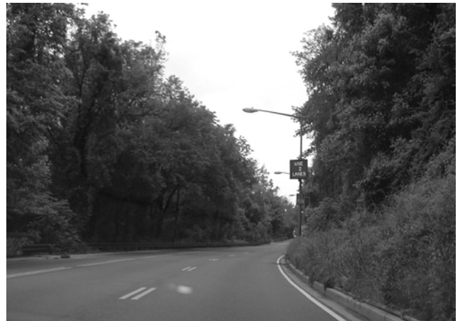
FIGURE 35 Canal Road—reversible lane variable message sign, Washington, D.C.
