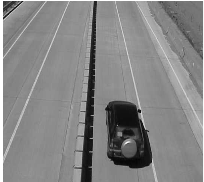
FIGURE 52 Overhead view of the use of shoulders as outer reversible lanes, Genesee County, Mich. (Courtesy: Armando Lopez, Michigan DOT).
