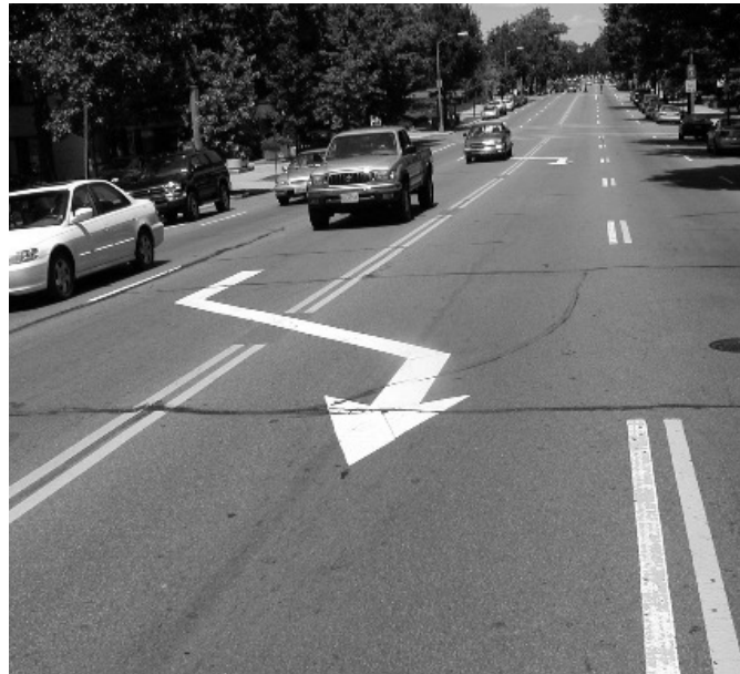
FIGURE 37 Connecticut Avenue—transition zone pavement markings, Washington, D.C.
