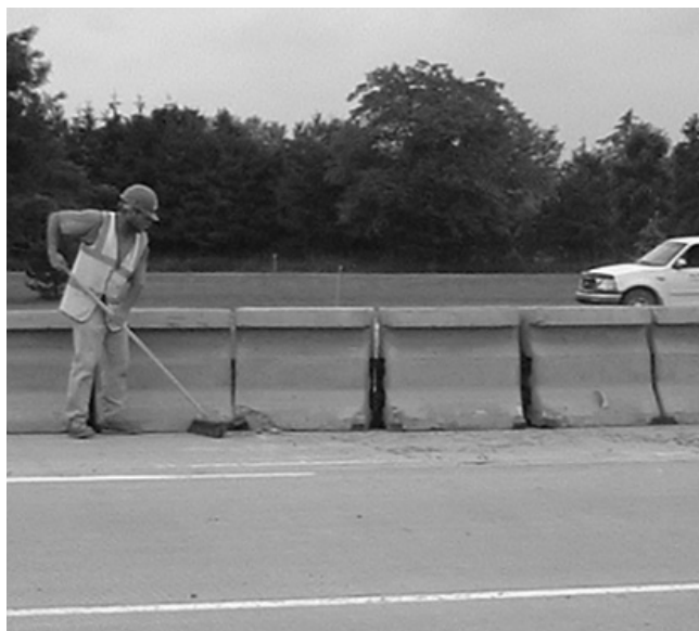
FIGURE 53 Cleaning of debris adjacent to movable barrier, Genesee County, Mich. (Courtesy: Armando Lopez, Michigan DOT).
