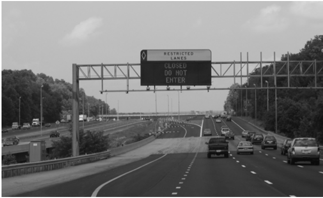
FIGURE 12 Gated reversible lane entry point, suburban Washington, D.C. and suburban Virginia.
