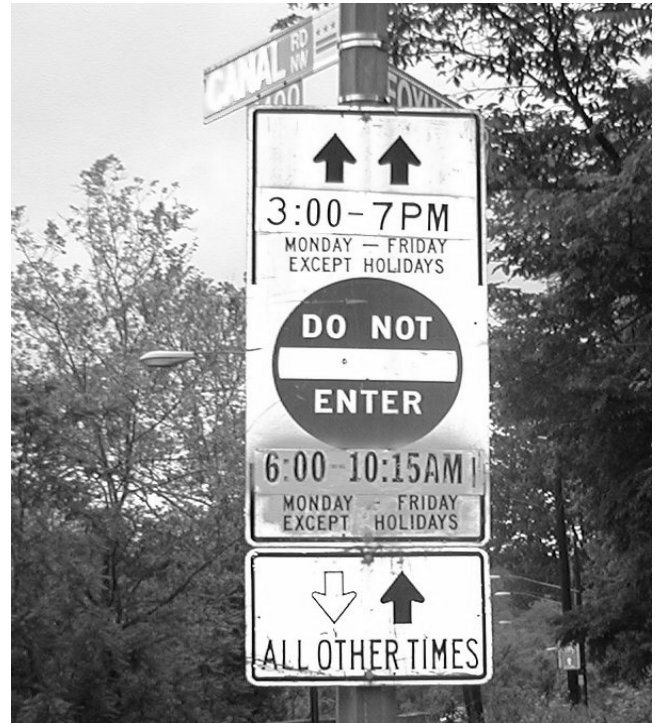
FIGURE 34 Canal Road—reversible lane control sign at Foxhall Road, Washington, D.C.
