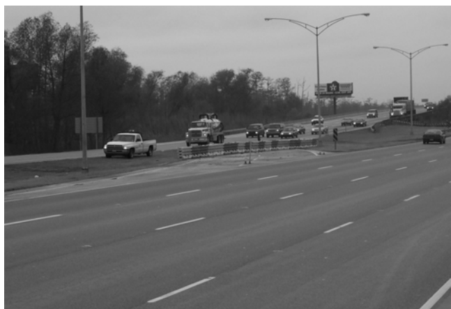
FIGURE 16 I-10 evacuation contraflow entry point, Kenner, La.
