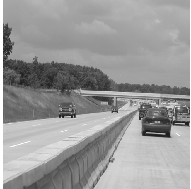
FIGURE 51 Cross-section view of the use of shoulders as outer reversible lanes, Genesee County, Mich. (Courtesy: Armando Lopez, Michigan DOT).
