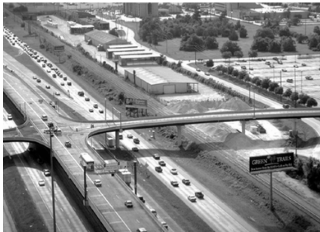
FIGURE 47 Elevated access ramp, Houston, Tex. [“High Occupancy Vehicle (HOV) Interactive 1.0” 1996].
