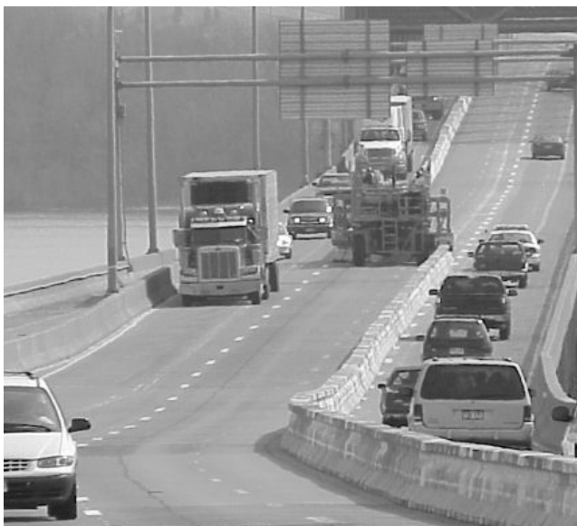
FIGURE 49 The "Zipper" moving the barrier into configuration for morning peak period, Peoria, Ill. ( Source : "Fact Sheet 5—Innovation During Bridge Rehabilitation Improves Mobility" 2003).
