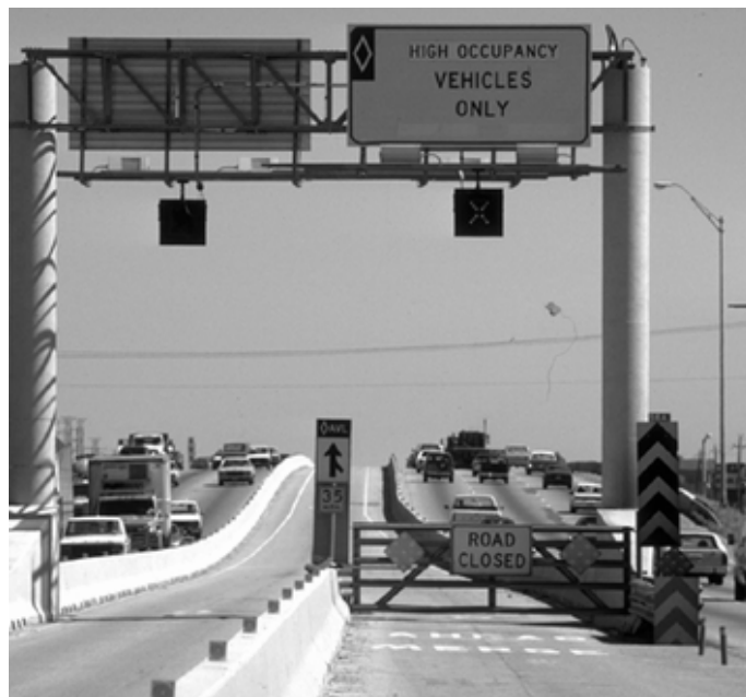
FIGURE 48 Intermediate access ramp, Houston, Tex. [“High Occupancy Vehicle (HOV) Interactive 1.0” 1996].
