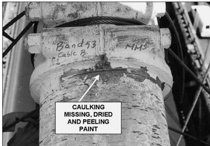
Figure 2.3.1.2.2-1 Damaged caulking and paint at cable band.
