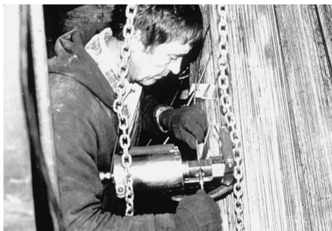
Figure D.1.3-2. Applying ferrules with a hydraulic ram.
