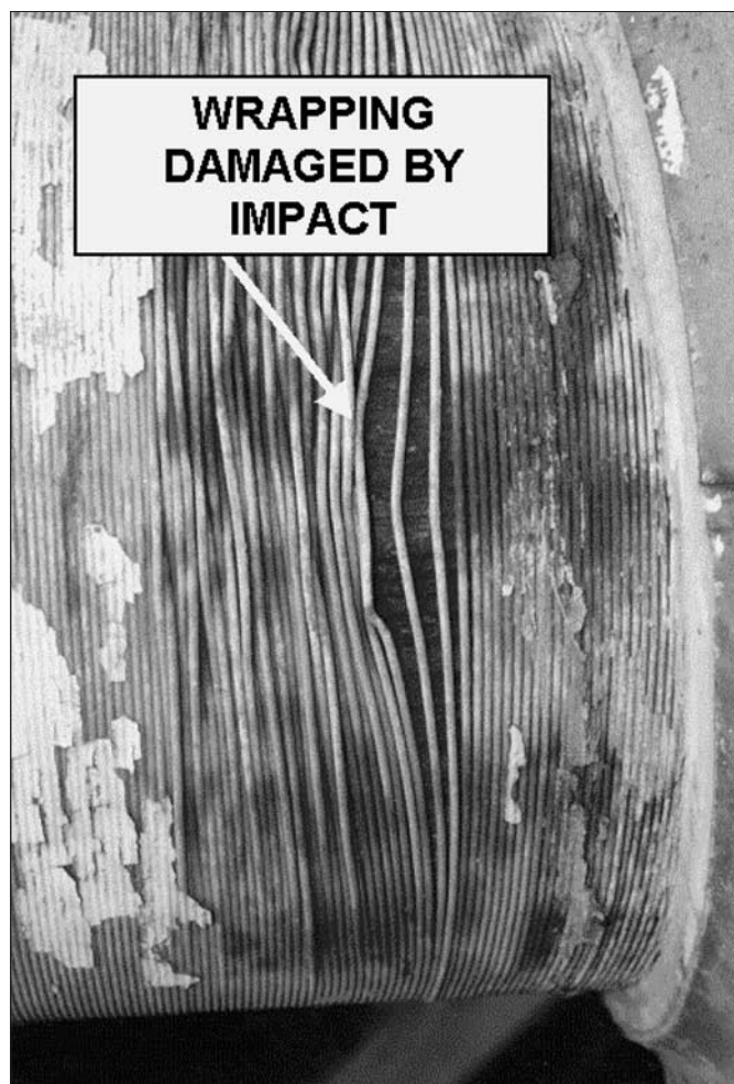
Figure 2.3.1.2.2-5. Damage to wrapping caused by vehicular impact.
