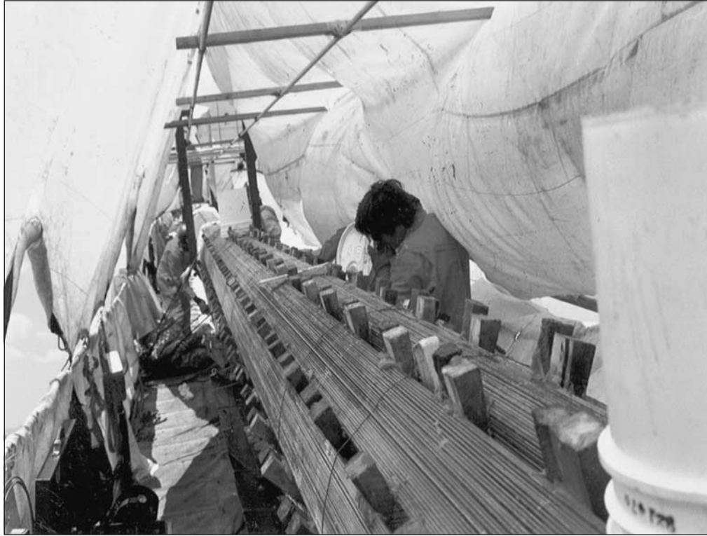
Figure 2.4.8.1-1. Inspection during cable rehabilitation.
