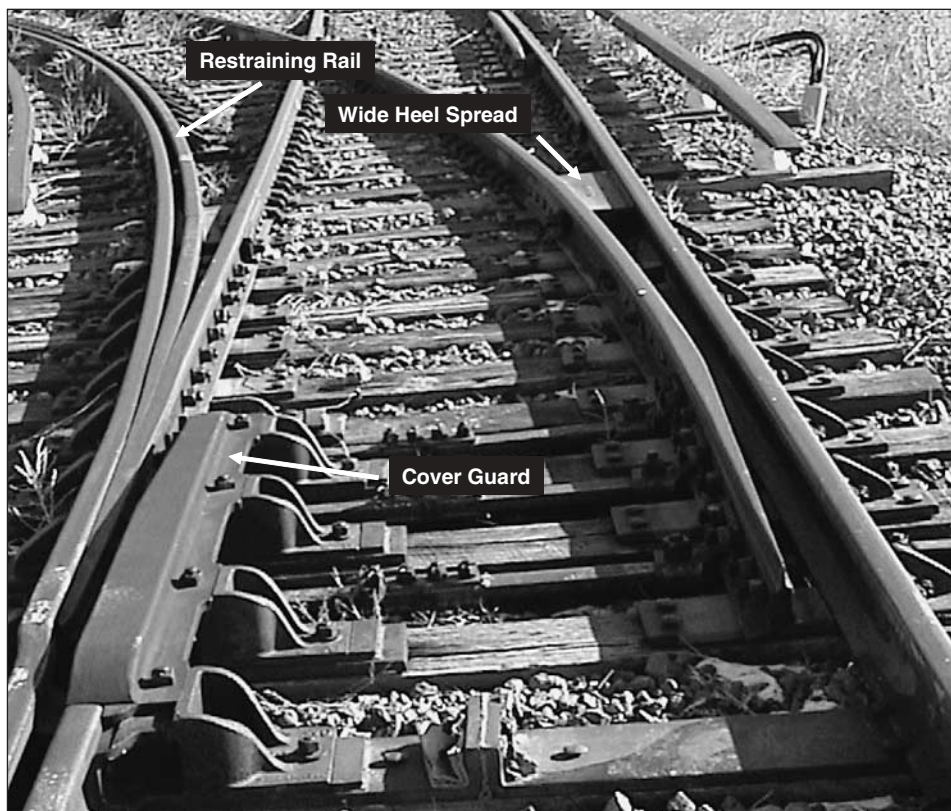
Figure 4. Typical guarded switch with cover guard.
