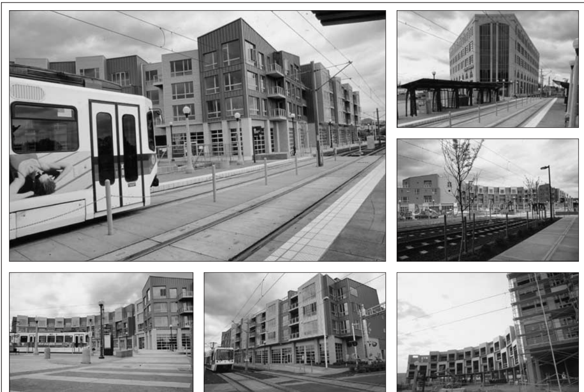
Photo 17.2. The Round. The Round stands out as a pioneering suburban downtown mixed-use infill project.
