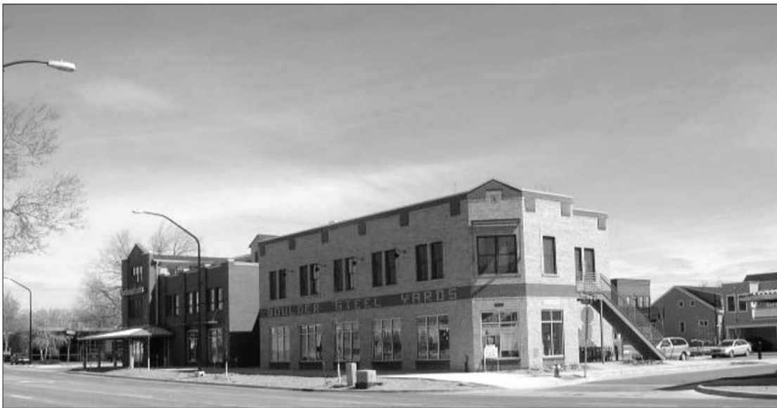
Photo 16.7. Mixed-Use Redevelopment Along Transit Corridors. Located along 30th Street, a corridor of industrial and automobile-oriented retail uses, the Steel Yards is precisely the type of redevelopment the city of Boulder hopes will reshape the area over coming decades. The $27-million project is being developed in phases and will total 22 buildings, including 90 residential units and 137,000 square feet of office and retail space, when completed. After rejecting earlier proposals for big-box retail on the site, the city rezoned the property in 1997 to allow for mixed-use development. The city views the Steel Yards as an example of the area’s redevelopment potential and is studying similar opportunities along 30th Street. The photo shows a view of the Steel Yards, with mixed-use commercial buildings fronting onto 30th Street and parking and additional residential uses tucked behind.
