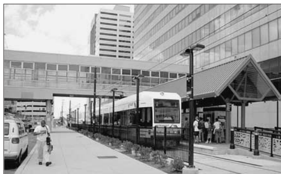
Photo 11.8. Light Rail at the Newport Centre Mall. The light-rail line lies under a pedestrian skywalk that connects Newport office tower (on the right) to the modern three-story indoor mall on the left (west) of the station.
