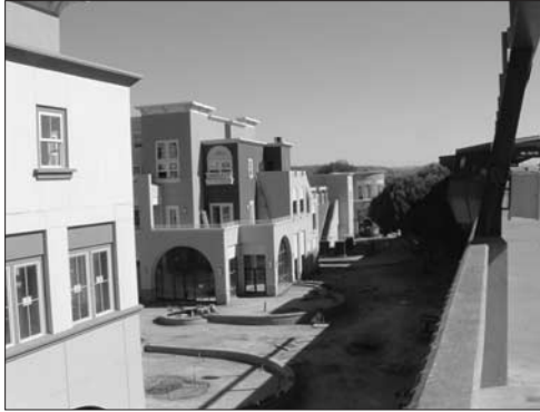
View from the BART Platform
