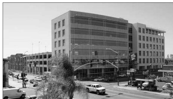
Photo 19.5. City Heights Office and Townhomes, San Diego, California.
