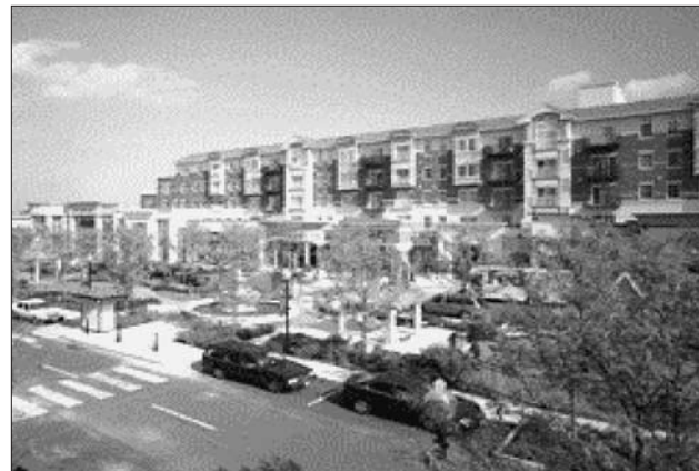
Photo 6.2. Contrasting Approaches to Mixed-Use TOD Parking in Arlington County, Virginia. Pentagon Row, in the top photo, relied heavily on below-surface podium parking, inflating construction costs. Market Common, in the bottom photo, put parking on the street, complemented by nice landscaping, to save costs, even though its building profile is similar.
