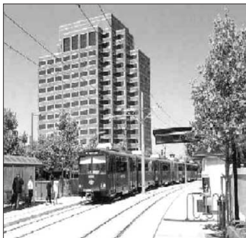
Hazard Center TOD, Mission Valley Trolley Line
