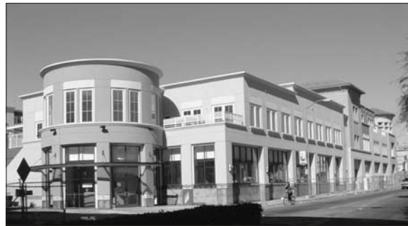
Corner Retail Near BART Station Entrance
