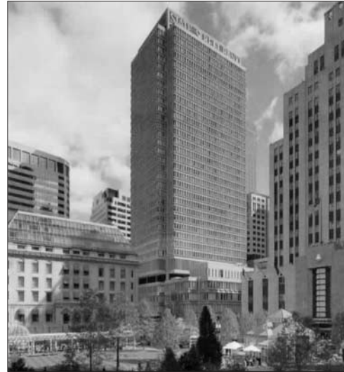
Photo 10.3. Renovated State Street Bank Building. The refurbished building's comeback typified the spectacular performance of the Boston office market and real-estate market in general in the 1990s.
