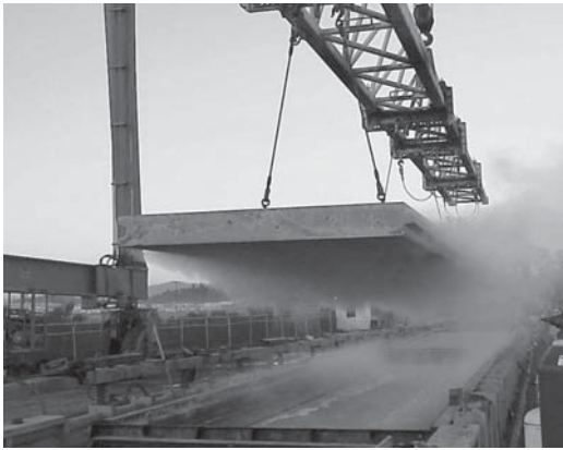
Prefabricated portland cement concrete panels installed on I-10.
