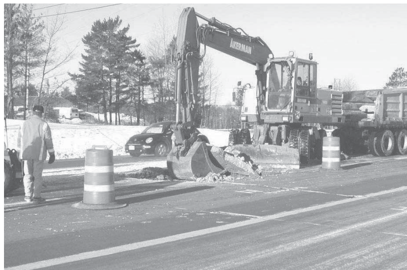
Removing a concrete pavement section in Wisconsin.
