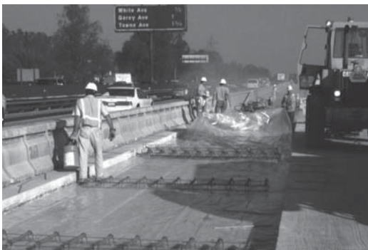
Construction crews work at night to minimize delays for motorists.
