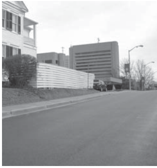
Pothole-free street in Rockville, Maryland, overlaid with smooth seal.
