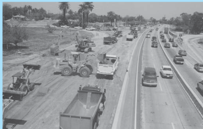
Planners relied on CA4PRS evaluations for I-710 Long Beach rehabilitation project.
