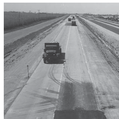
Working on the 1 million applications in each Road Test lane.
