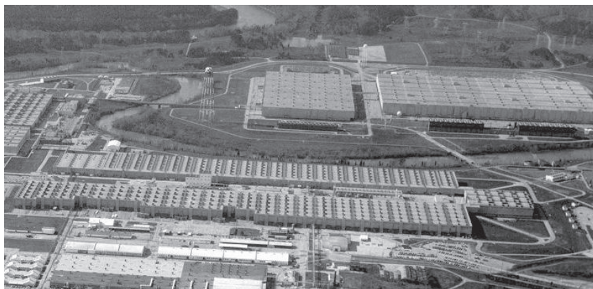
FIGURE 2.1 Much of the gaseous diffusion equipment in the K-25 plant at Oak Ridge dating back to the Manhattan Project-era remains classified. Worker access restrictions make the massive job of decommissioning K-25, which includes about 14 million square feet of floor space, more difficult. Photo courtesy of Oak Ridge Operations Office.
