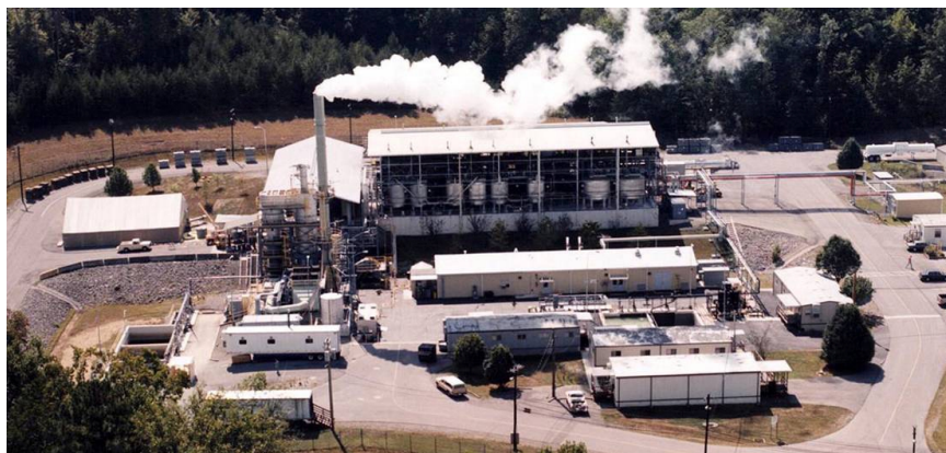
FIGURE 3.1 The TSCA incinerator at Oak Ridge provides EM's only capability for burning mixed low-level radioactive wastes. Photo courtesy of Oak Ridge Operations Office.
