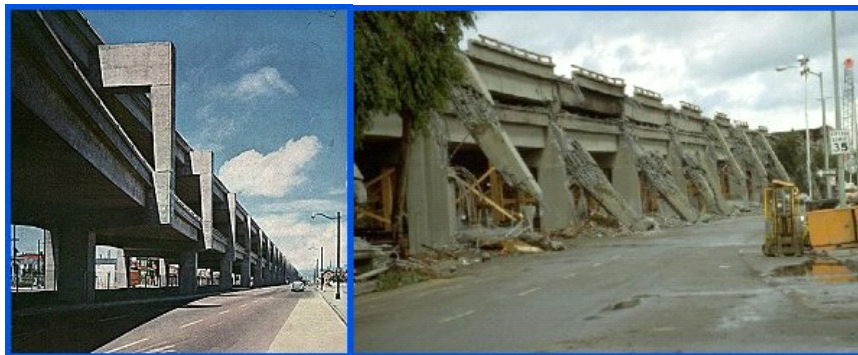
FIGURE 2.1 The Cypress Street Viaduct (left) before the earthquake of 1989 destroyed much of the structure (right), requiring its demolition. SOURCE: EBMUD Seismic Improvement Program. Available [on-line] at: http://home.pacbell.net/hywaymn/Cypress_Viaduct_Freeway.html
