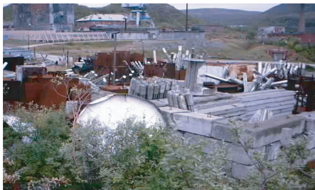
FIGURE 17 View of an open accumulation area for solid radioactive waste at the Andreeva Bay base.
