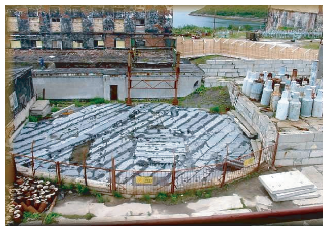
FIGURE 16 View of the concrete ceiling of Building 3A of the spent nuclear fuel dry storage facility at the Andreeva Bay base.
