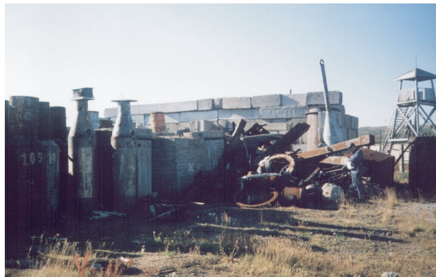
FIGURE 18 Storage area for solid radioactive waste in Gremikha.
