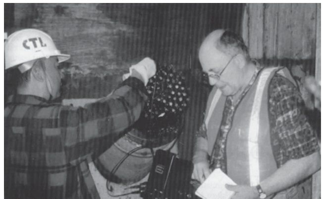
FIGURE 60 Ultrasonic testing of cable anchorage (Ciolko and Yen 1999).
