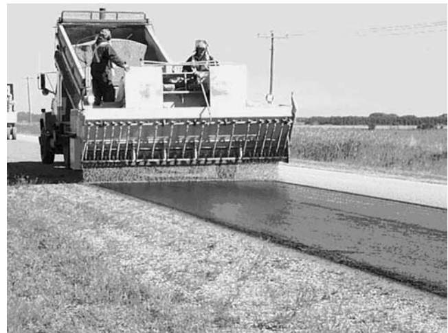
FIGURE 49 Aggregate applied with self-propelled spreader.
