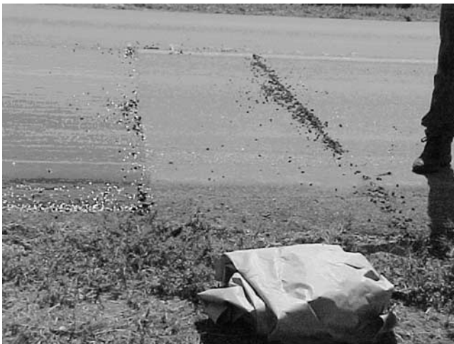
FIGURE 48 Paper used to ensure seamless transverse joint.
