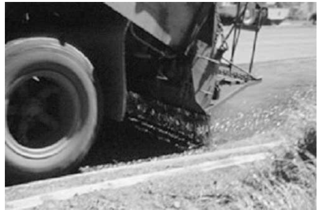
FIGURE 34 Dump truck bed aggregate spreader.
