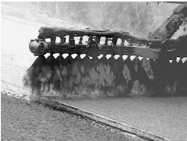
FIGURE 46 Spray bar applying bituminous binder.
