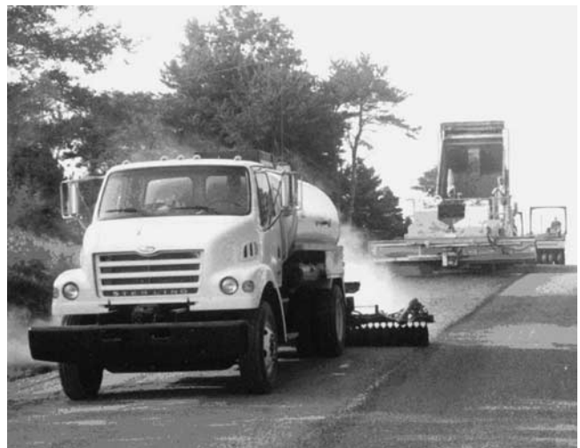
FIGURE 47 Aggregate spreader within proximity of distributor.
