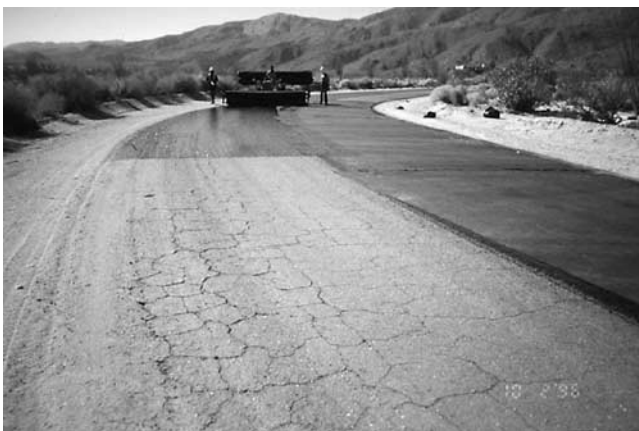
FIGURE D1 Geotextile installation on cracked road surface.
