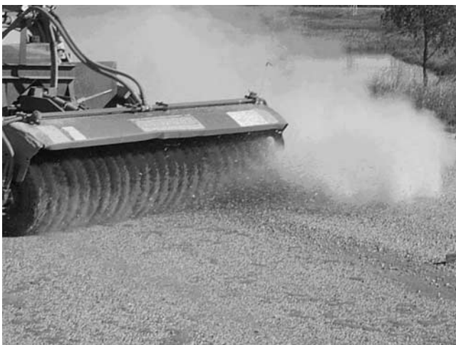
FIGURE 43 Rotary broom sweeper preparing surface for sealing.
