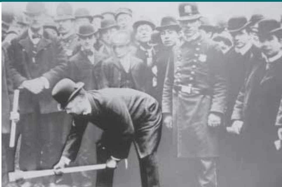
Parsons swings the pickaxe to start construction on the subway at Bleecker and Greene Streets.
