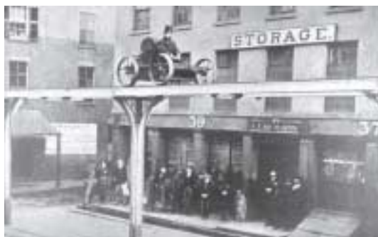
Charles T. Harvey, who designed and promoted the West Side and Yonkers Patent Railway, runs a test on Greenwich Street, 1867. The system experienced frequent breakdowns and closed in 1870.
