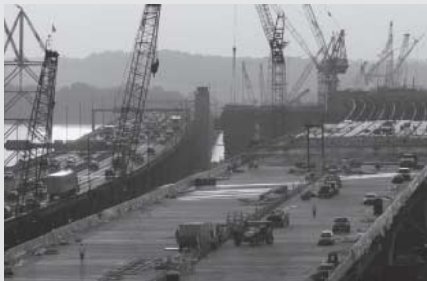
The draw spans, or bascules, of the new Woodrow Wilson Bridge, near Washington, D.C., feature eight opening leaves composed of more than 14 million pounds of steel.
