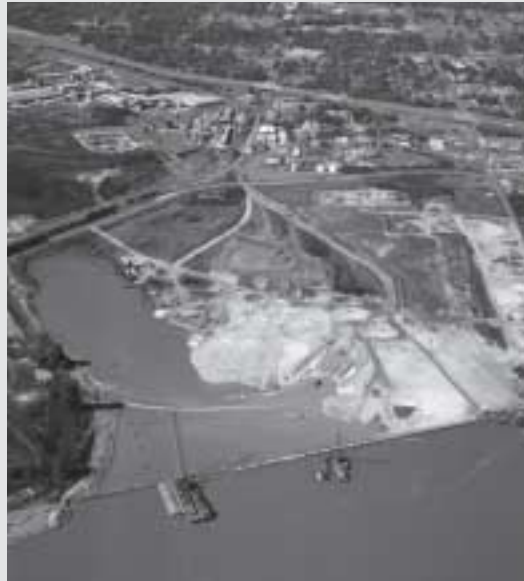
Site for the construction of Choctaw Point Terminal, Mobile, Alabama.
