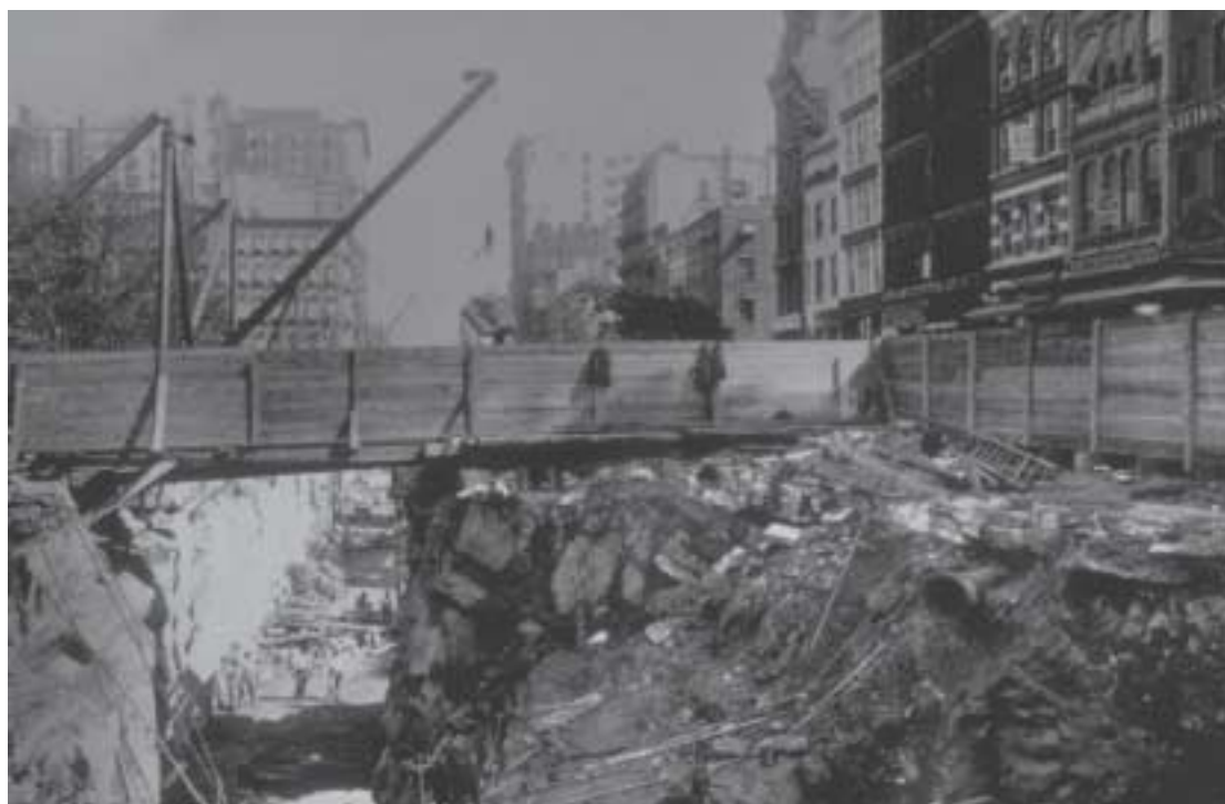
Cut-and-cover construction of the subway earned the name "Parsons's ditch."
