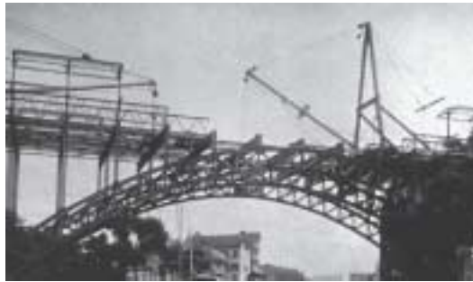
At Broadway and 125th Street, the first subway line crossed a trussed arch bridge, still standing today.
