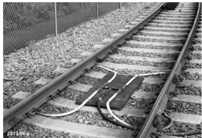
Figure 17. TOR applicator bars dispensing friction control material.
