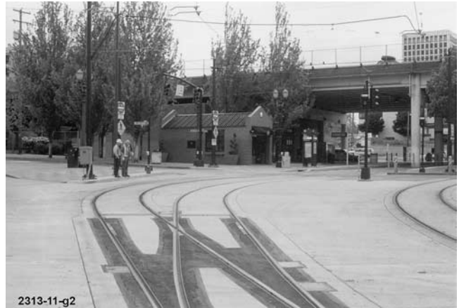
Figure 8. Curve protected by drilled-hole applicator system.
