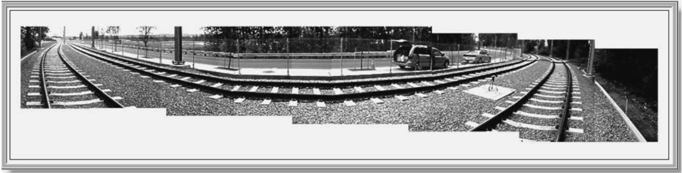
Figure 2—Photo of test site near north end of transit line close to the Portland Expo Center. Note: Northbound rail is near photographer. Southbound rail is nearest autos in the photo.
