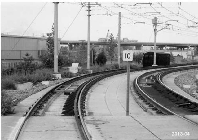
Figure 16. Two mainline curve lubricator applicators supplied from one centrally located reservoir and pump system.
