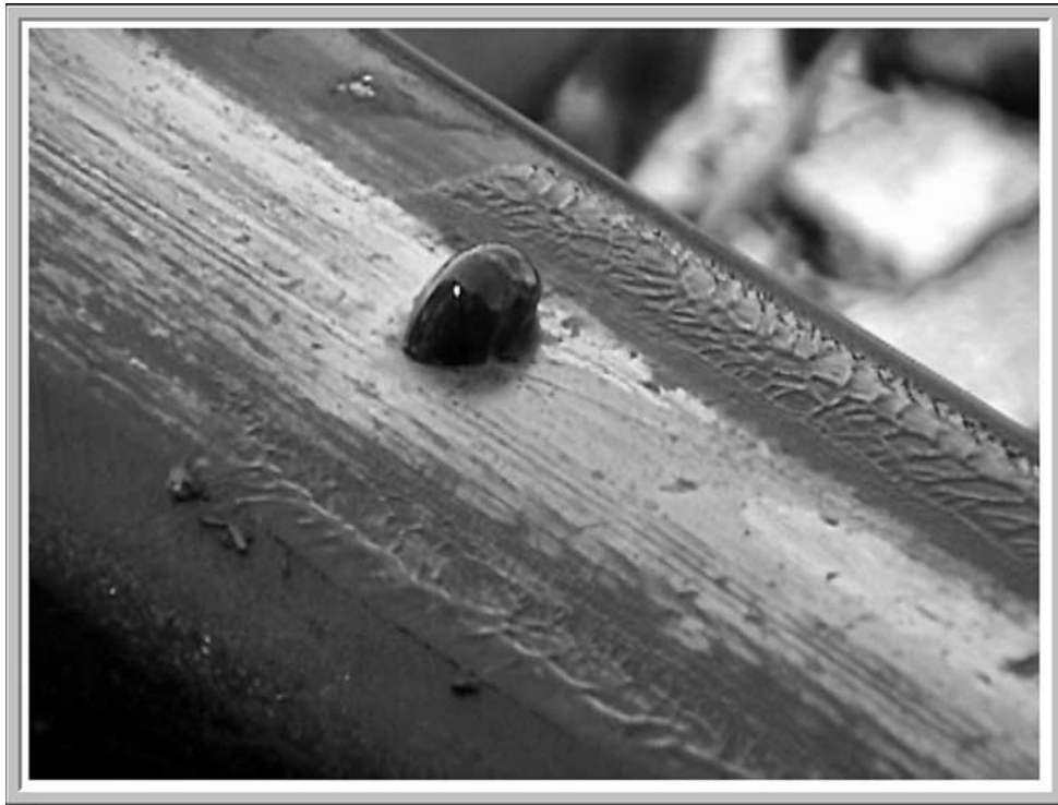
Figure 17—TOR at point of lubrication showing extruded bead of grease.
