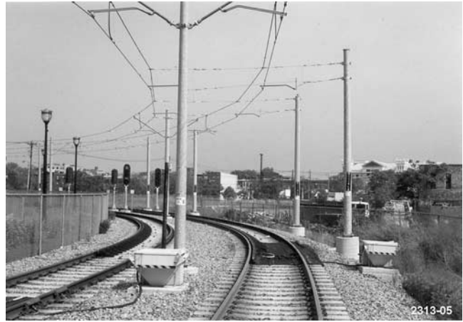
Figure 19. Site with soybean-based lubrication applied for gage face and restraining rail wear protection (right track) and friction control material applied to the top of the running rail (left track).
