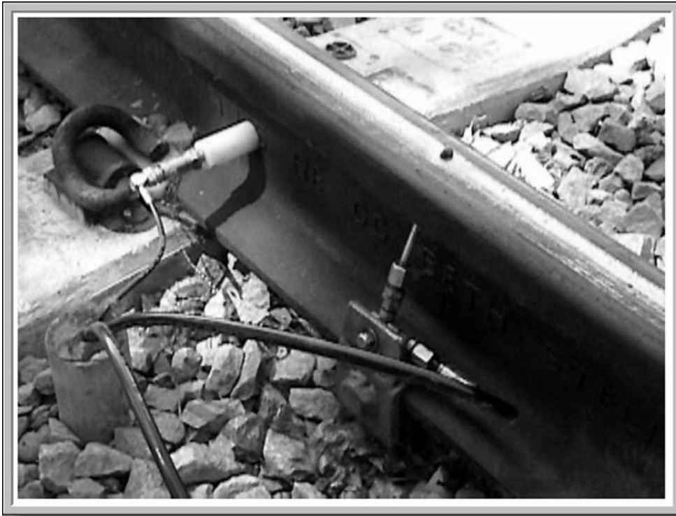
Figure 18—TOR at point of lubrication showing pressure feed tubes leading to rail.
