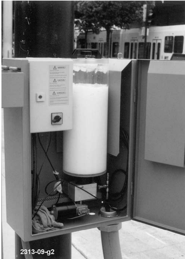
Figure 10. Interior view of the applicator system, showing grease reservoir.
