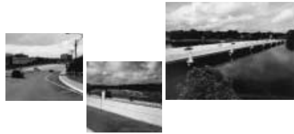
FIGURE 3 Navesink River Bridge, Route 35.
