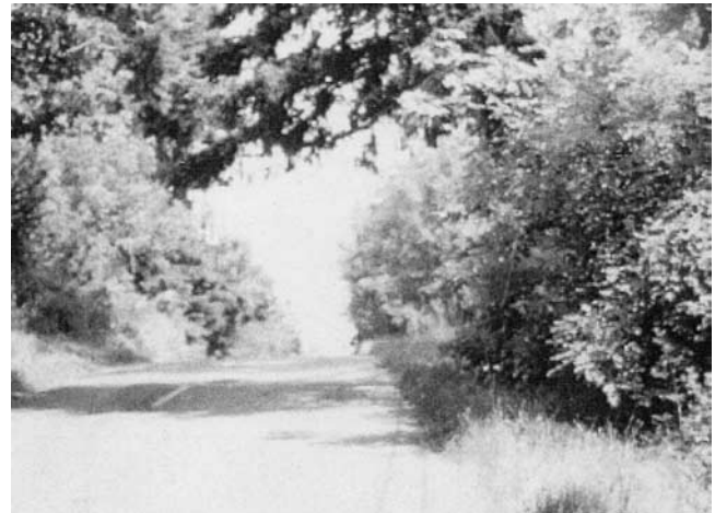
FIGURE 2 Uncontrolled encroachment of vegetation on a rural highway (courtesy: John Cantlon, E. I. DuPont Co.).
