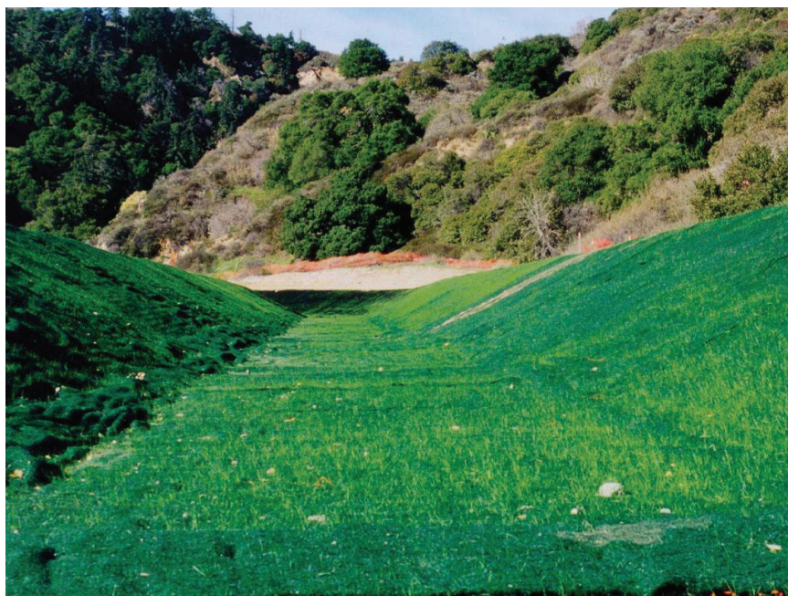
FIGURE 2.2 Geosynthetically stabilized vegetated drainage channel. Sunshine Canyon Landfill, Sylmar, California (photo courtesy of SI Geosolutions).
