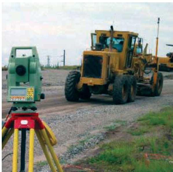
FIGURE 2.4 Laser-guided earthmover (photo courtesy Lecia Geosystems, http://www.leica-geosystems.com ).
