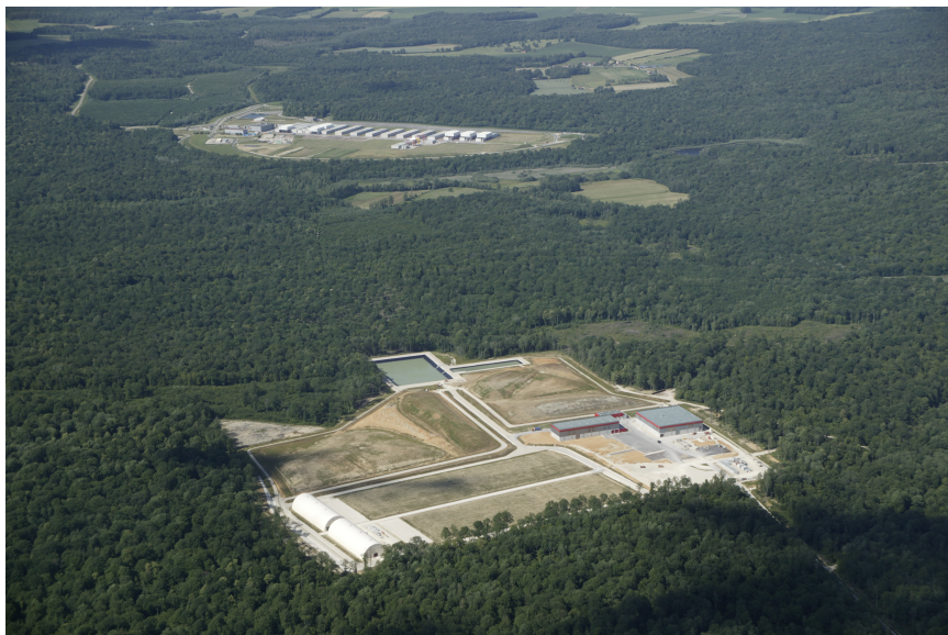
FIGURE 2.1 The Morvilliers, France, site (foreground) is the world's first facility designed especially for disposing of very low activity radioactive wastes. Low- and intermediate-activity short-lived wastes are disposed of at the Centre de l'Aube (background). These facilities are located about 250 kilometers east of Paris.
