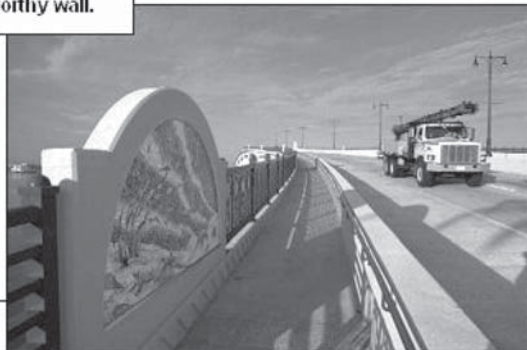
Examples of steel rails were typically protected by a wall. In most cases, they were used in conjunction, located on a low traffic speed street.
