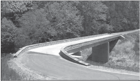
Most of the unique designs were located in scenic areas where traffic speeds and traffic counts are quite low. This stone railing from Kentucky is a good example.
