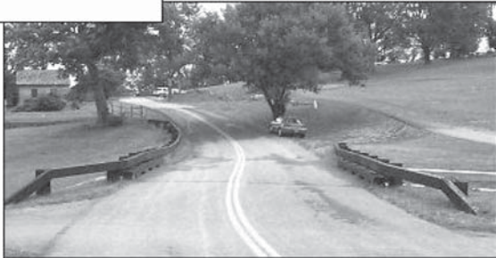
This culvert bridge is located near a golf course in Kentucky but is interesting for its craftsmanship and ingenuity. This is a steel-backed timber railing.
