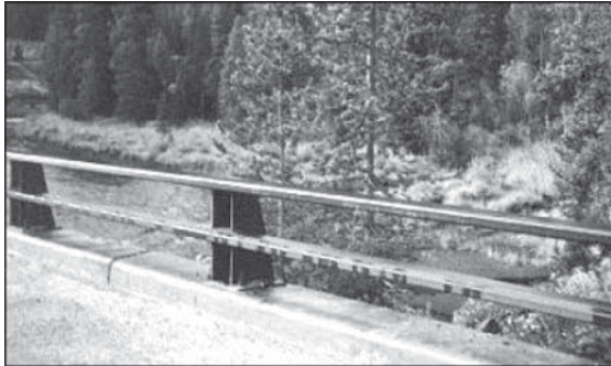
This Wyoming Rail from Virginia is a good example of the reason for a see-through rail. The rail is also suitably unassuming.
