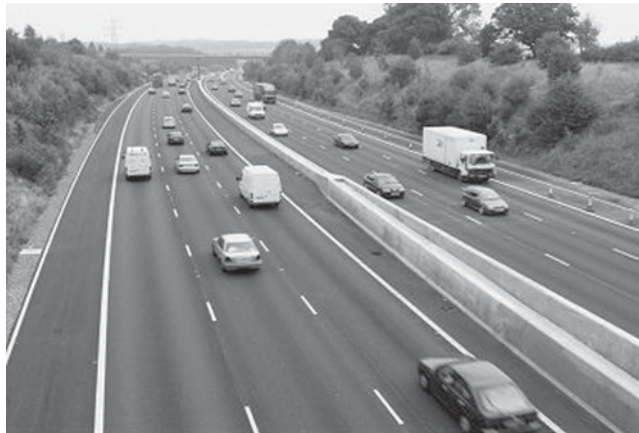
Figure 7. Concrete barriers used in the United Kingdom.
