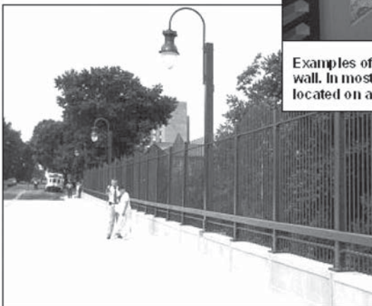
This rail is another example of a popular method to create attractive rails in urban areas. This Virginia project is located in low-traffic-speed street.
