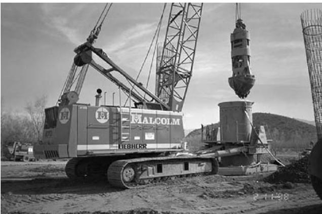
FIGURE 49 Casing oscillator and hammergrab tool.
