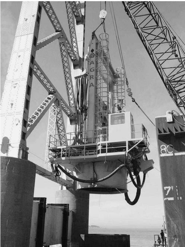
FIGURE 56 Toledo T40-4 pile top unit being placed over casing for reverse circulation drilling, Richmond–San Rafael Bridge (California) (Byles 2004).
