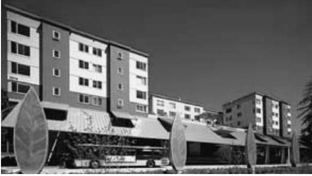
FIGURE 16 Transit facility serves the Overlake (Washington State) housing development (Courtesy: The Allied Group, Inc., Renton, Washington.)
