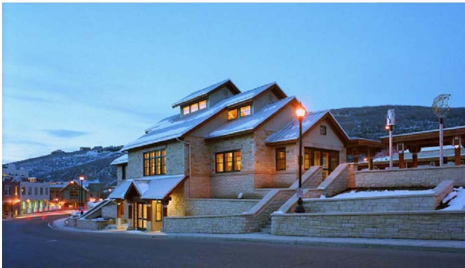
FIGURE 2 The Park City Transit Center in Utah respects the surrounding area's historical and topographical contexts.
