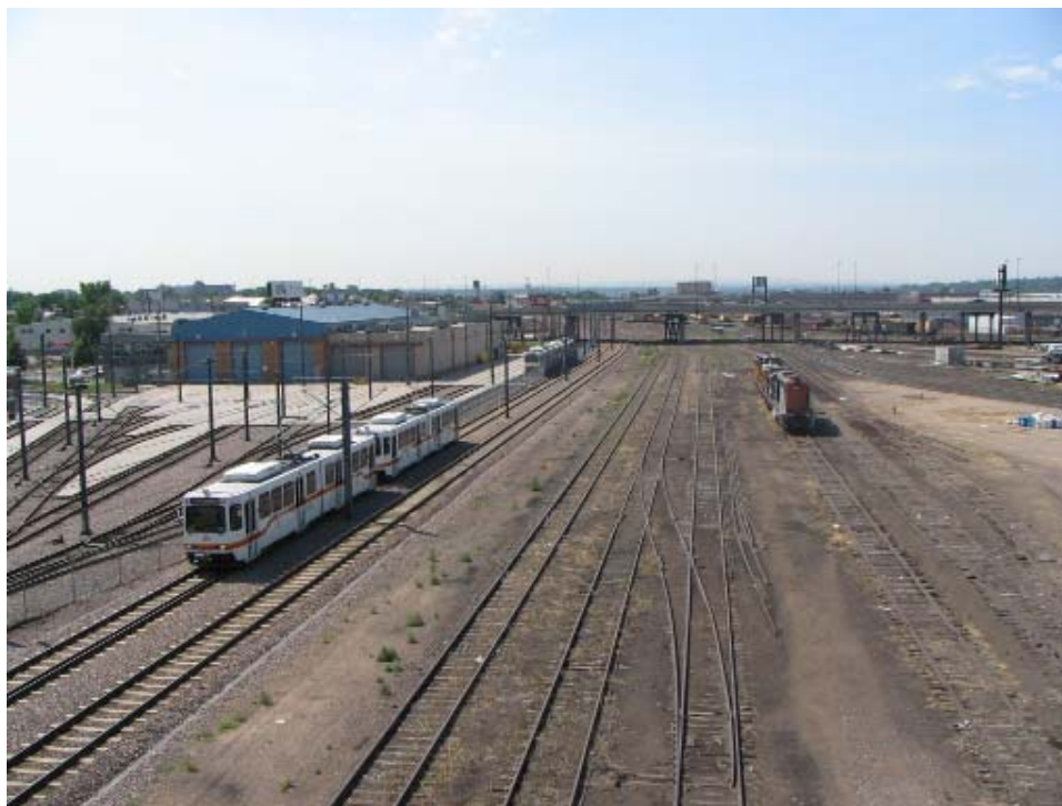
FIGURE 5 Central Corridor and Burnham Yard.
