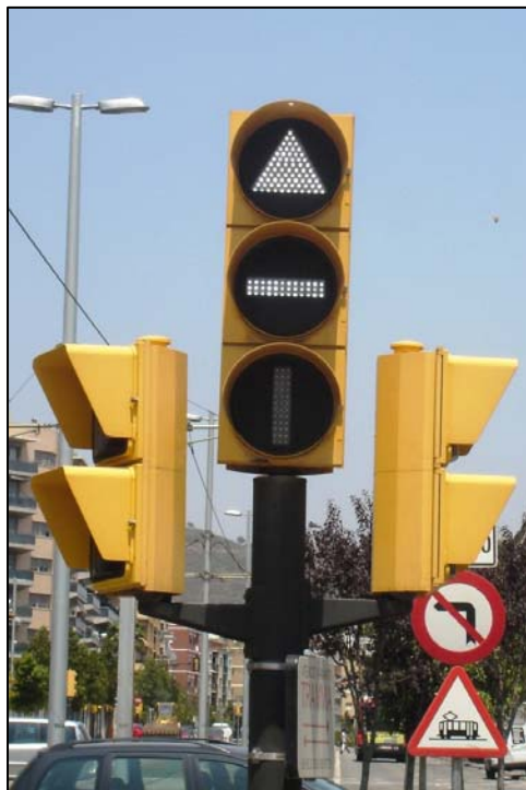
FIGURE 22 LRT signal indication (LRV Detected/Stop/Proceed), Barcelona, Spain.
