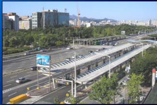
Yeouido Transfer Center
