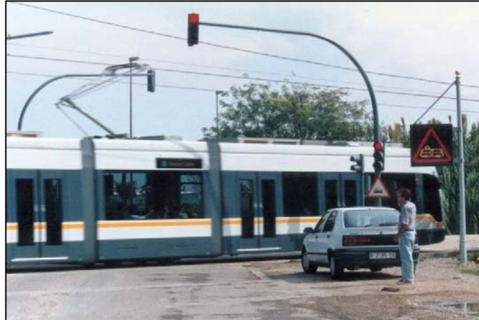
FIGURE 17 LRV-activated, internally illuminated warning sign at midblock motor-vehicle crossing, Valencia, Spain (suburban environment, separate ROW operation).
