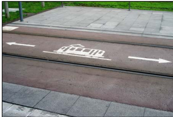
FIGURE 12 LRV directional striping (warning) on a two-way track, Barcelona, Spain (urban environment, median operation).
