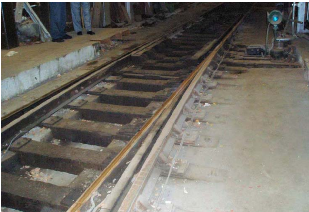
FIGURE 8 Fully guarded switch with added house top protection.
