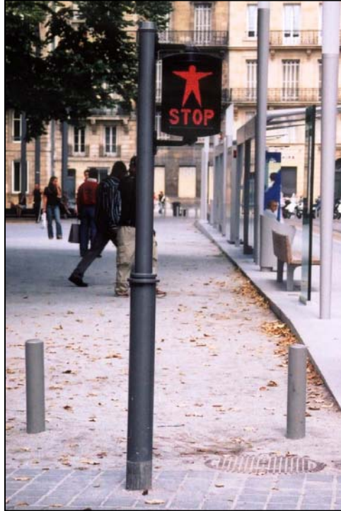
FIGURE 8 LRV-activated pedestrian signal (regulatory), Bordeaux, France (urban environment, pedestrian mall operation).
