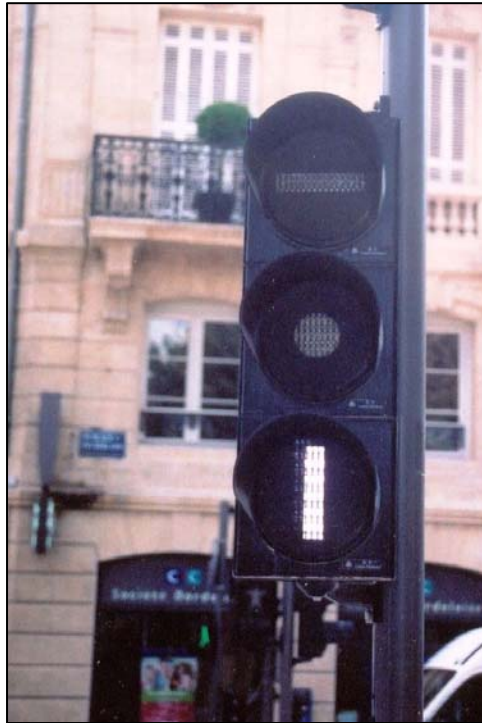
FIGURE 21 LRT signal indication (Stop/Prepare to Stop/Proceed), Bordeaux, France.
