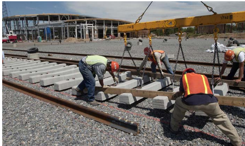
FIGURE 3 Resalvaged materials—including steel from the old Mile High Stadium—were reused at Elati.
