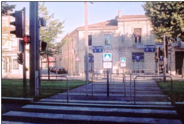
FIGURE 13 Bedstead barrier midblock crossing (regulatory), Bordeaux, France (urban environment, median operation).
