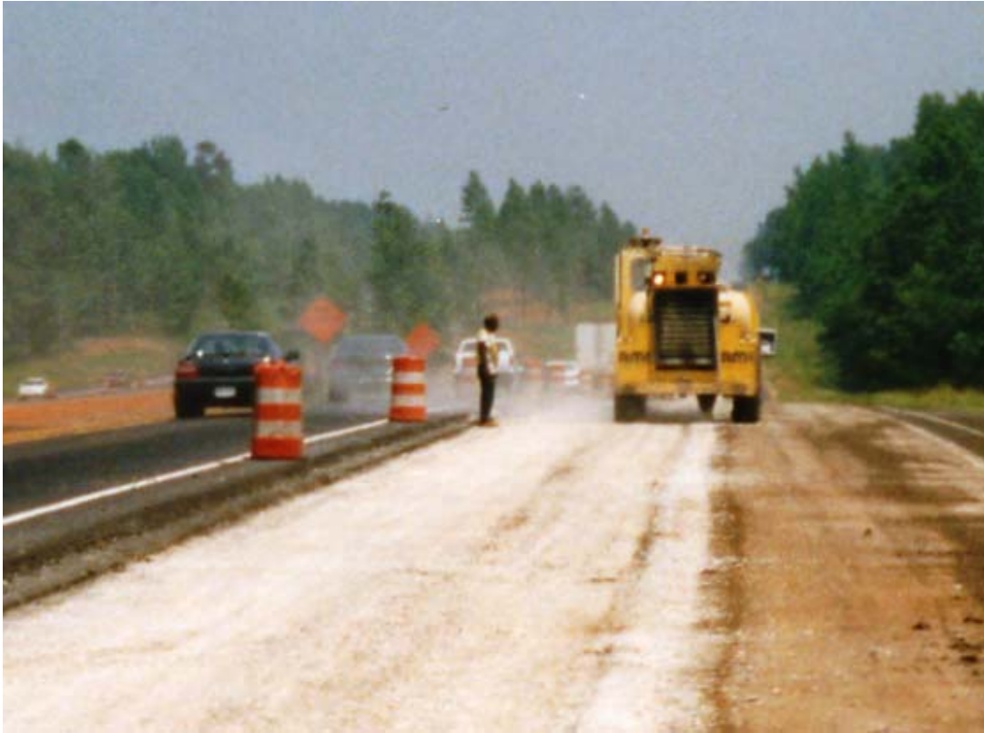
FIGURE 5 Resonant rubblizing starting from pavement edge.
