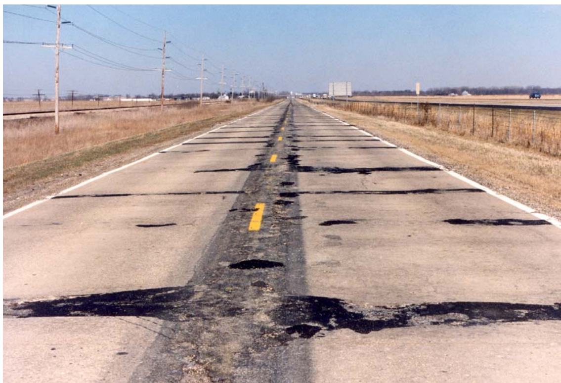
FIGURE 1 Prime candidate project for rubblization.
