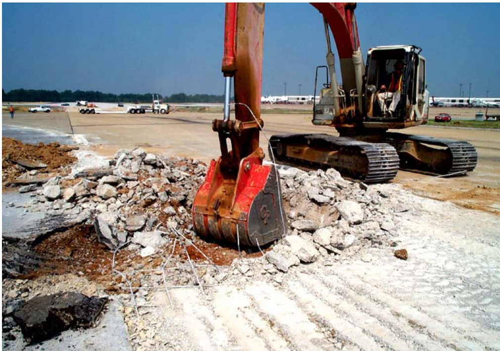
FIGURE 10 Test pit showing complete debonding of steel.
