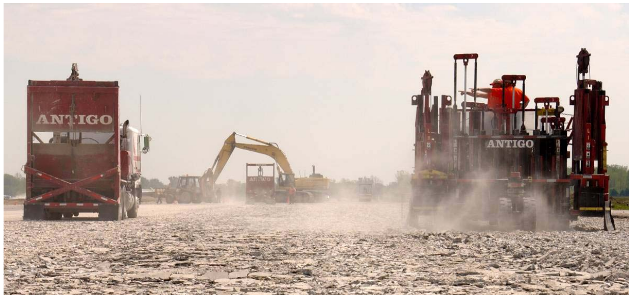
FIGURE 8 Dust generated during rubbleization.
