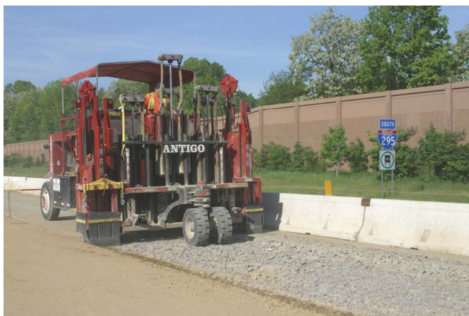
FIGURE 6 MHB for PCC rubblization. (Photo courtesy of Antigo Construction.)
