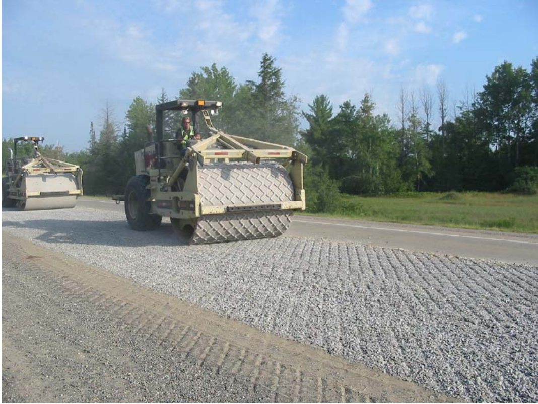
FIGURE 6 A vibratory Z-grid roller followed by a vibratory steel-wheeled roller.
