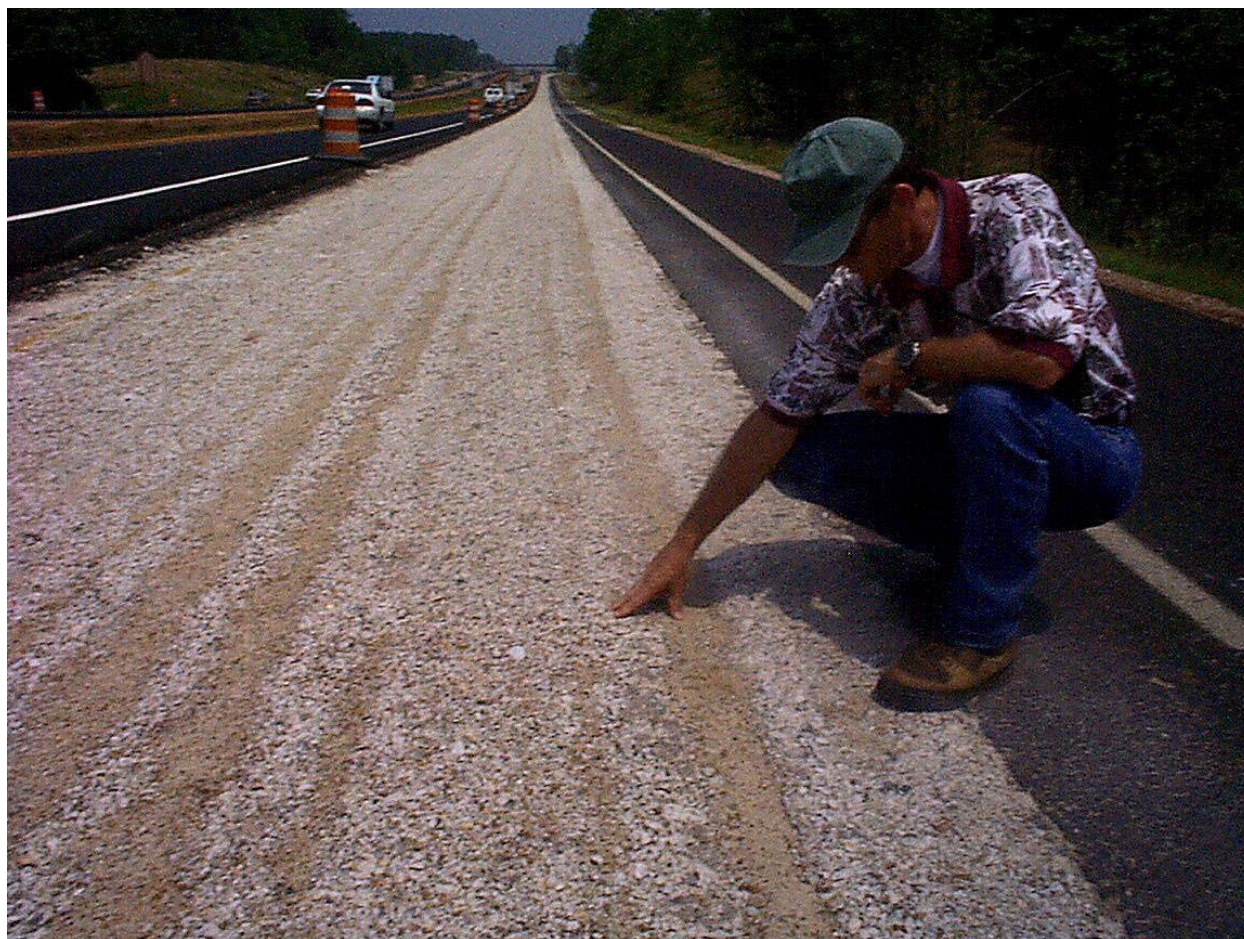
FIGURE 7 Resonant rubblized PCC, before rolling.
