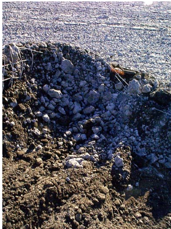
FIGURE 10 Rubblization test hole. (Photo Courtesy of RMI.)
