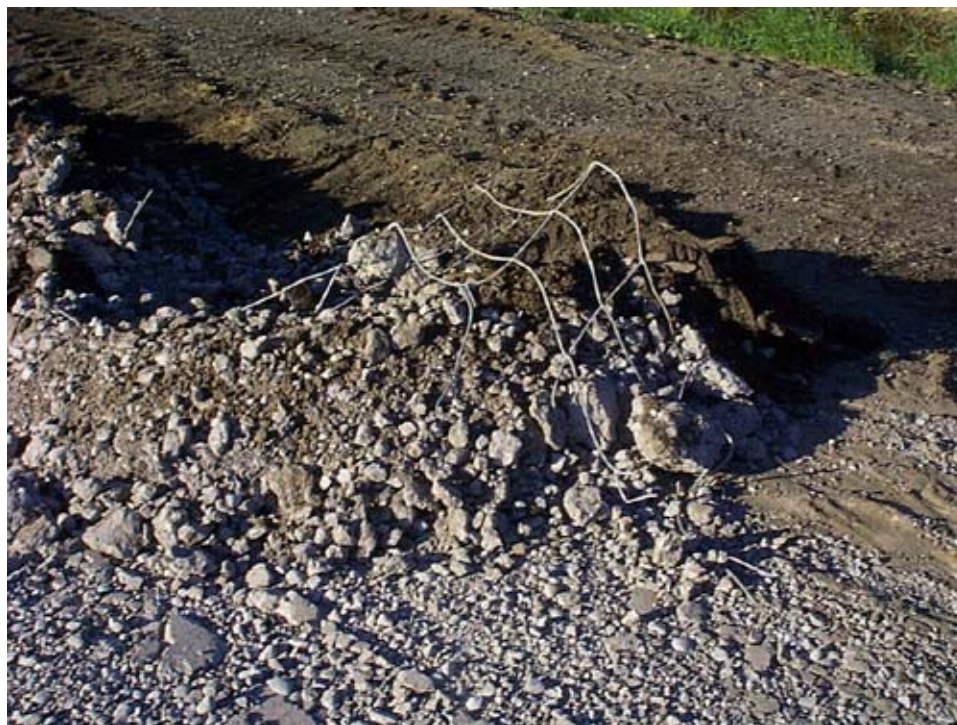
FIGURE 11 Exposed reinforcing steel after rubblization. (Photo Courtesy RMI.)
