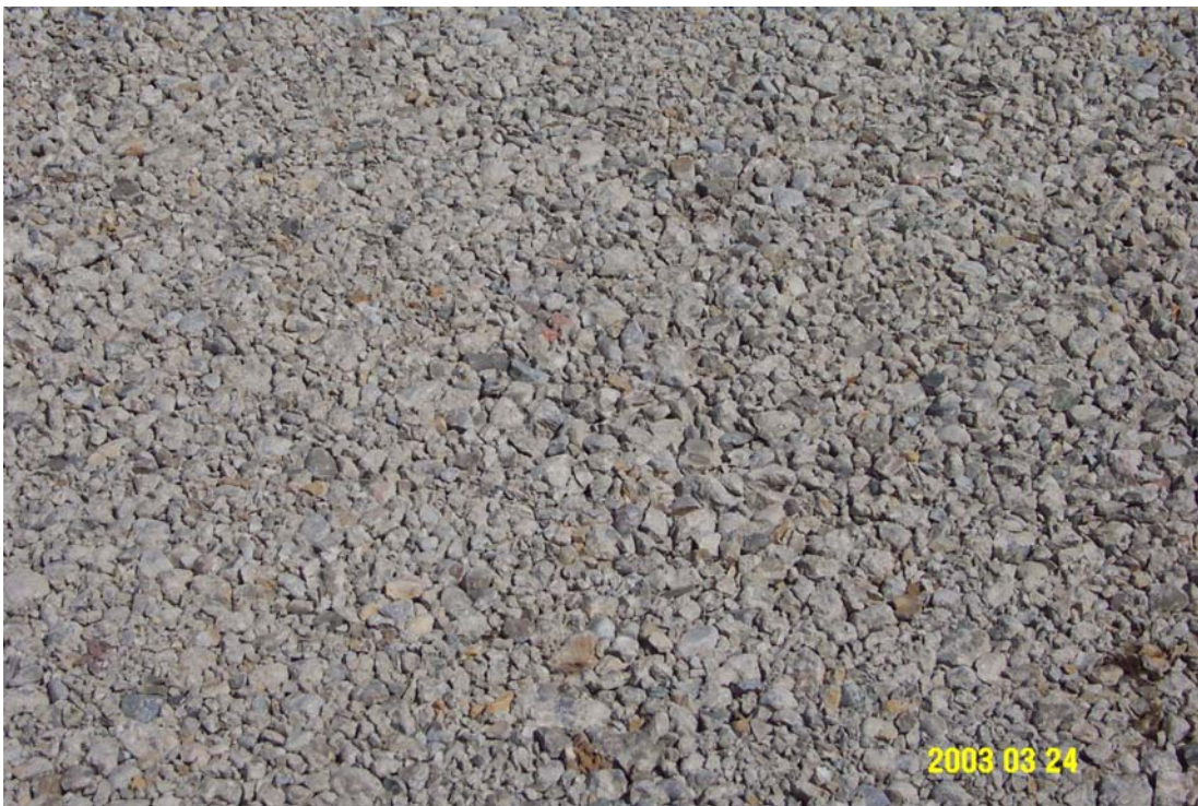
FIGURE 7 The final rubblized and compacted PCC surface.
