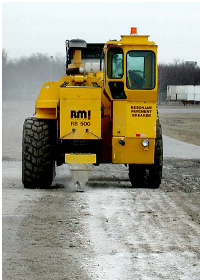
FIGURE 7 RFB for PCC Rubblization. (Photo courtesy of RMI.)
