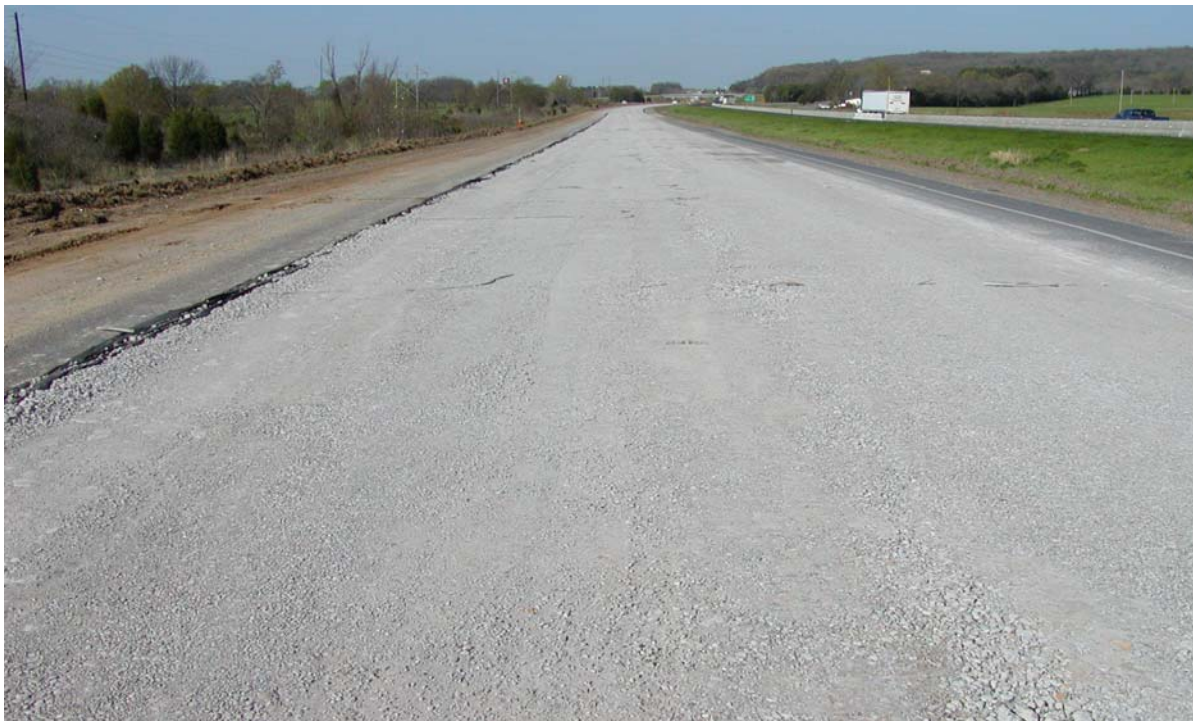
FIGURE 8 Resonant rubblized PCC, after rolling. (Photo courtesy of RMI, Inc.)
