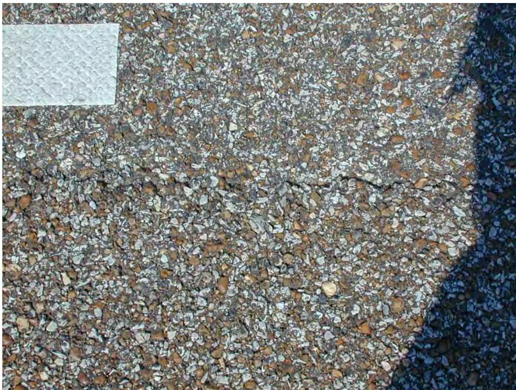
**Figure C9. Centerline Longitudinal Joint, AR-2 after Four Years.**
