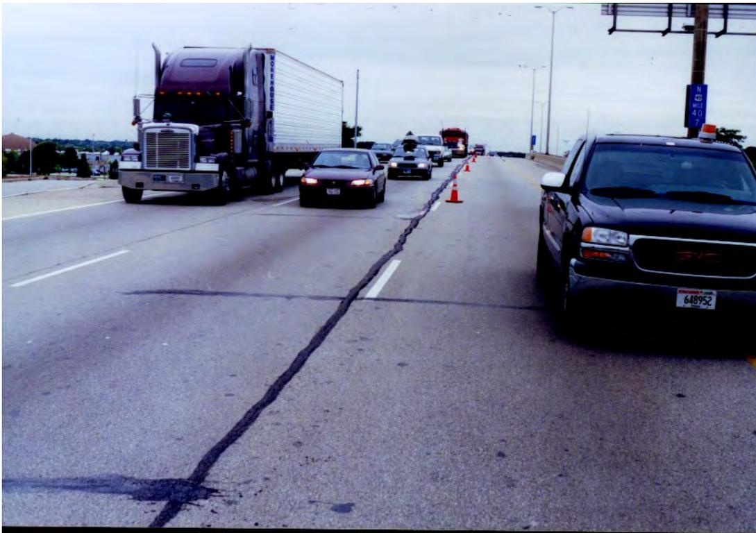
FigureC60. Reflective Cracking WI-1
