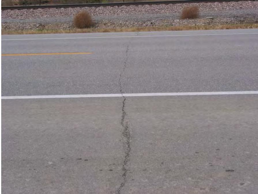
**Figure C53. Thermal Crack after Two Years, NE-2**
