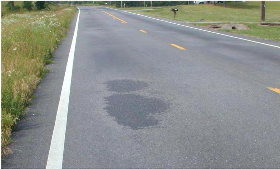
**Figure C2. Wet Area Indicating Permeability, AL-2 Highway 168 Boaz, AL**
