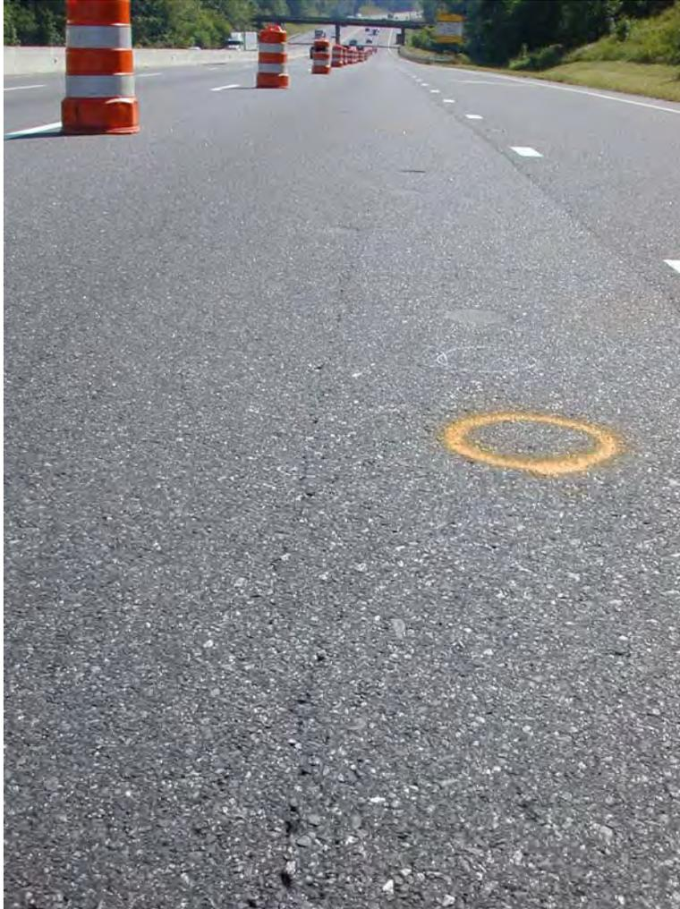
**Figure C50. Longitudinal Crack in Right Wheel-Path NC-1.**
