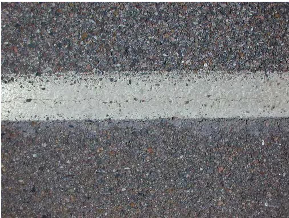
**Figure C36. Edge line Crack with Evidence of Water and Fines KS-1.**
