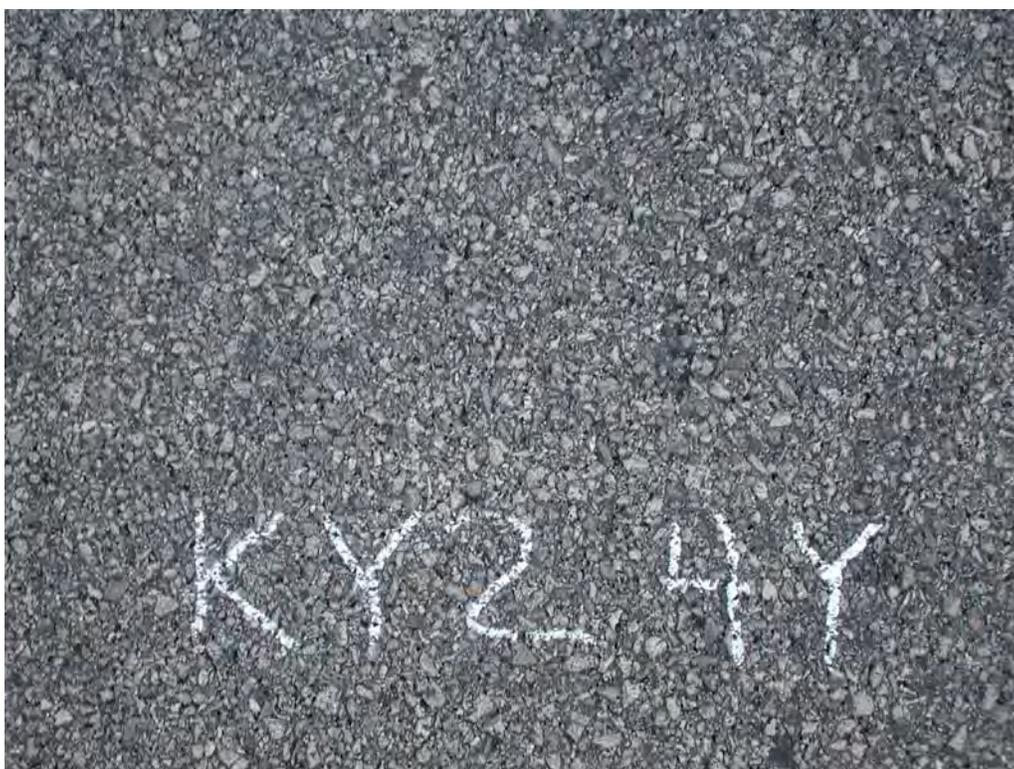
**Figure C41. Surface Texture with Raveling of KY-2.**
