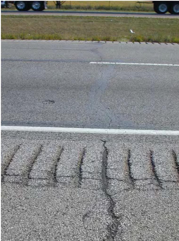
**Figure C34. Transverse Reflective Crack IN-2.**
