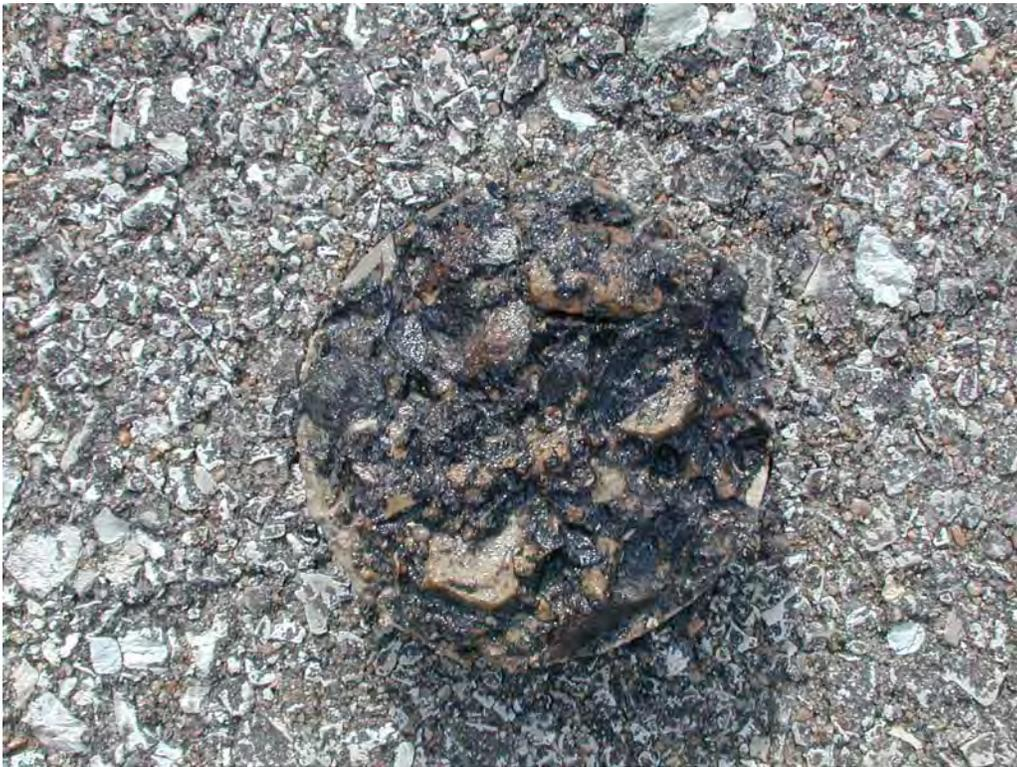
**Figure C31. Moisture Damage in Underlying Layer.**
