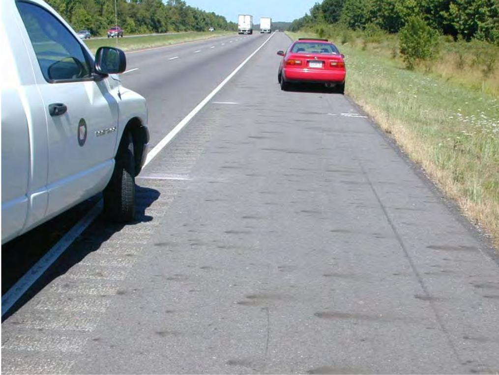
**Figure C6. Rust Spots evident in AR-1, I-40 West of Conway, AR.**
