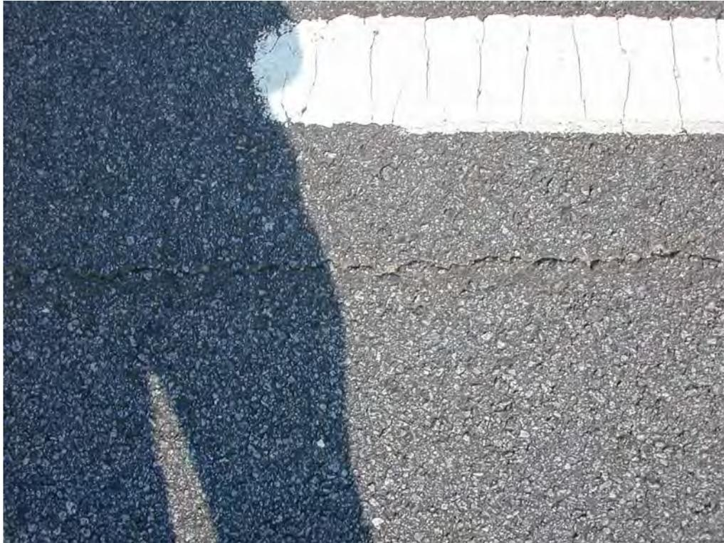
**Figure C24. GA-1 Longitudinal Joint after Two-Years.**
