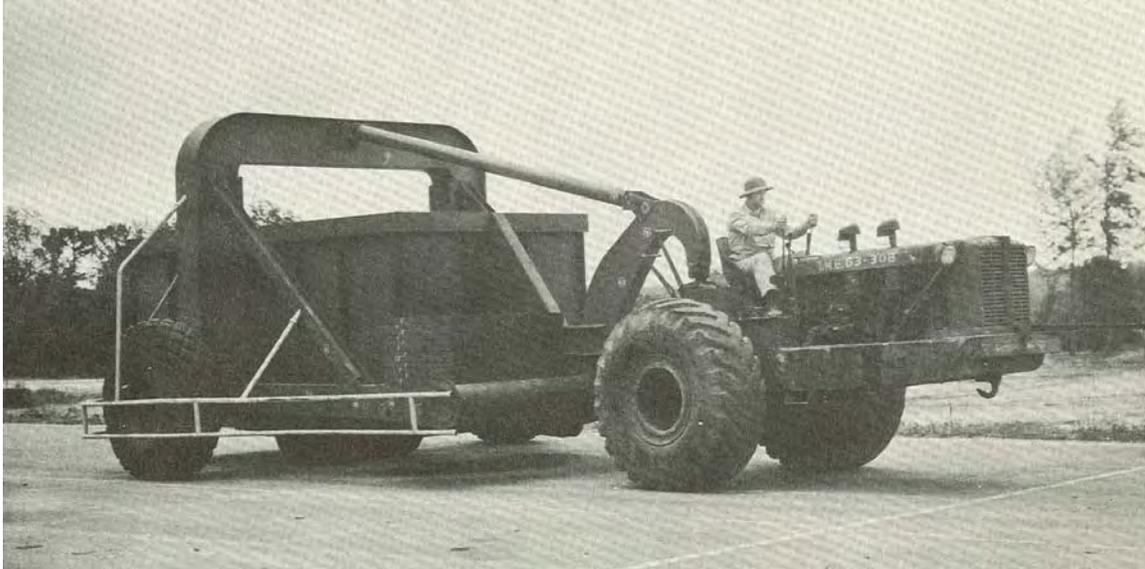
**Figure A.2. Model C Tournpull with Specially Built Loading Cart (10).**
