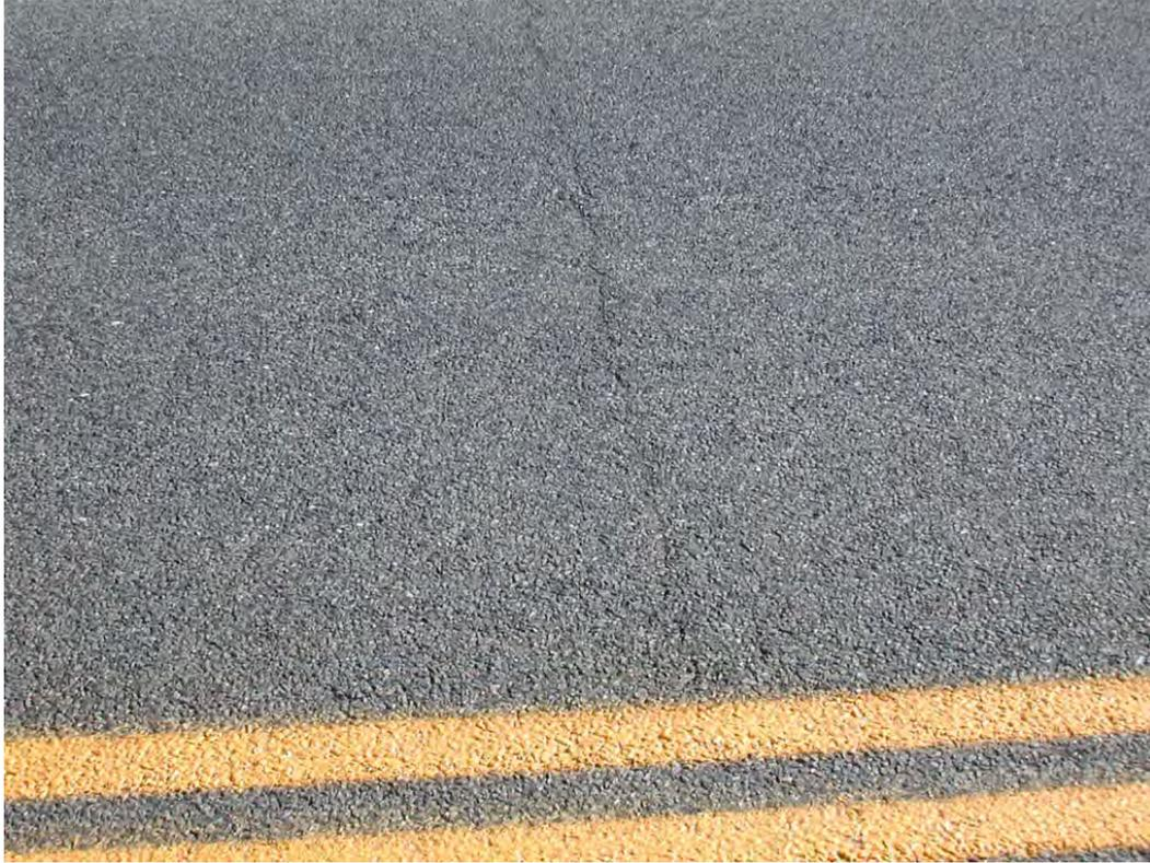
**Figure C58. Transverse Crack, UT-1.**
