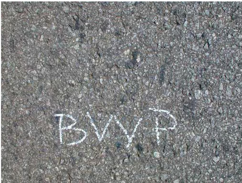
**Figure C26. Close-up of GA-1 Surface Texture after Four-Years.**
