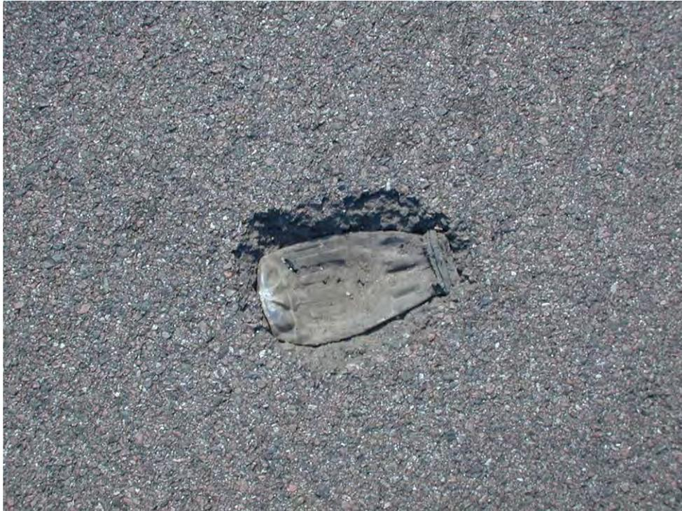
**Figure C23. Small Pothole Caused By Bottle Paved into Pavement, FL-1**
