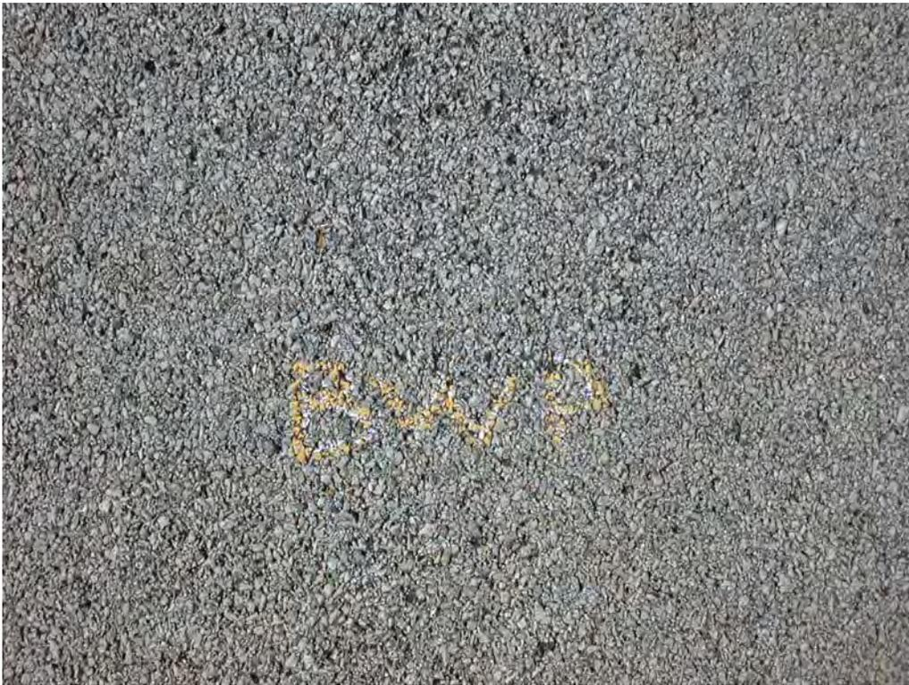
**Figure C28. Minor Raveling between Wheel Paths, IL-1.**
