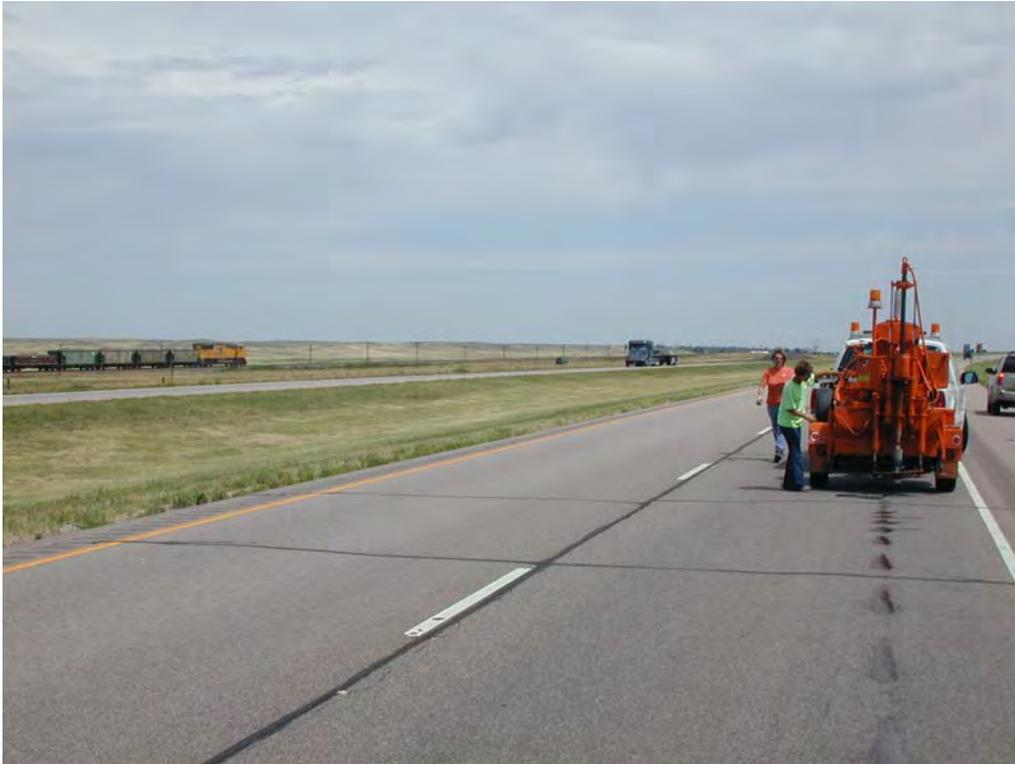
**Figure C56. Transverse Crack NE-4 after Four Years.**
