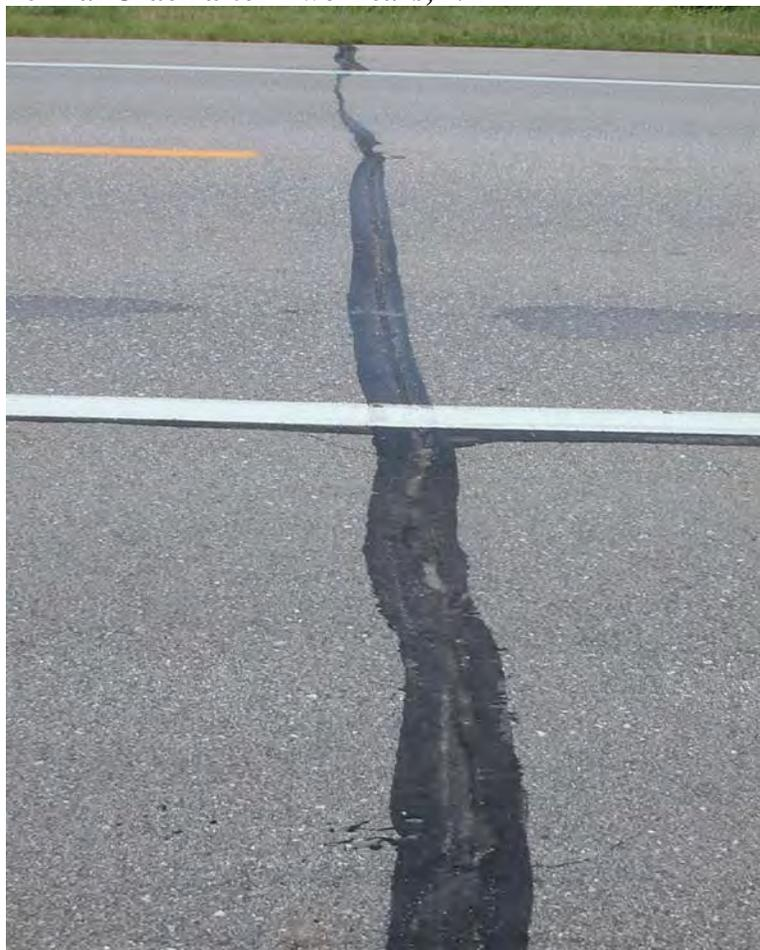
**Figure C54. Sealed Thermal Crack after Four Years NE-2**
