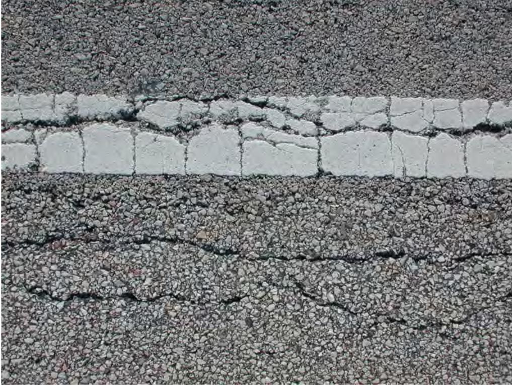
**Figure C27. Longitudinal Cracking along Shoulder IL-1, I-57, Gilman, IL.**
