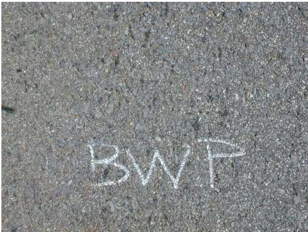
**Figure C57. Low Severity Raveling between Wheel-path (and elsewhere), TN-1.**
