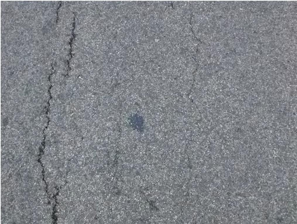
**Figure C33. Longitudinal Cracking Site 3, IN-1.**
