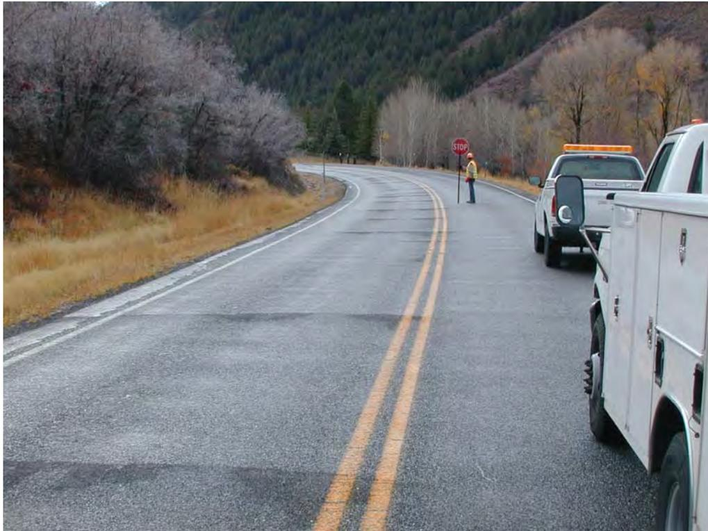
**Figure C59. Transverse Cracking in Westbound (non-test) Lane UT-1.**
