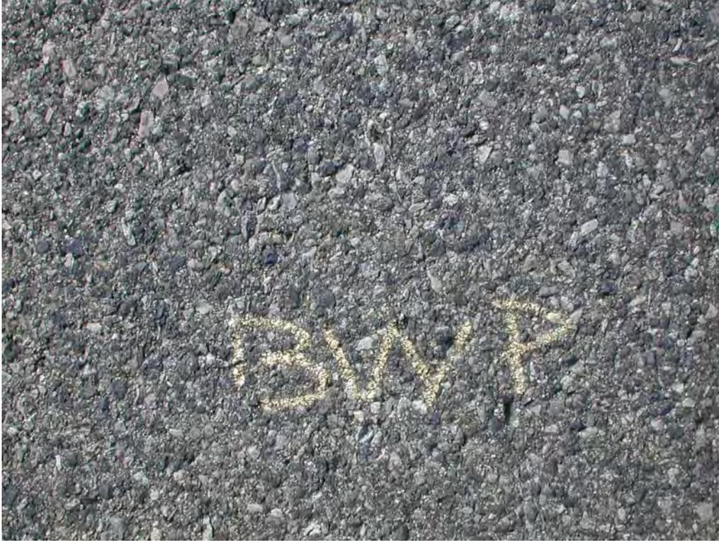
**Figure C35. Pavement Texture between Wheel-paths for IN-2.**
