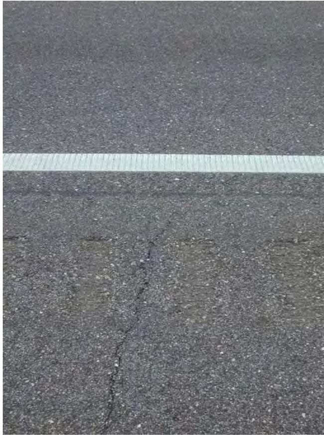
**Figure C3. Transverse Crack in Shoulder, AL-3 Whitehall, Alabama**
