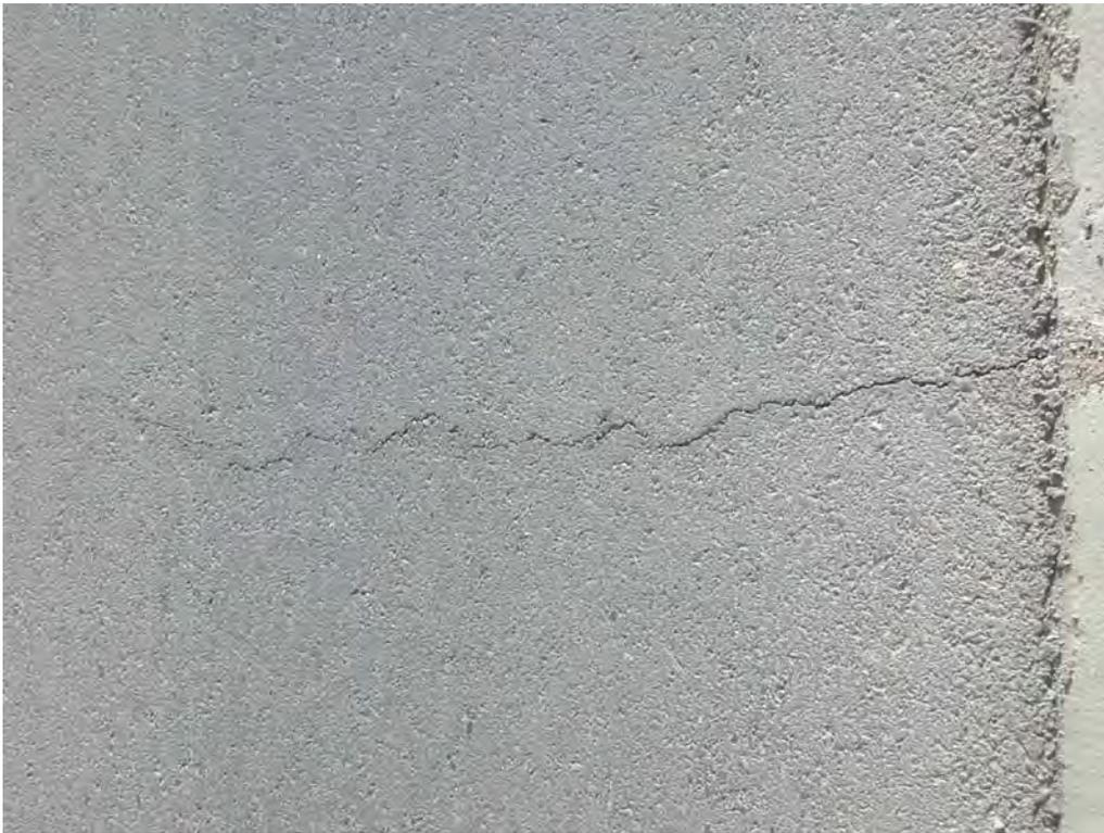
**Figure C19. Transverse Crack CO-3.**
