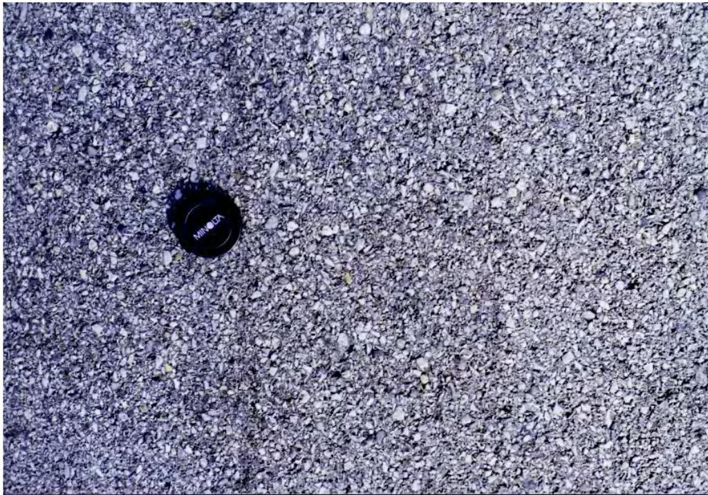
**Figure C45. Longitudinal Joint (Right Edge of Lens Cap) and Surface Texture, MI-1**
