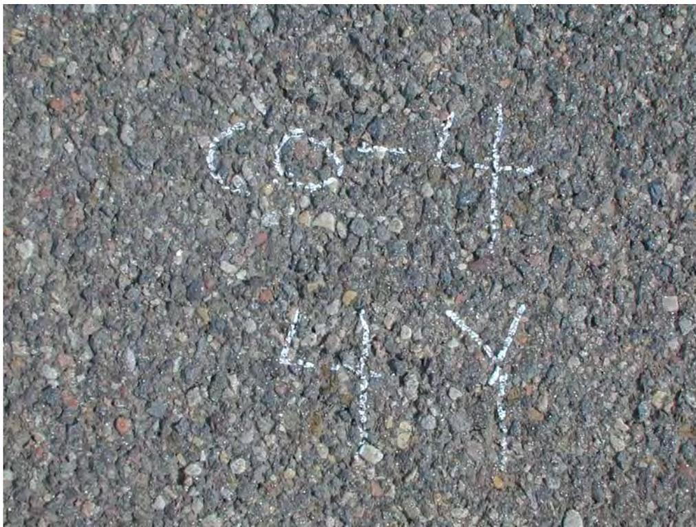
**Figure C21. Close-up of CO-4 Surface Texture after Four Years.**
