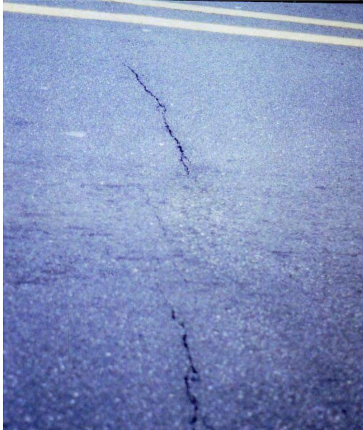
**Figure C47. Reflective Crack, MI-3**
