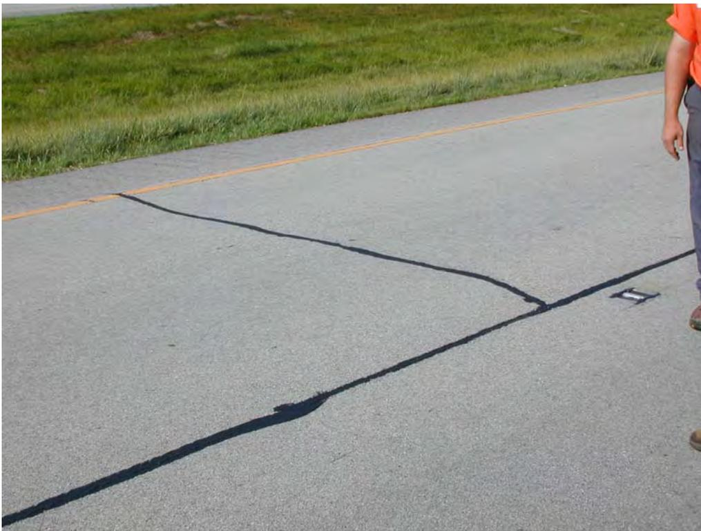
**Figure C32. Sealed Reflective Crack IL-3.**
