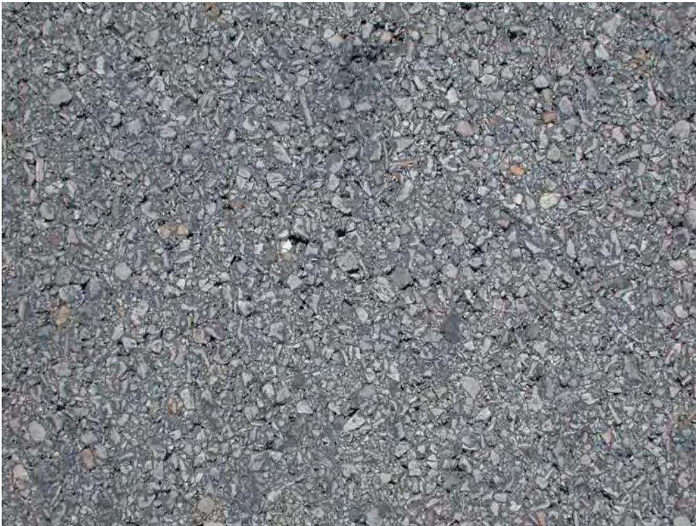
**Figure C7. Close-up of AR-1 Surface Texture after Four Years.**
