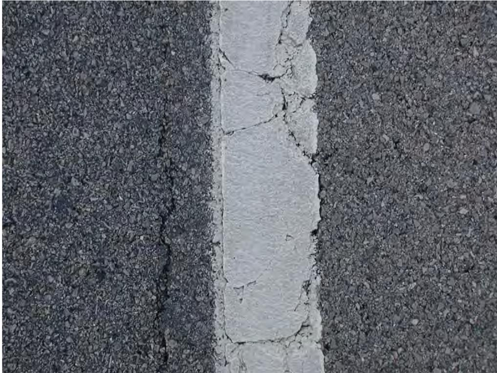
**Figure C49. Cracking at Edge of Pavement MO-3.**
