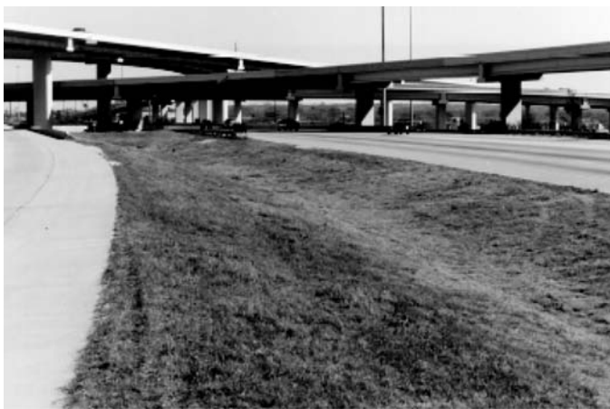
Figure 8-1. Vegetated filter strip at U.S. 183 site.
