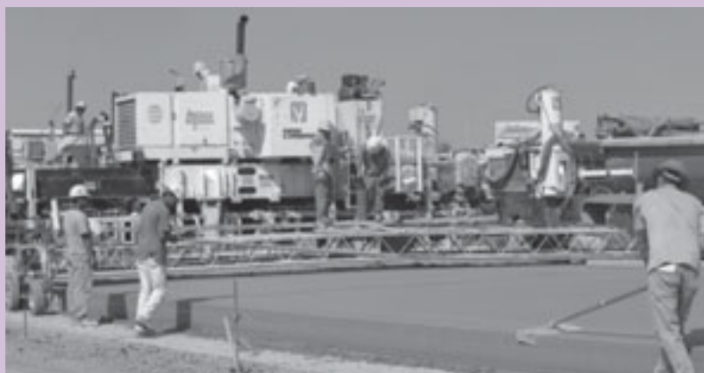
Reconstruction of I-70 pavement near Salinas.
