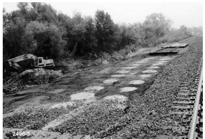
Figure 15 Stone columns installed in approach subgrade.
