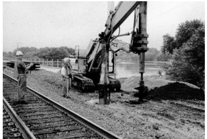
Figure 14 Hole boring in approach subgrade for stone column.
