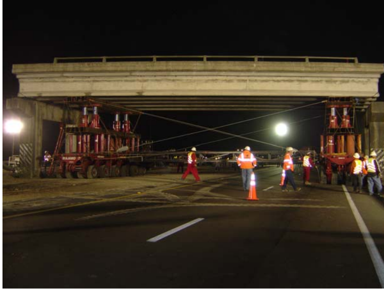
FIGURE 11 Complete bridge change-out.
