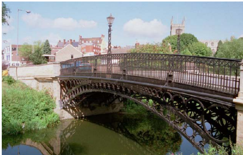
FIGURE 18 The cast-iron Tickford Bridge in Newport Pagnell, United Kingdom ( http://www.telfordsites.co.uk/telford/tickfibr.html ).
