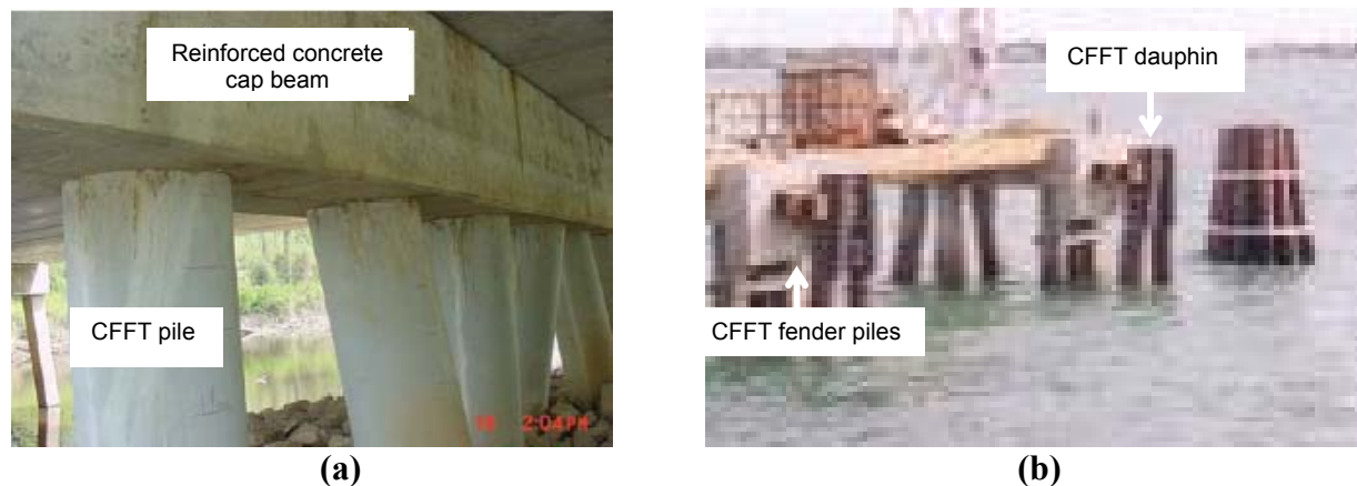
FIGURE 7 Applications of CFFT piles (a) completed Virginia DOT Route 40 bridge pier (Fam et al., 2003b) and (b) fender piles and dauphins at the Ingleside Naval Station (Fam et al., 2003a).
