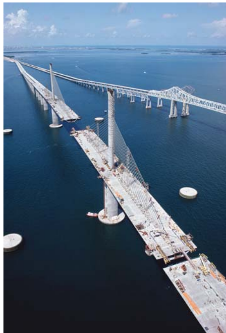
FIGURE 9 Sunshine Skyway construction.
