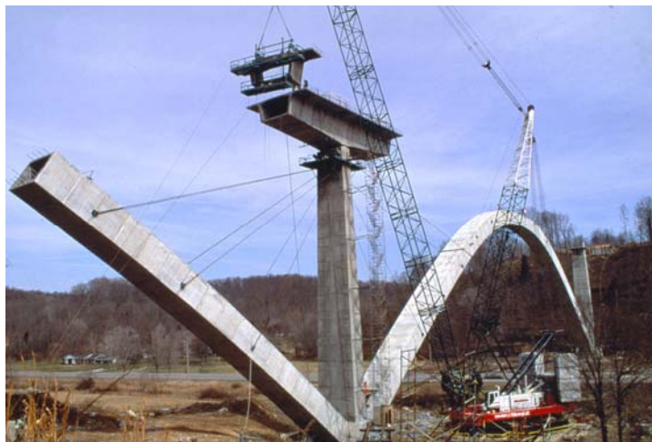
FIGURE 10 Natchez Trace Parkway construction,
