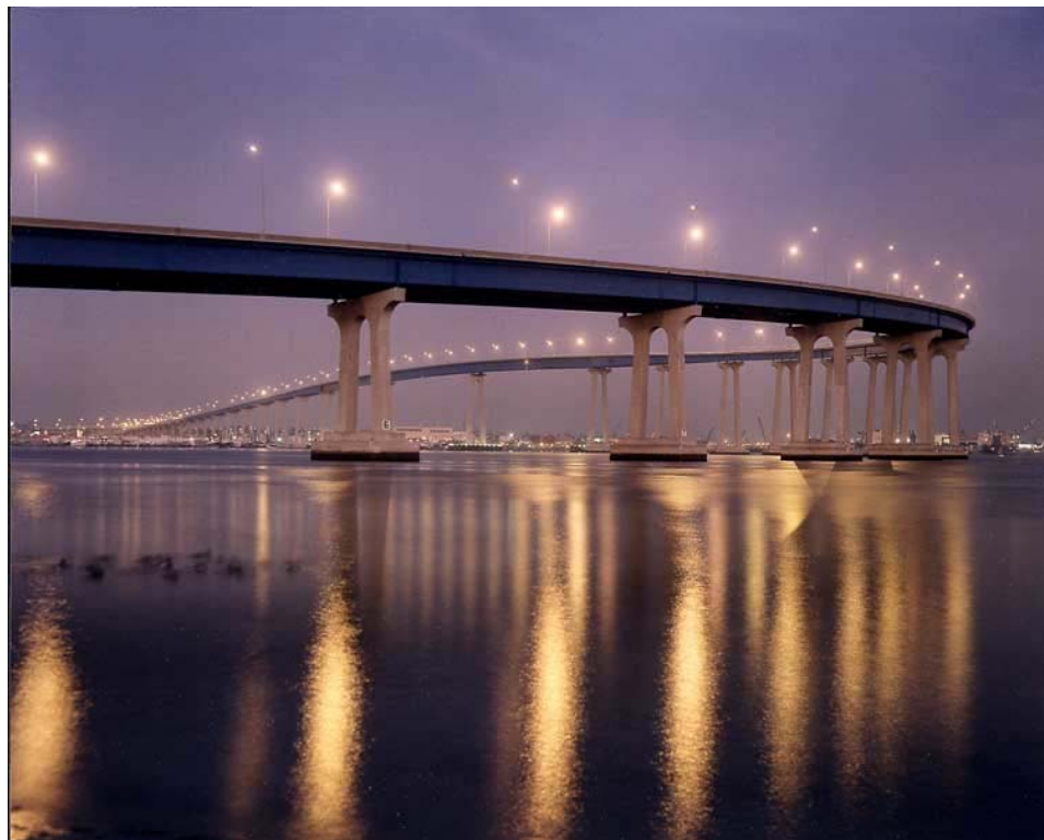
FIGURE 6 The Coronado Bay Bridge in San Diego opened to traffic in 1969, and is arguably the single most important example of a steel box girder bridge. (Photo courtesy of the California Department of Transportation.)
