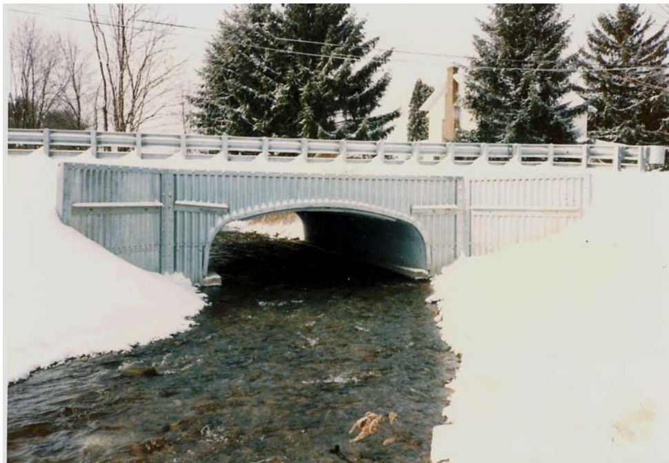
FIGURE 2 Metal box culvert with metal end sections.
