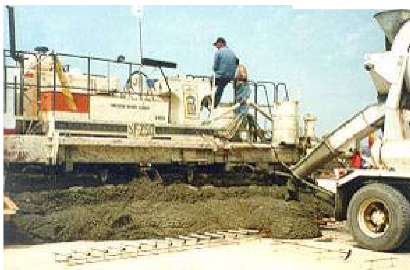
FIGURE 4 Installation of GFRP highway dowels (Gentile et al., 2001).
