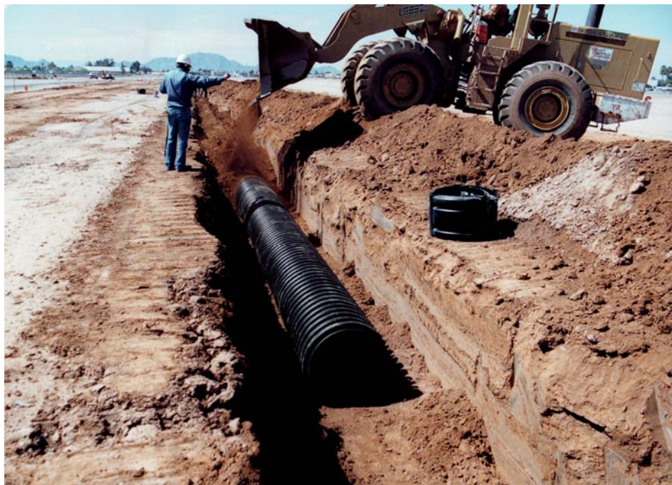
FIGURE 3 Corrugated PE installation.
