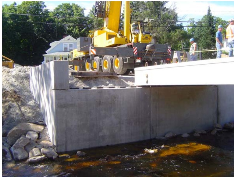
FIGURE 12 Rapid bridge replacement.
