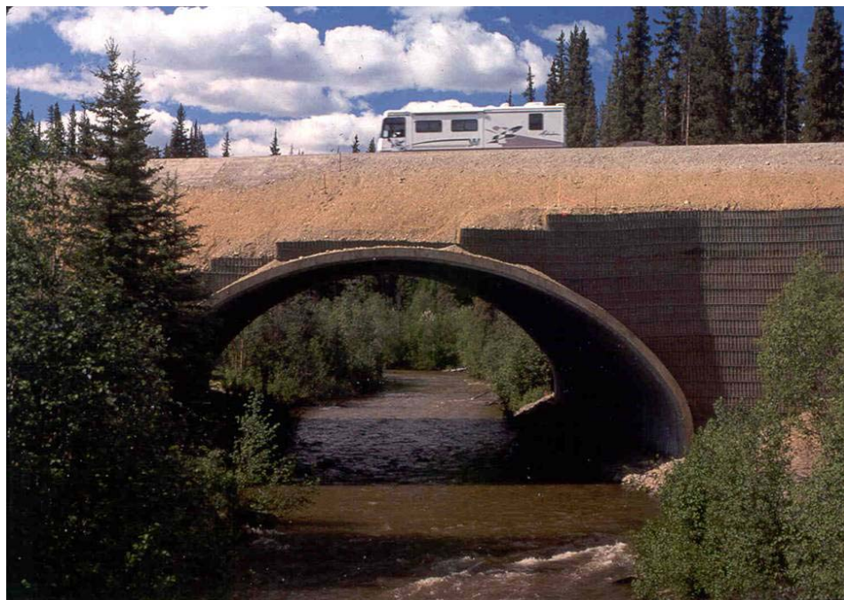
FIGURE 1 Large-span culvert used for stream crossing.
