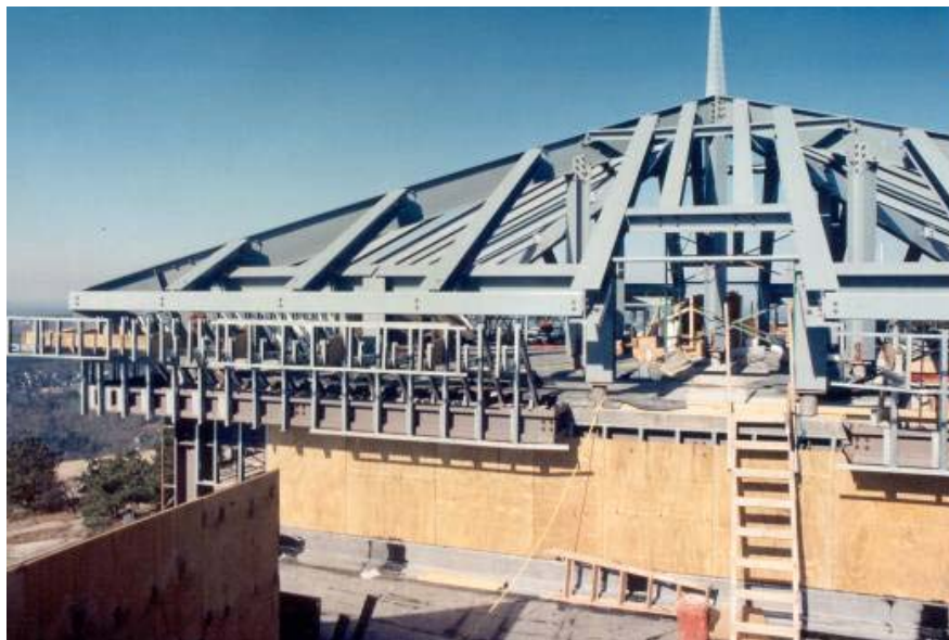
FIGURE 12 Aerial Train Station, FRP roof structure in Stone Mountain, Georgia.
