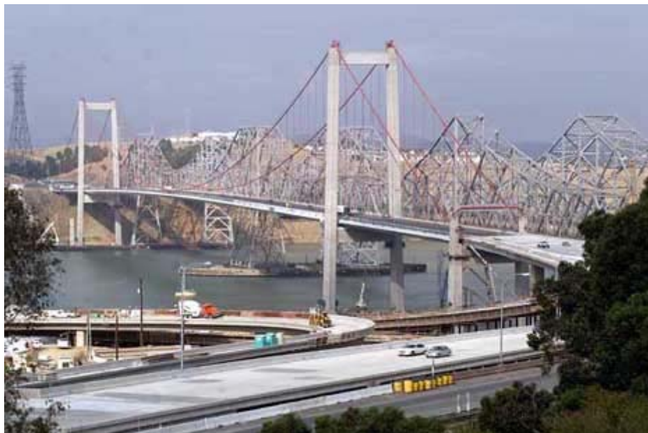
FIGURE 3 The two bridges linking the San Francisco Bay Area and the Sacramento Valley are jointly referred to as the Carquinez Bridge. The three-lane southbound bridge opened in 1927. The northbound bridge, now with four lanes, opened in 1958 and is 200 ft east of the original bridge. In 2003, a new bridge was built just west of the 1927 bridge, replacing the aging span that did not meet standards for seismic design or traffic safety. (Photo courtesy of the California Department of Transportation.)
