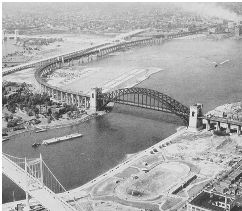
FIGURE 1 The Hell Gate Bridge spanning New York’s East River opened in 1916. (Photo: HAER, en.structurae.de.)
