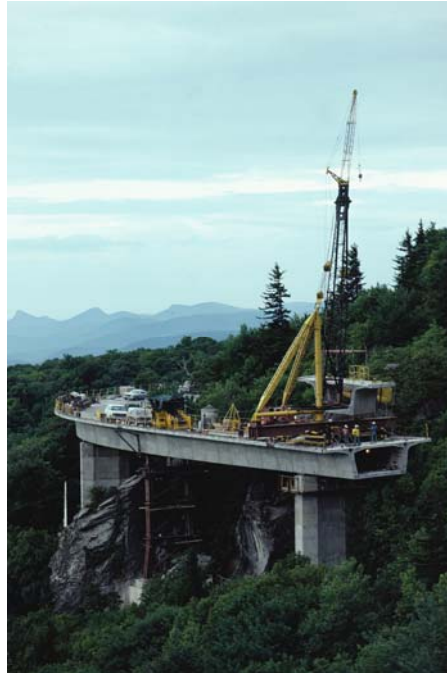
FIGURE 8 Linn Cove Viaduct construction.
