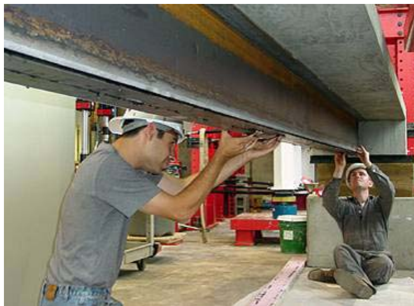
FIGURE 20 Strengthening steel bridge girders with HM CFRP laminates.
