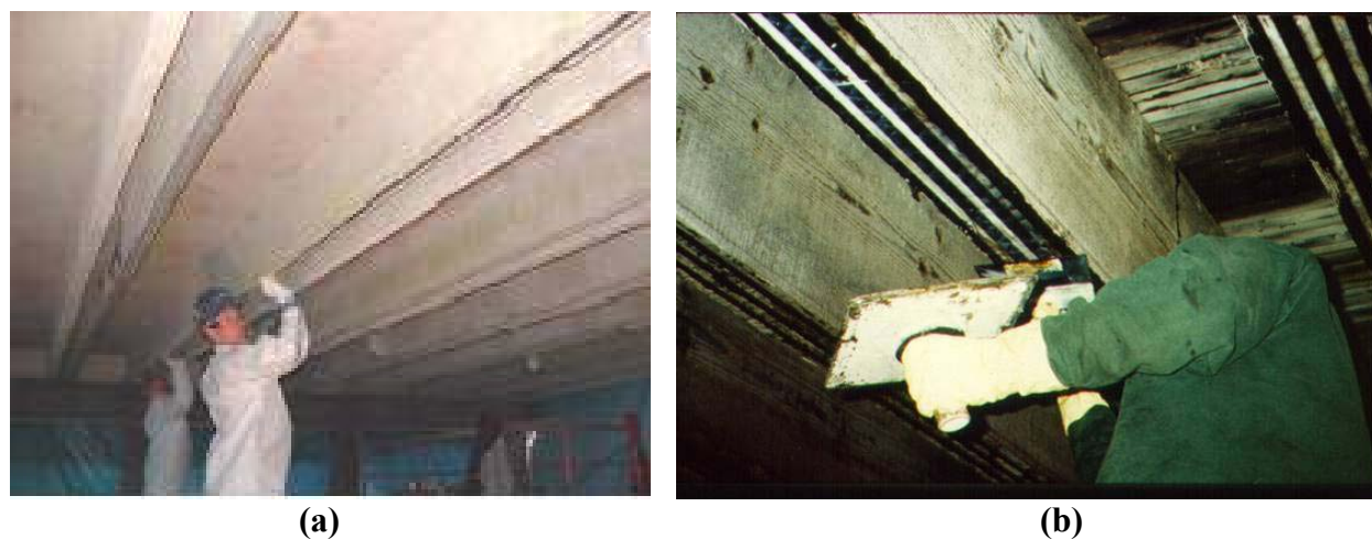
FIGURE 14 NSM strengthening of (a) prestressed concrete beams and (b) timber beams.
