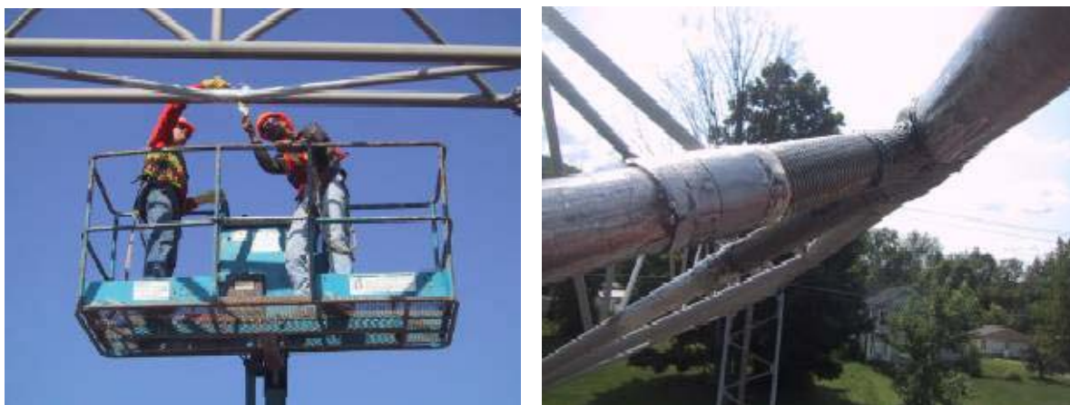
FIGURE 19 Repair of an aluminum overhead sign truss structure (Fam et al., 2005).
