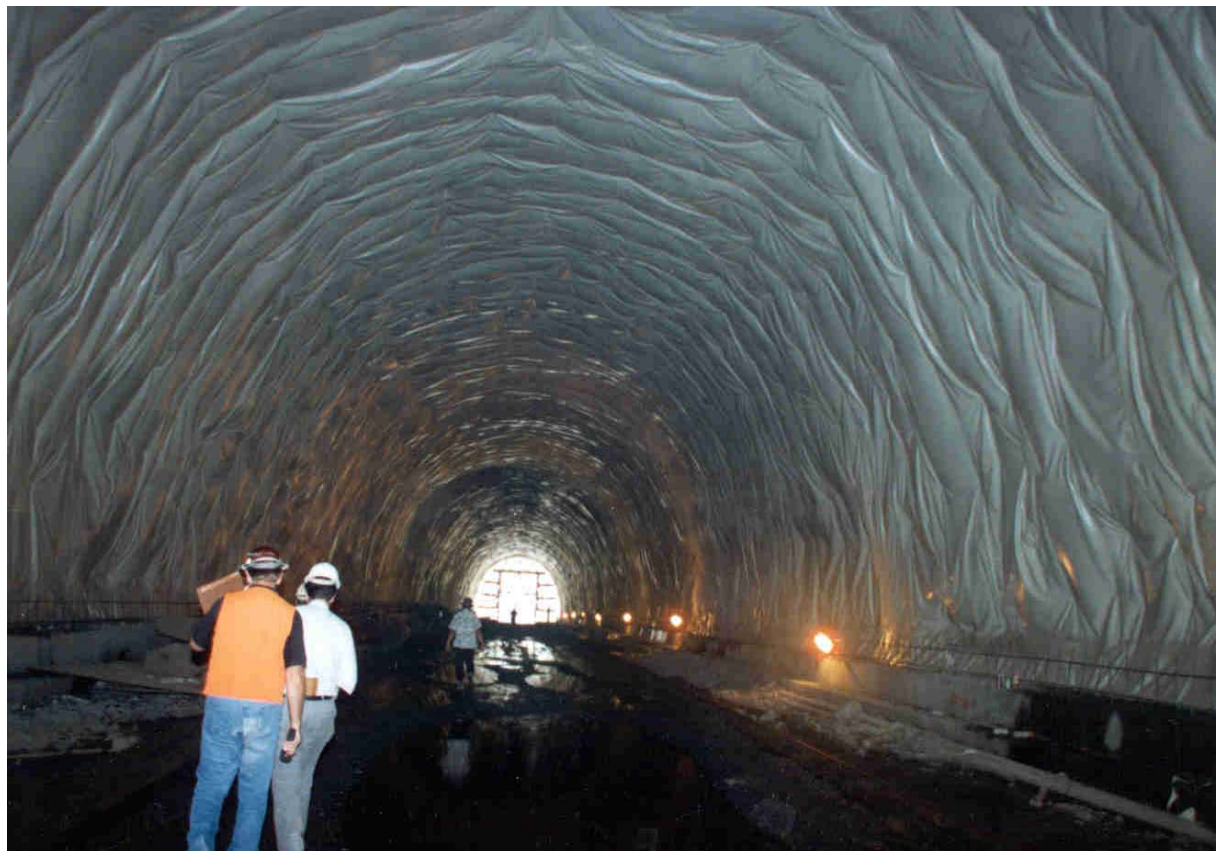
FIGURE 2 Waterproofing membrane installation in Interstate H-3 Trans Koolau Tunnel.
