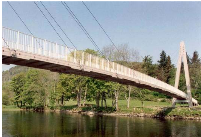
FIGURE 11 Aberfeldy Footbridge across the Tay River in Perthshire, Scotland.
