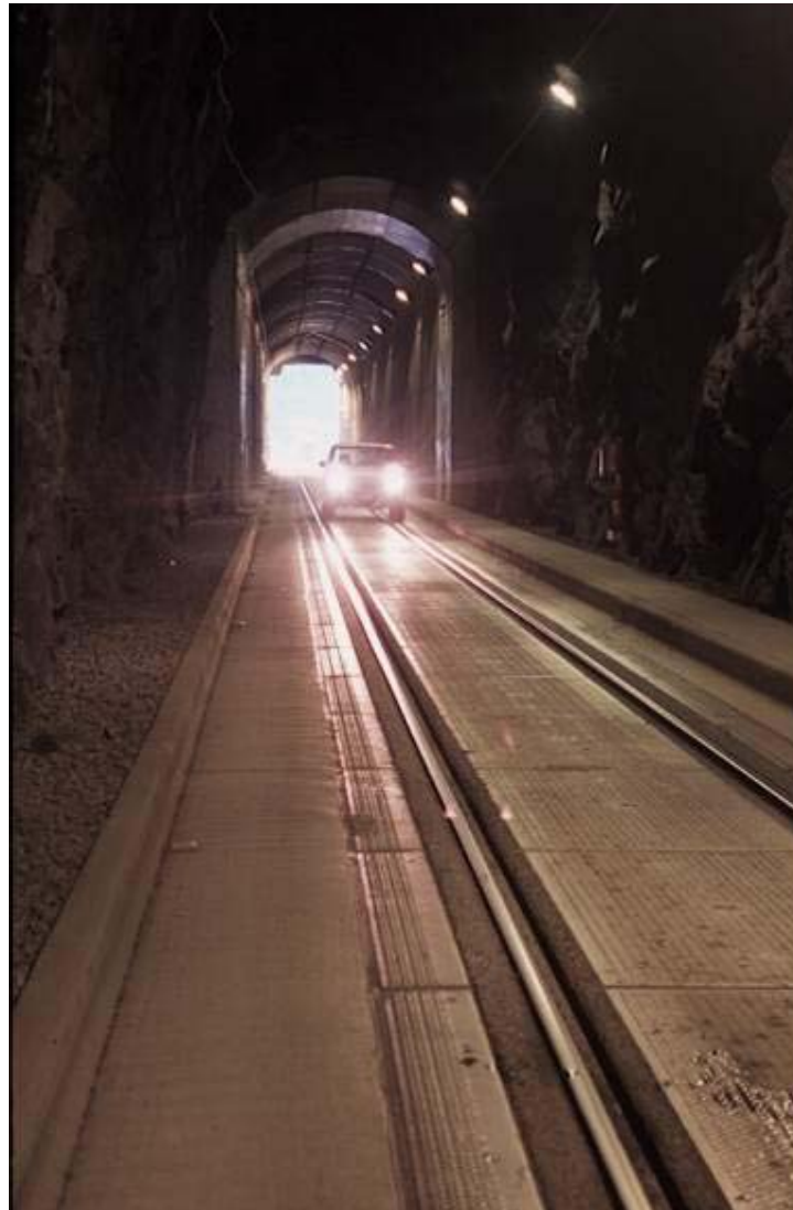
FIGURE 5 Composite roadway and rails in Whittier Tunnel.
