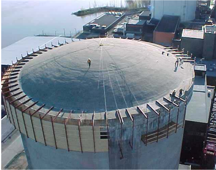
FIGURE 17 Repair of the Gentilly 1 nuclear containment structure.
