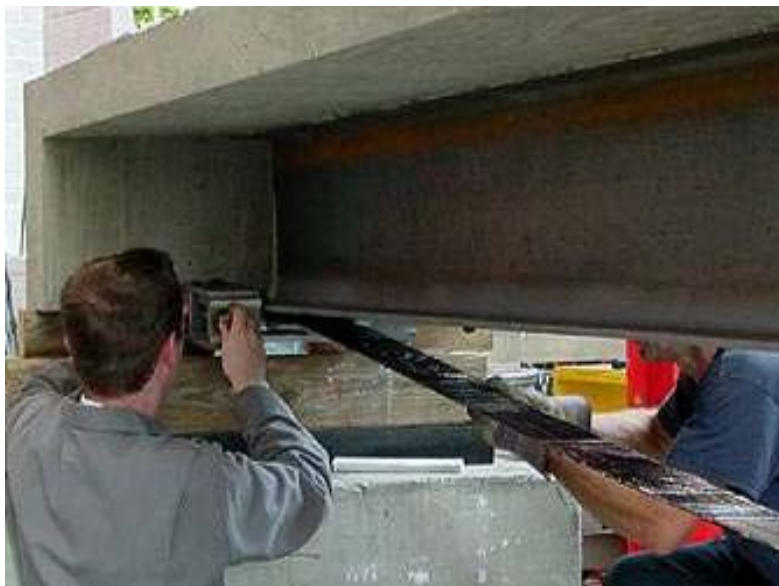
FIGURE 21 Prestressing of externally bonded CFRP strips for a steel-concrete composite beam.
