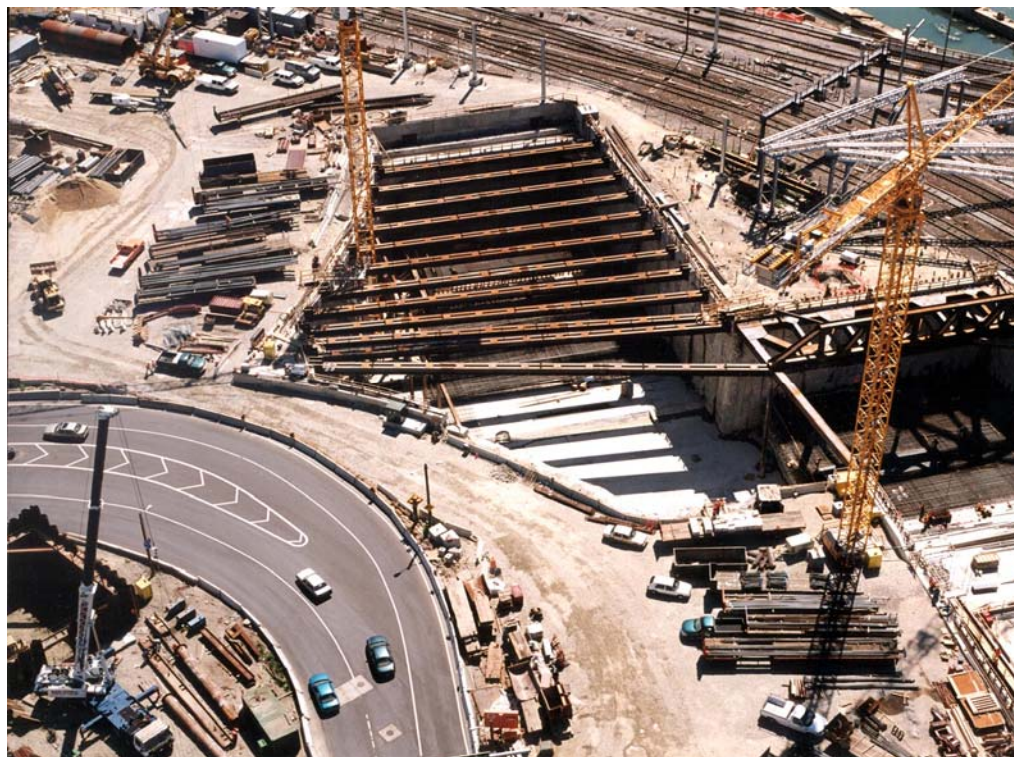
FIGURE 4 Central Artery Tunnel jacking pit.
