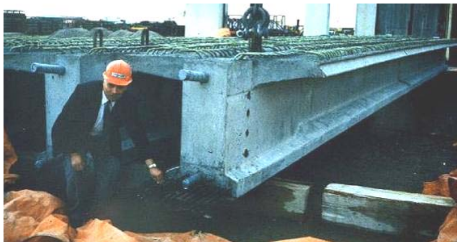
FIGURE 5 Centre Street–Beddington Trail Bridge bulb-tee girders.
