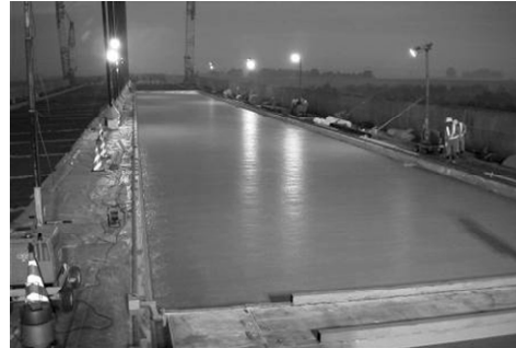
FIGURE 19 Mihara cable-stayed bridge, Hokkaido, Japan, with deck superstructure constructed from composite ECC-steel, opened 2004 for traffic. (Courtesy of V. C. Li, University of Michigan, 2005)
