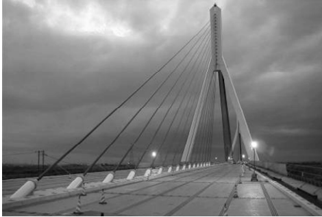
Cable Stayed Bridge Hokkaido, Japan Completed: Oct., 2004 Open to traffic: April, 2005 Length: 1000 m, span: 340 m Deck area: 20,000 sq. m.; ECC layer thickness: 38 mm
