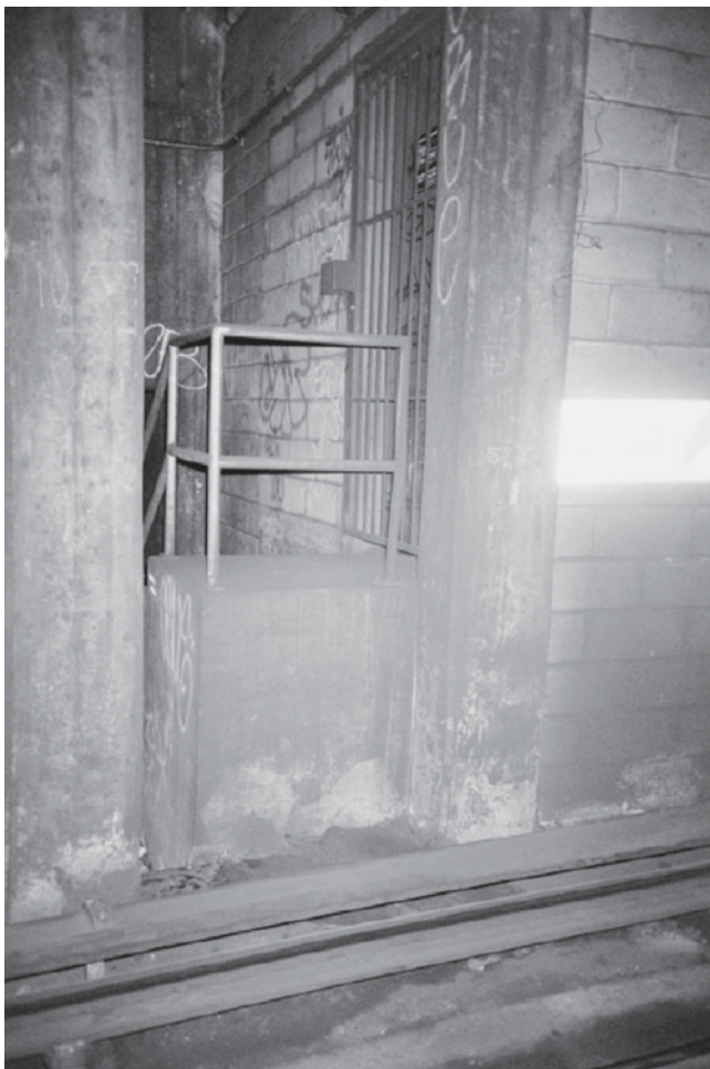
Figure 8 View of receiver location. Access to relay Room is through fenced doorway.
