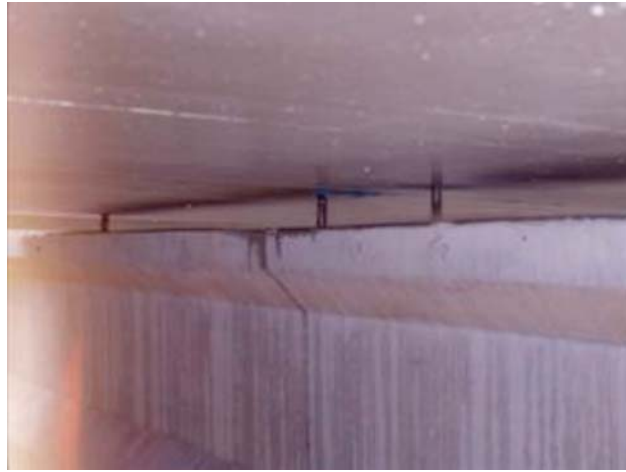
Figure 5.2.1.2-1 FRP deck and connection studs.
