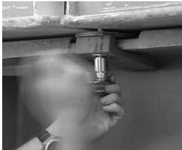
Figure 3.7.3.2.3-1 Anchor clips used on Jay Street Bridge.
