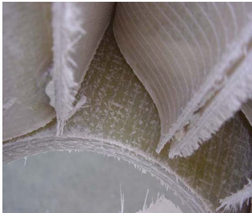
Figure 8-8 No adhesive between facesheet and core webs.
