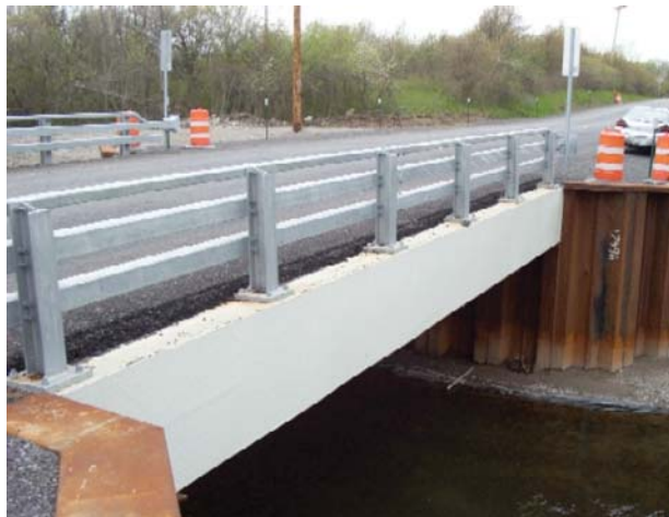
Figure 5.2.1.5-1 Typical steel railing connected to FRP deck.
