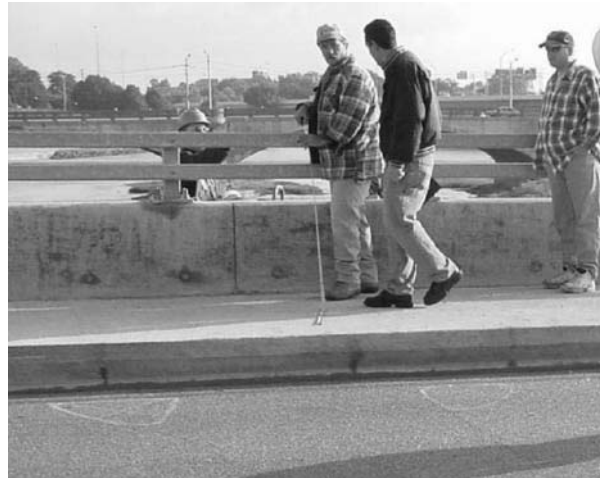
Figure 3.7.5.1-1 Finished cast-in-place curb, sidewalk, and parapet.
