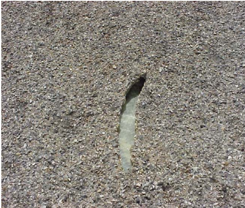
Figure 8-2 Wear surface lift on deck.
