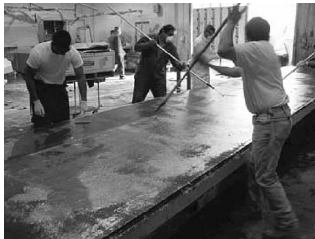
3.5.1-2 Hand lay-up operation: fabric saturation.
