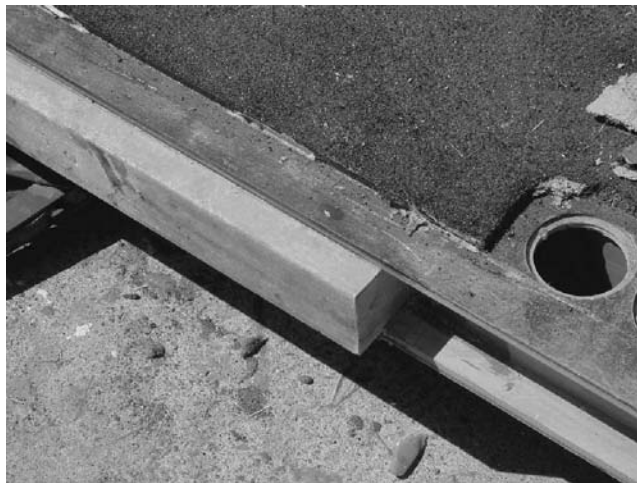
Figure 3.7.3.1.1-2 Shear key on Schuyler Heim decks.
