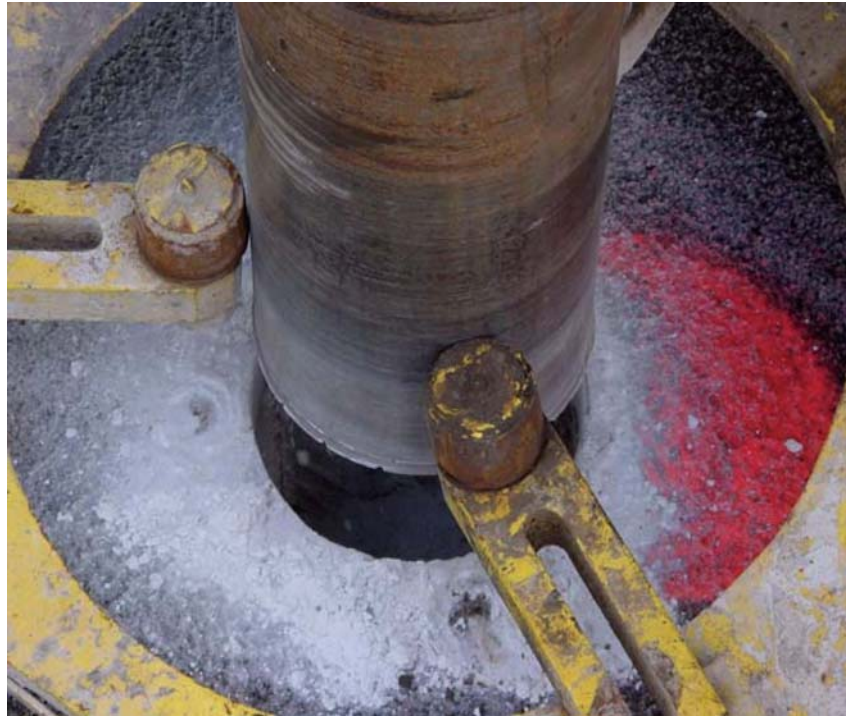
Figure 8-7 Coring through deck.
