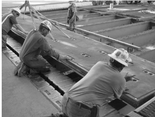
Figure 3.7.3.2.4-1 Carbon/fiberglass deck being installed in the Schuyler Heim lift bridge.
