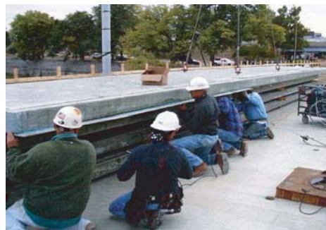
(c) Butt joint with shear splice plate strip
