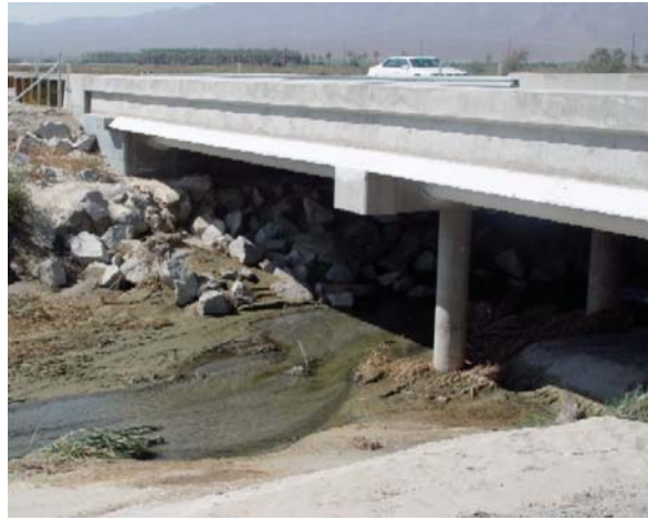
Figure 5.2.1.5-2 Typical concrete parapet.
