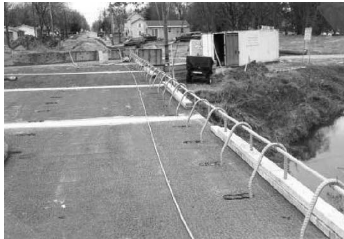
3.7.5.1-2 Reinforcing anchor details for the cast-in-place curb.
