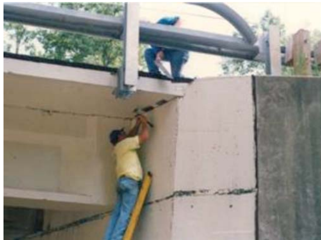
Figure 5.2.1.3-1 Shimming of gap between deck and abutment.
