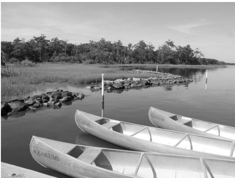
FIGURE 3-9 Stone sill examples from St. Mary's River, St. Mary's County, Maryland, and North Carolina Patches of existing marsh were incorporated into the plan. SOURCE: VIMS shoreline photo archive, and North Carolina Coastal Federation. Courtesy of VIMS and the North Carolina Coastal Federation.
