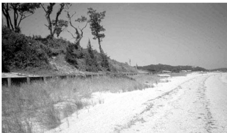
FIGURE 3-6 Landward placement of bulkheads leaving existing marsh and beach intact, at least for the near term.
