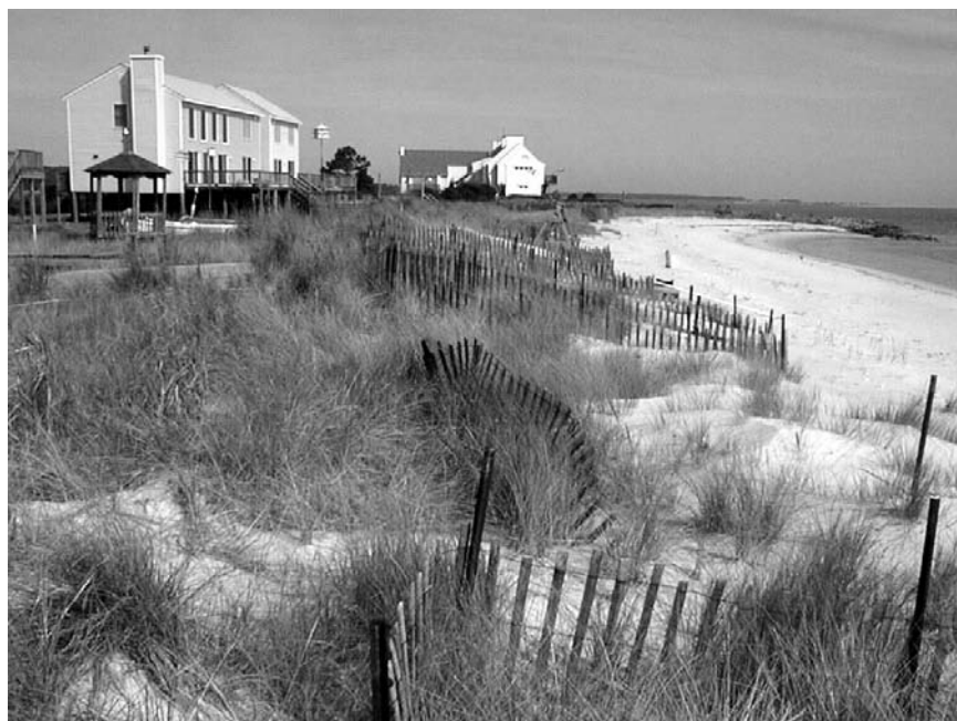
FIGURE 3-2 A dune beach along Virginia's Chesapeake Bay. Note the fencing and dune grass plantings. The fences and vegetation help to induce baffling and sand settlement. SOURCE: VIMS photo archive. Courtesy of VIMS.
