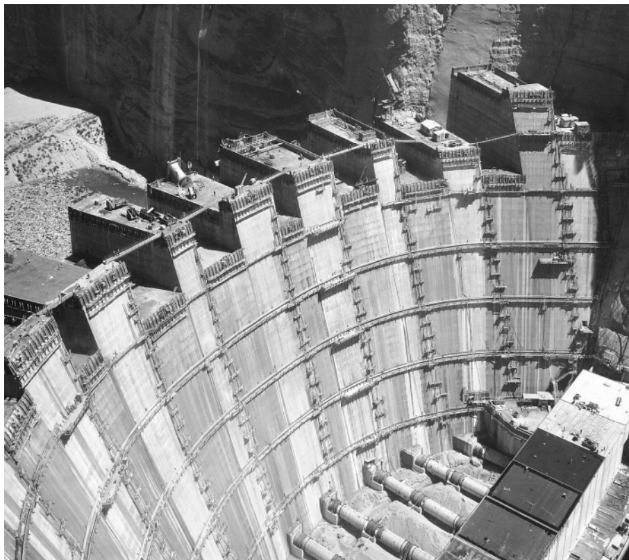
FIGURE 2-4 Glen Canyon Dam, nearing the end of its construction and prior to the beginning of water storage in 1963. SOURCE: U.S. Bureau of Reclamation.
