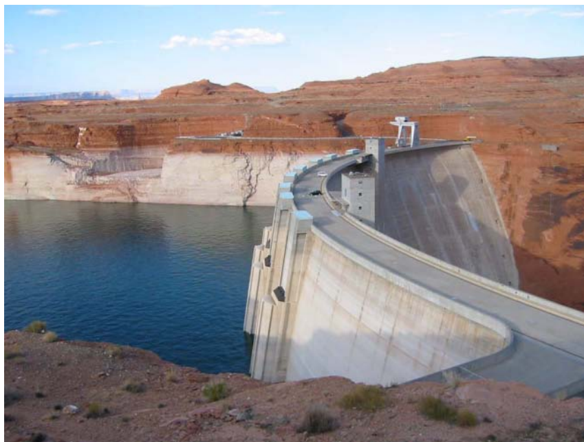
FIGURE 2-9 Glen Canyon Dam and Lake Powell, August 2004. Note the residual ring around the top of the lake caused by declining water levels. SOURCE: Courtesy of Brad Udall, University of Colorado.
