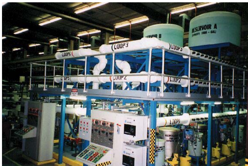
FIGURE 4-1 Research pipe loops at the EPA's Test and Evaluation Center that are used to examine contaminant transport behavior, decontamination strategies, and contaminant monitoring approaches.
