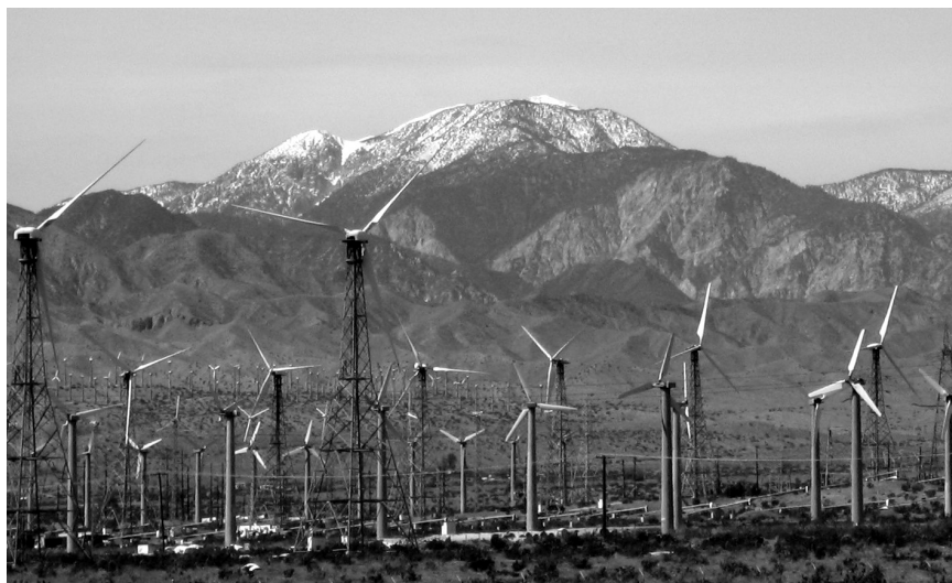
FIGURE 3-2a Turbines at San Gorgonio showing lattice and monopole towers. SOURCE: Photograph by David Policansky.
