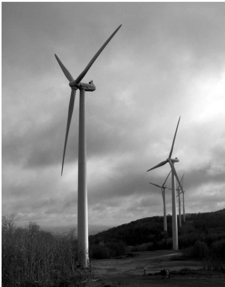
FIGURE 3-3 Mountaineer Wind Energy Center, West Virginia. The five turbines in this photograph are at the southwest end of the array of 1.5 MW turbines; they are at the lower left of the aerial view in Figure 3-7. SOURCE: Photograph by David Policansky.
