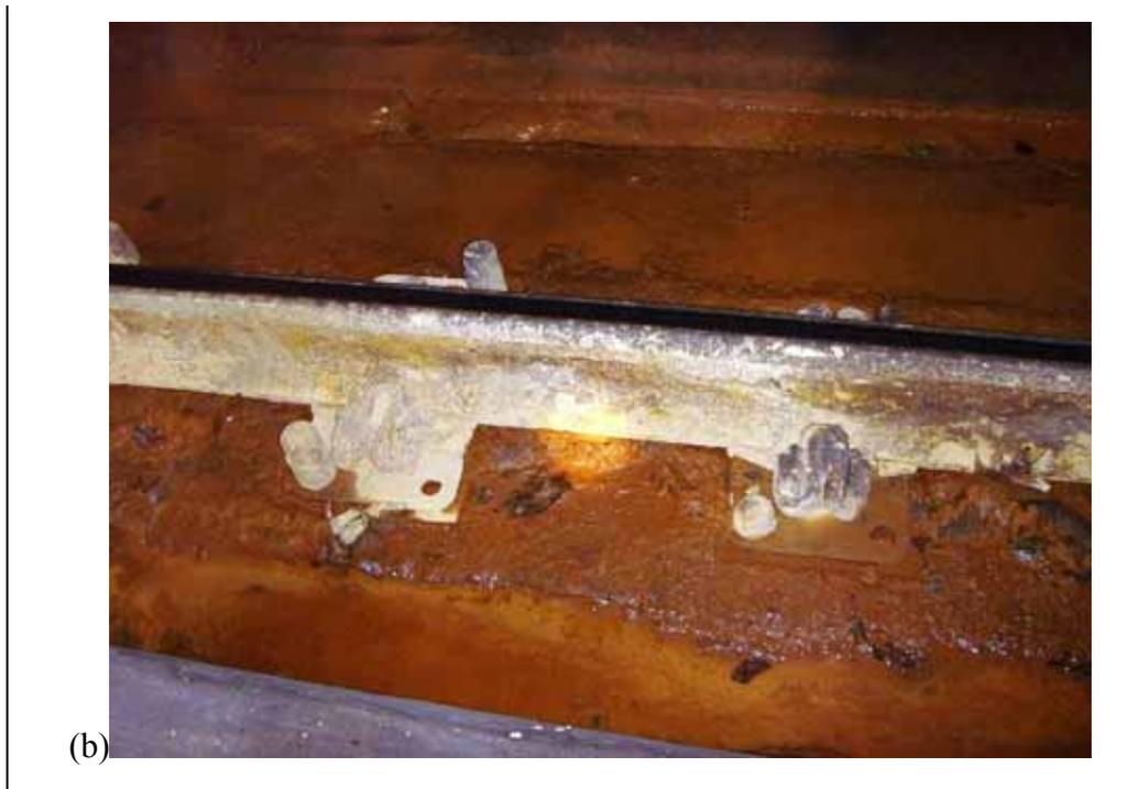
Figure 16. (b) Salts deposited along the tracks at Southeastern Pennsylvania Transportation Authority.
