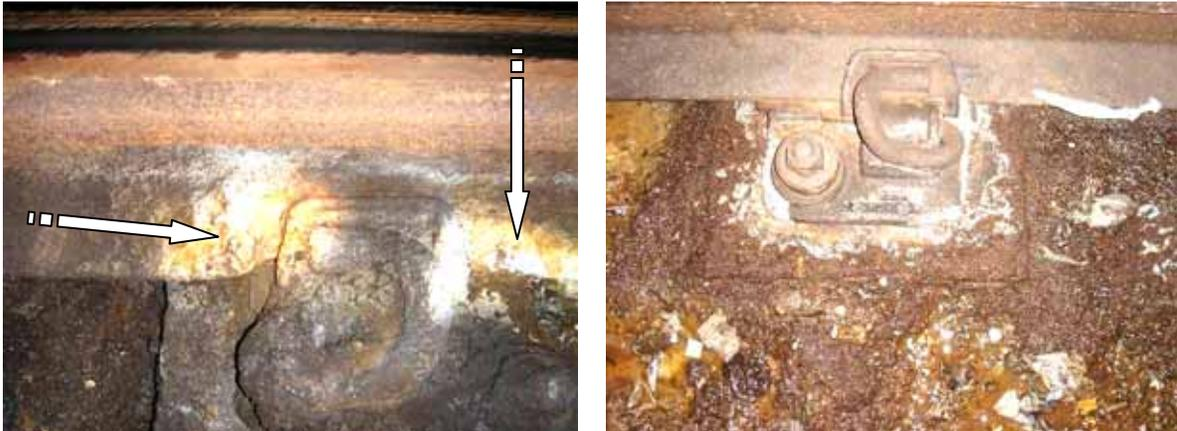
*TTC-Toronto tracks showing deposited salts and resulting corrosion.*
