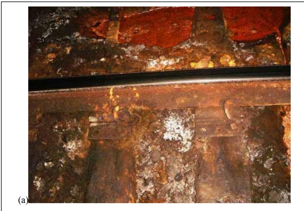
Figure 16. (a) Salts deposited along the tracks at Port Authority Trans-Hudson.
