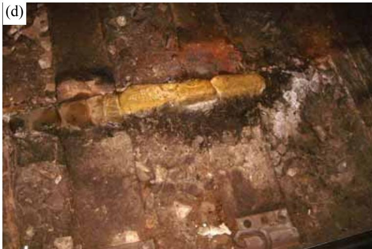
*PATH Transit System showing (a, b) rail corrosion, (c) ice spikes from sealant used to prevent water leaks in the tunnel, and (d) salts deposited along the tracks. Note: The site visit was conducted during January 2006 and due to the weather conditions in New York and New Jersey, the water leaks froze forming the ice spikes shown in photo (c).*
