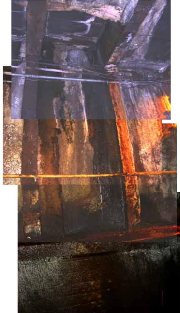
*MTA-NYCT tunnels showing severe water leakage from the walls, severe humidity under the tracks, and erosion of the rail base.*
