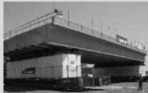
*Graves Avenue span over I-4, northeast of Orlando, Florida, was installed in minutes with self-propelled modular transporters.*
