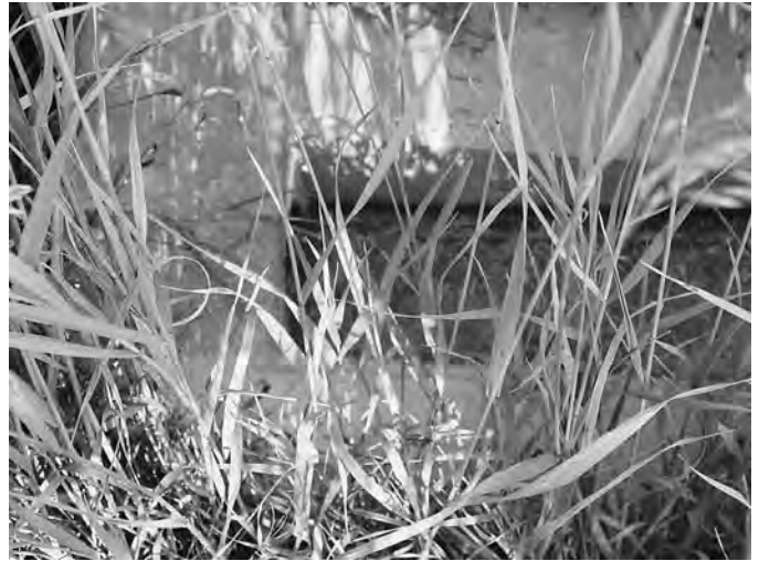
Figure 44. View from shoulder and close-up view of overgrown drainage outlet, Kansas SPS-2.
