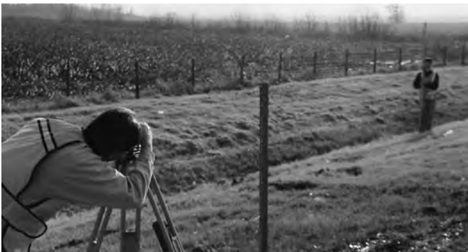
Figure 56. Rod and level measurement of elevation of bottom of drainage outlet pipe at headwall.
