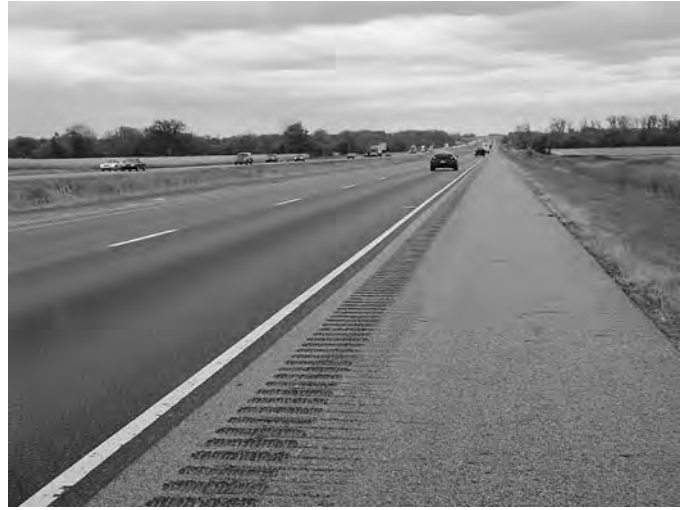
Figure 31. Michigan SPS-1 site.
