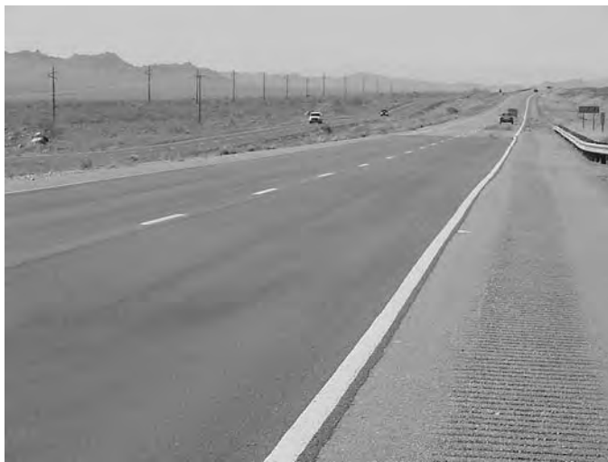
Figure 14. Arizona SPS-1 site.
