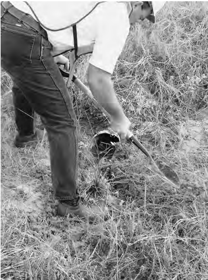
Figure 47. Clearing drainage outlet, Texas SPS-1.
