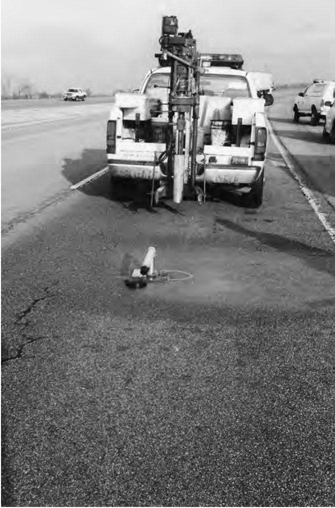
Figure 53. Coring by state DOT personnel, Arkansas SPS-1.
