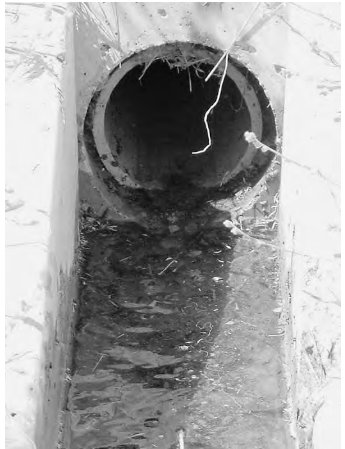
Figure 63. Free flow is established when clear water flows out of drain.
