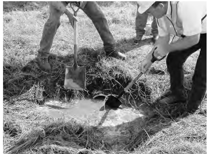
Figure 48. Clearing drainage outlet, Texas SPS-1.
