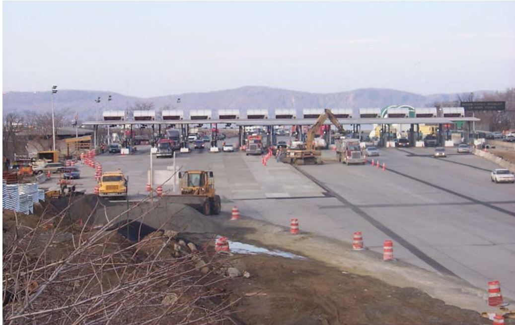
FIGURE 6 Progression of work on Tappan Zee Toll Plaza.
