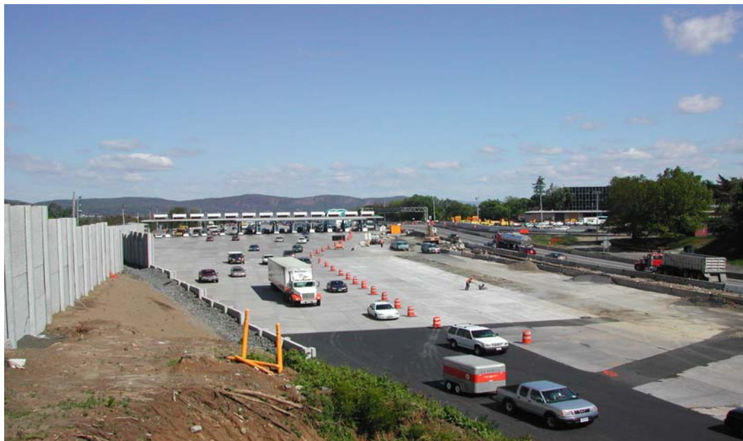
FIGURE 7 Construction nearing completion on Tappan Zee Toll Plaza.
