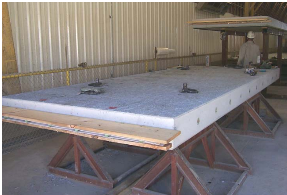
FIGURE 4 Precast concrete panel for Tappan Zee Toll Plaza reconstruction.
