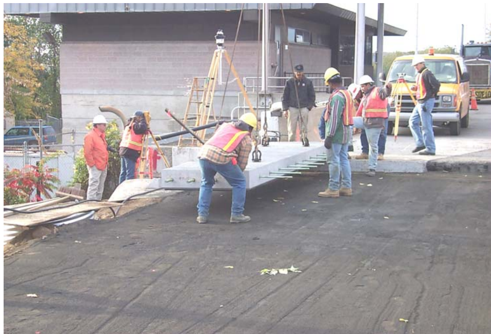
FIGURE 5 Placement of precast panel at Tappan Zee Toll Plaza.
