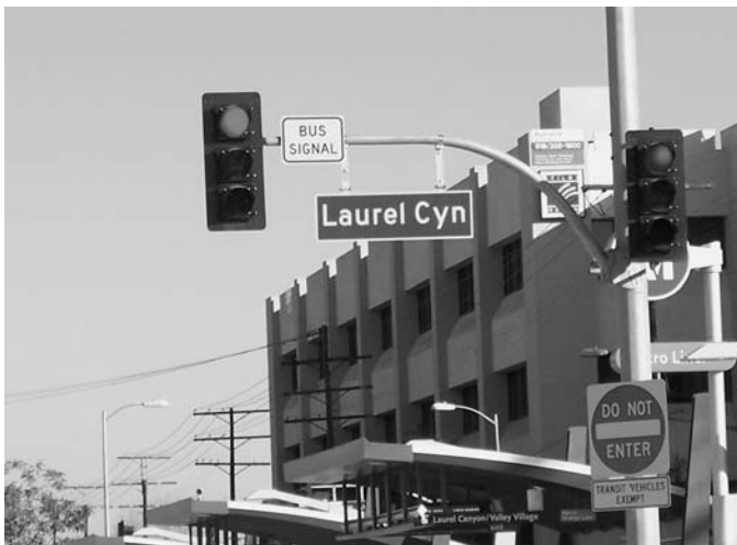
Figure 5-5. Bus signal sign mounted next to bus signal at intersection of Orange Line busway, Los Angeles.
