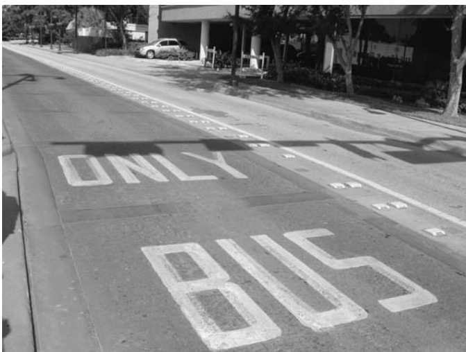
Figure 5-7. “BUS ONLY” pavement markings at LYMMO intersection, Orlando, Florida.
