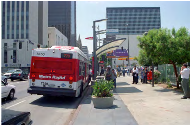
SOURCE: Kittelson & Associates, Inc. EXHIBIT 4-7 Curb Bus Lane (Los Angeles)
