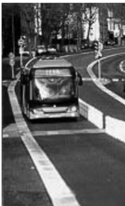
Exhibit 5-3. Exclusive lane for BRT in Rouen, France.
