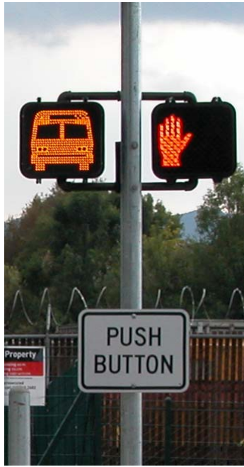
Figure D-4: Pedestrian Signal Bus LED Indication
