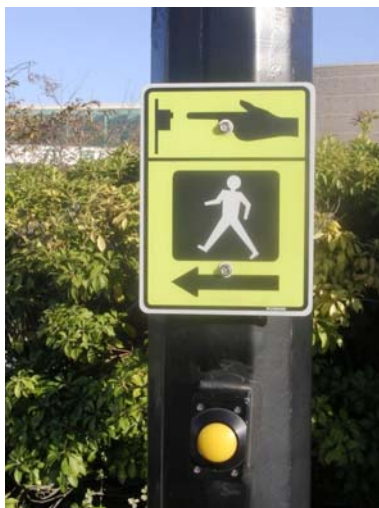
Figure G-7: Pedestrian Push Button and Sign
