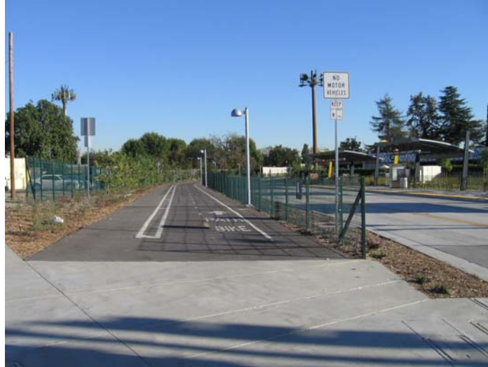
Figure D-3: Bicycle/Pedestrian Path along the Metro Orange Line
